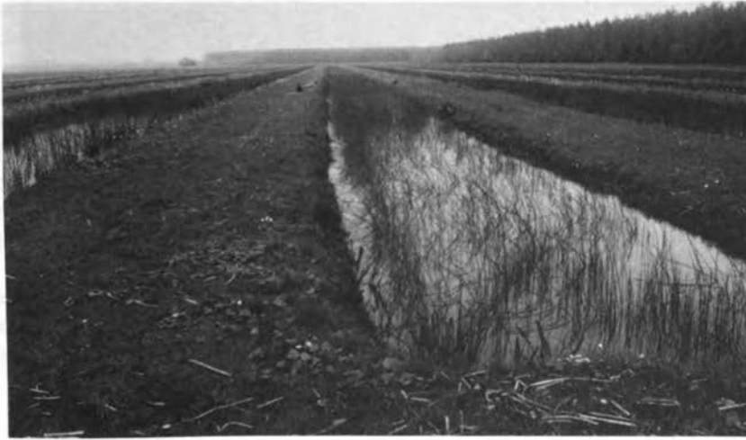
Wastewater is purified as it percolates through beds of the bulrush Scirpus lacustris near Elburg, the Netherlands. (C. D. McNabb)
