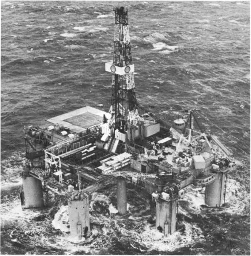
Oil drilling platform in North Sea buffeted by heavy seas. (Courtesy, Asiatic Petroleum Corporation)
