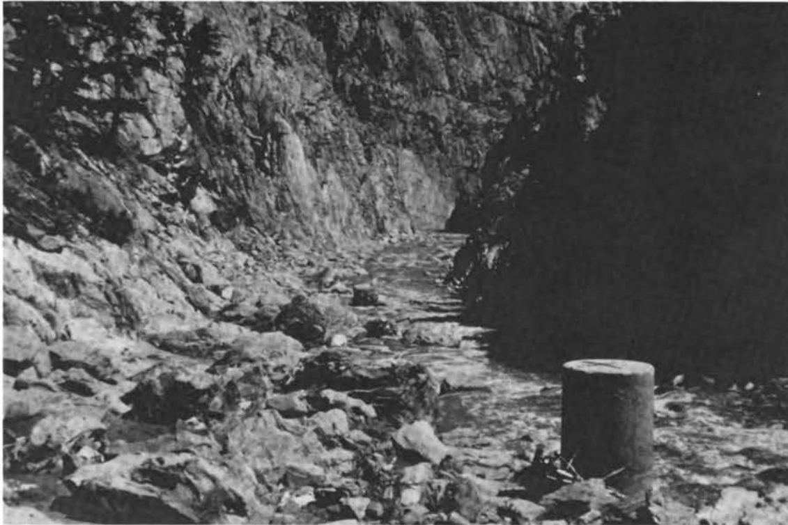
FIGURE 33 Scour in the Narrows Area near the Bureau of Reclamation Diversion Structure
