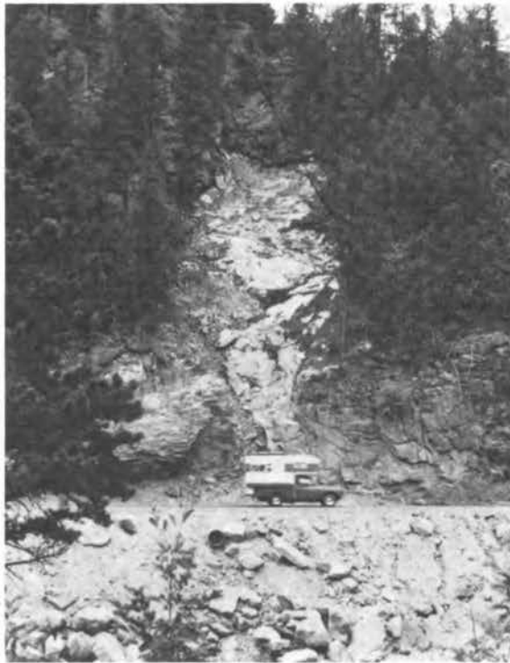
FIGURE 57 Landslide in Residual Soil
