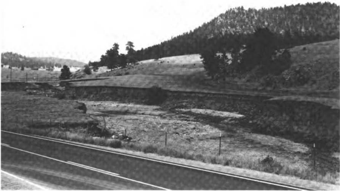
FIGURE 62 Erosion along Dry Gulch
