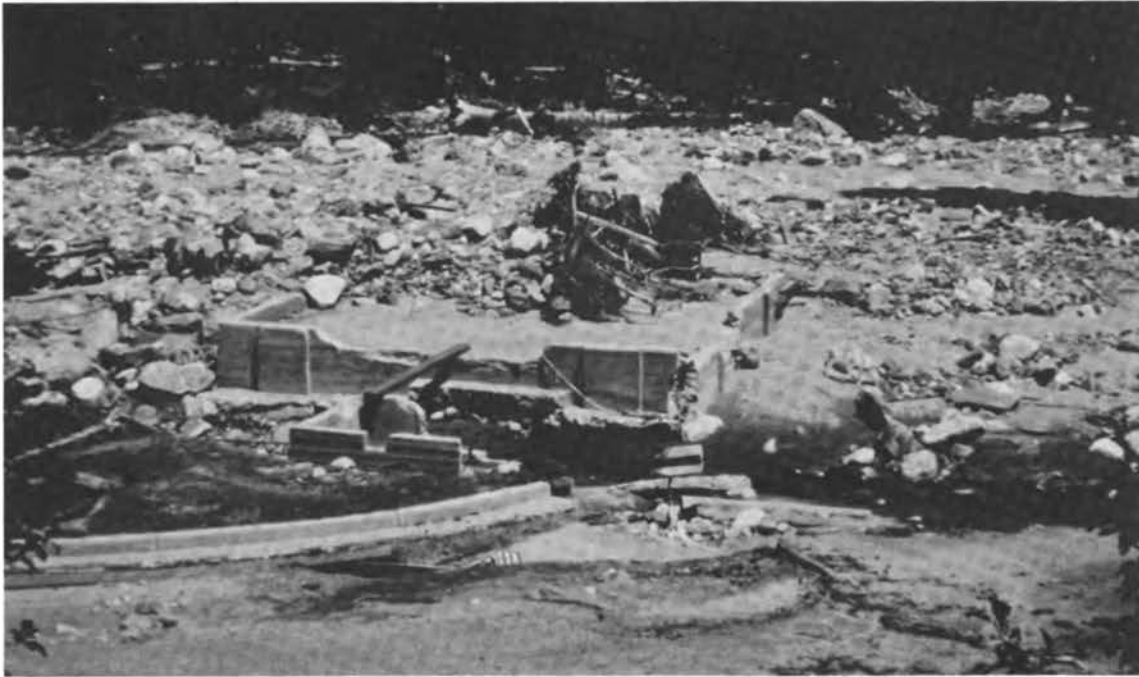
FIGURE 48 Loveland Power Plant
