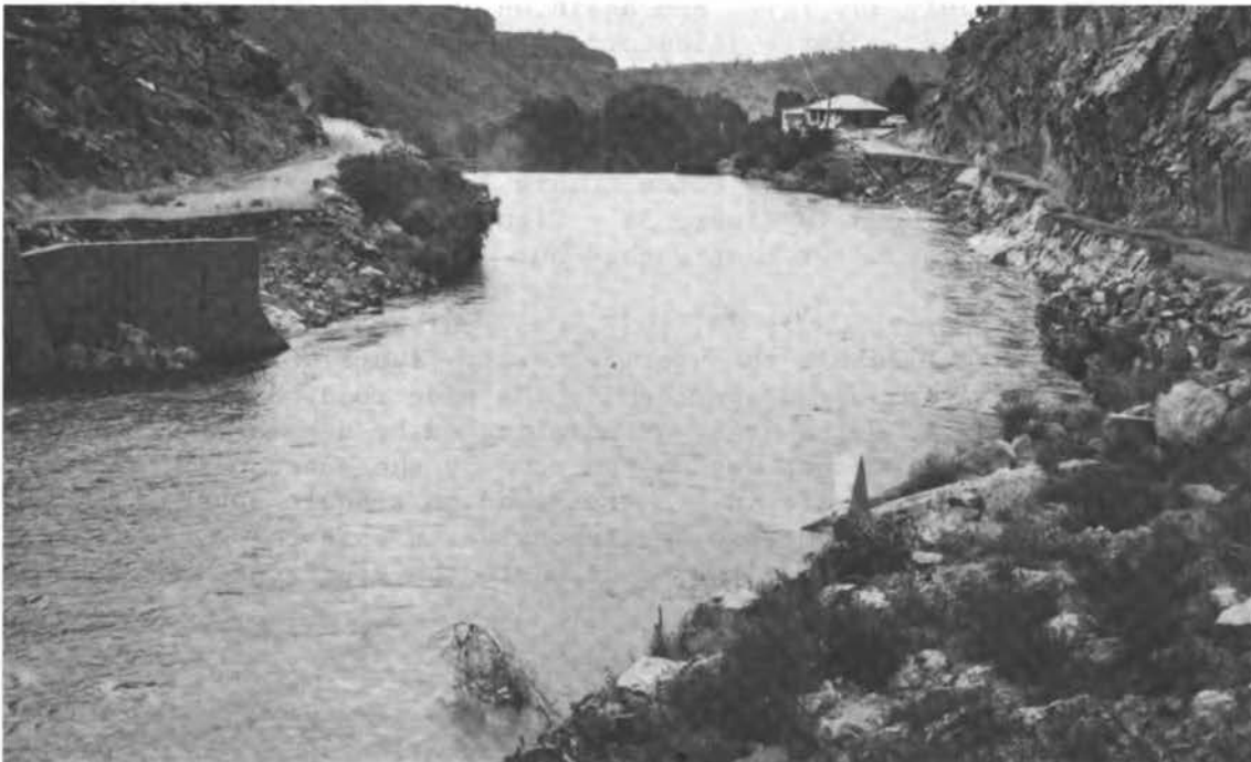
FIGURE 41 Abutments of Destroyed Bridge near Loveland Filtration Plant
