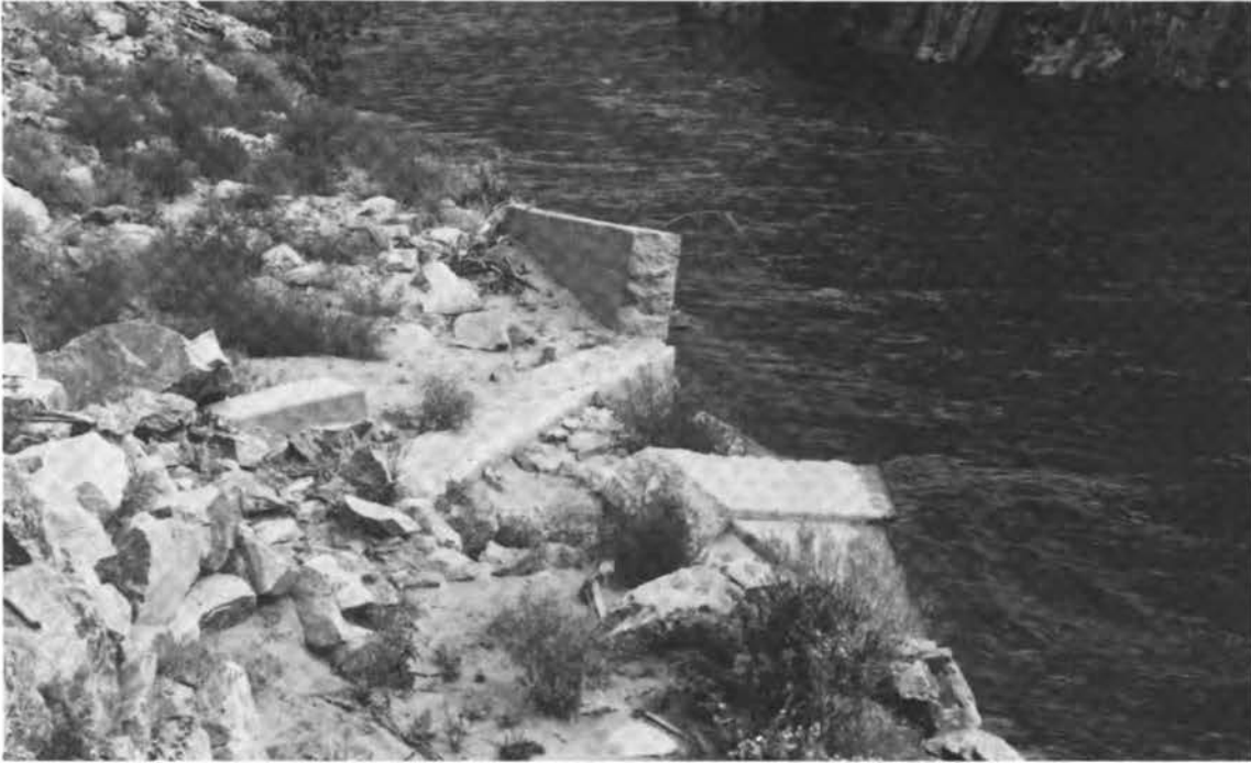
FIGURE 42 Close-up View of Right Abutment Shown in FIGURE 41
