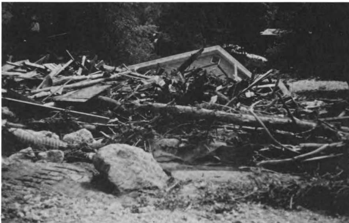
FIGURE 67 House near Drake Flattened by Boulders and Debris
