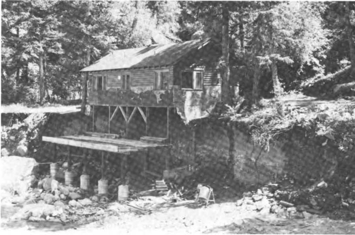
FIGURE 53 Remedial Measures Being Taken for Foundation Repair
