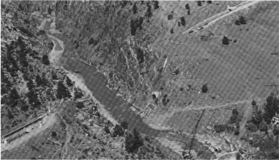
FIGURE 70 Siphon Support Structure and Feeder Canal Located at the Mouth of the Canyon
