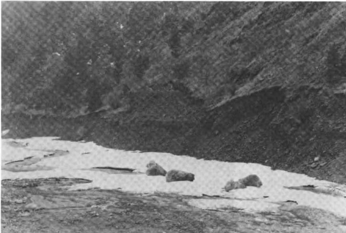
FIGURE 61 Slope Failure Formed about One Week after the Flood
