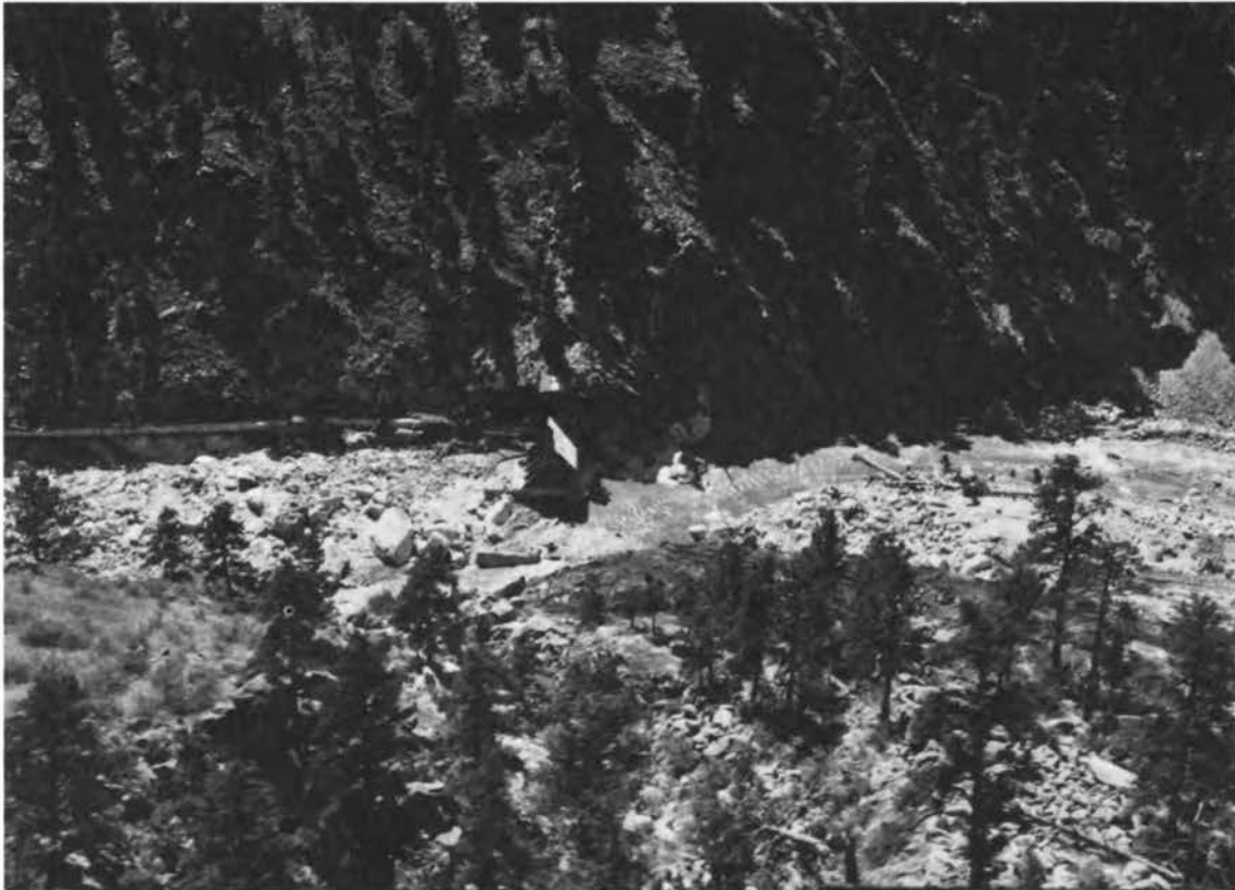
FIGURE 64 Remains of Loveland Hydroelectric Dam
