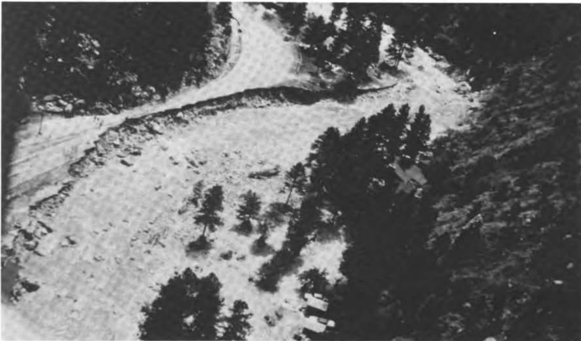
FIGURE 36 Erosion of Outside Bend on U.S. Highway 34
