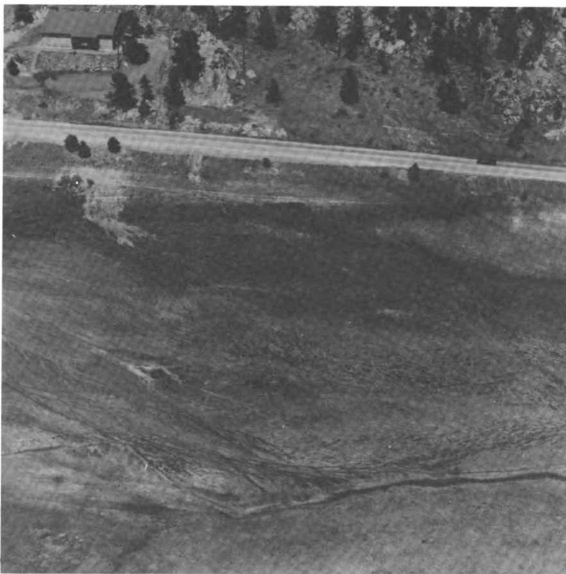
FIGURE 15 Sheet Erosion along Dry Gulch near Estes Park
