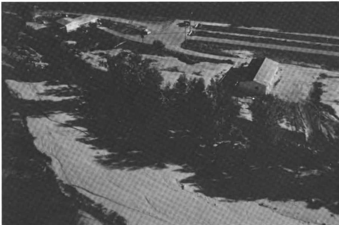
FIGURE 28 Deposits along the North Fork near the Fish Hatchery just Upstream from Drake
