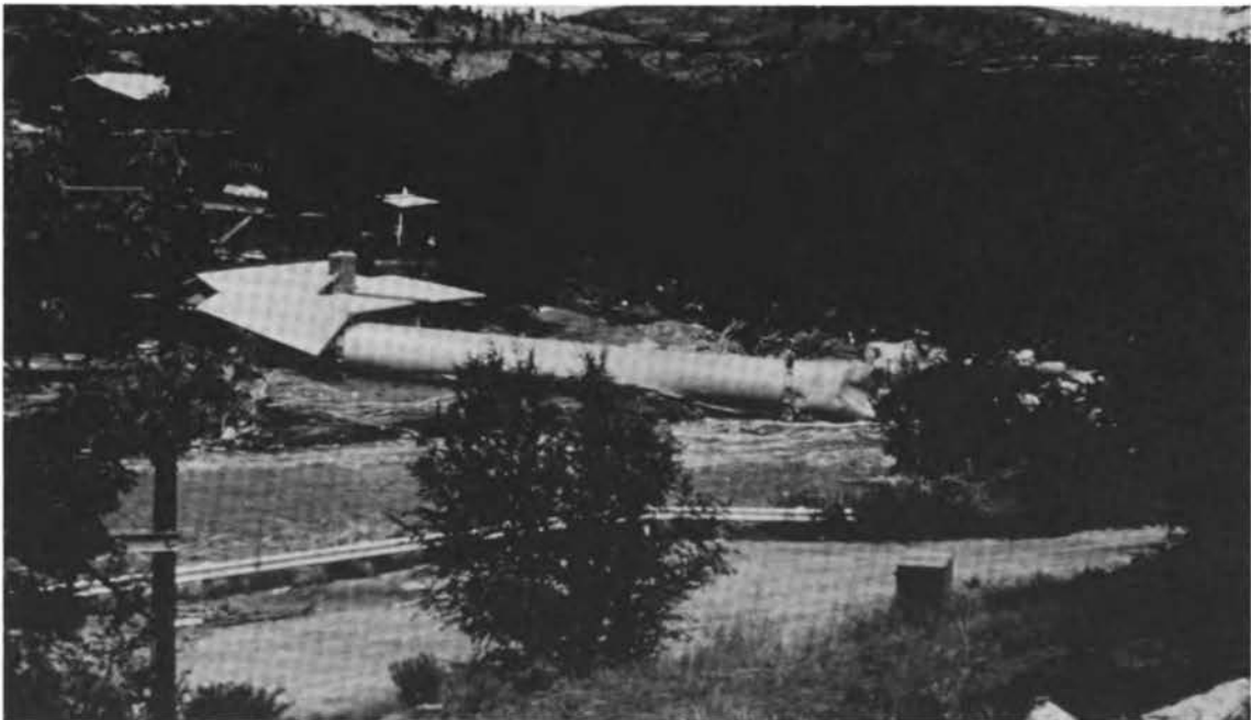
FIGURE 71 Remains of the U.S. Bureau of Reclamation Siphon
