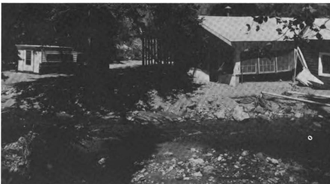
FIGURE 68 Sediment Deposited around House along West Creek
