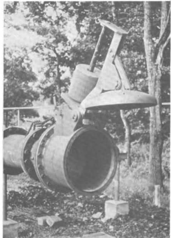
Fig. 57 : Relief device at end of pipeline Adequate mechanical strength
