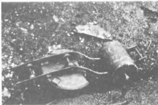
Fig. 56 : Relief device at end of pipeline after explosion. Insufficient mechanical strength
