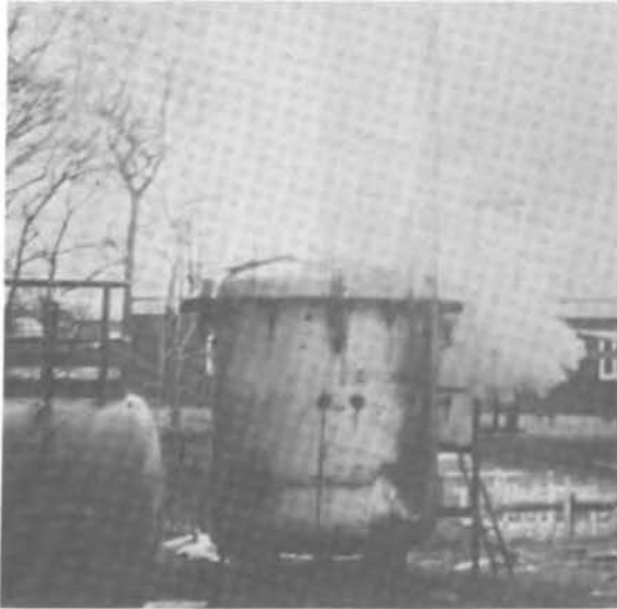
Fig. 37 : 10 m 3 vessel with pressure relief. Pigment dust explosion
