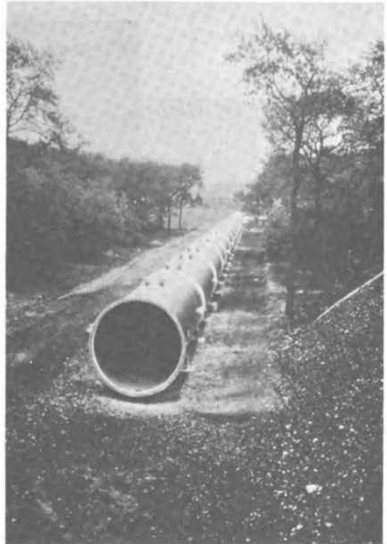
Fig. 24: Pipeline for basic research \varnothing 2500 mm length 140 m
