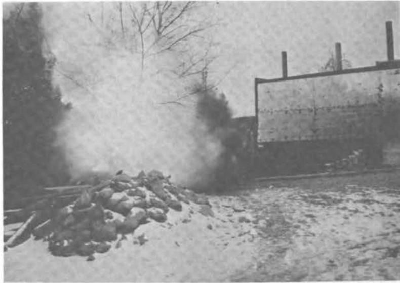
Fig. 40 : 60 m 3 bunker with pressure relief. Coal dust explosion
