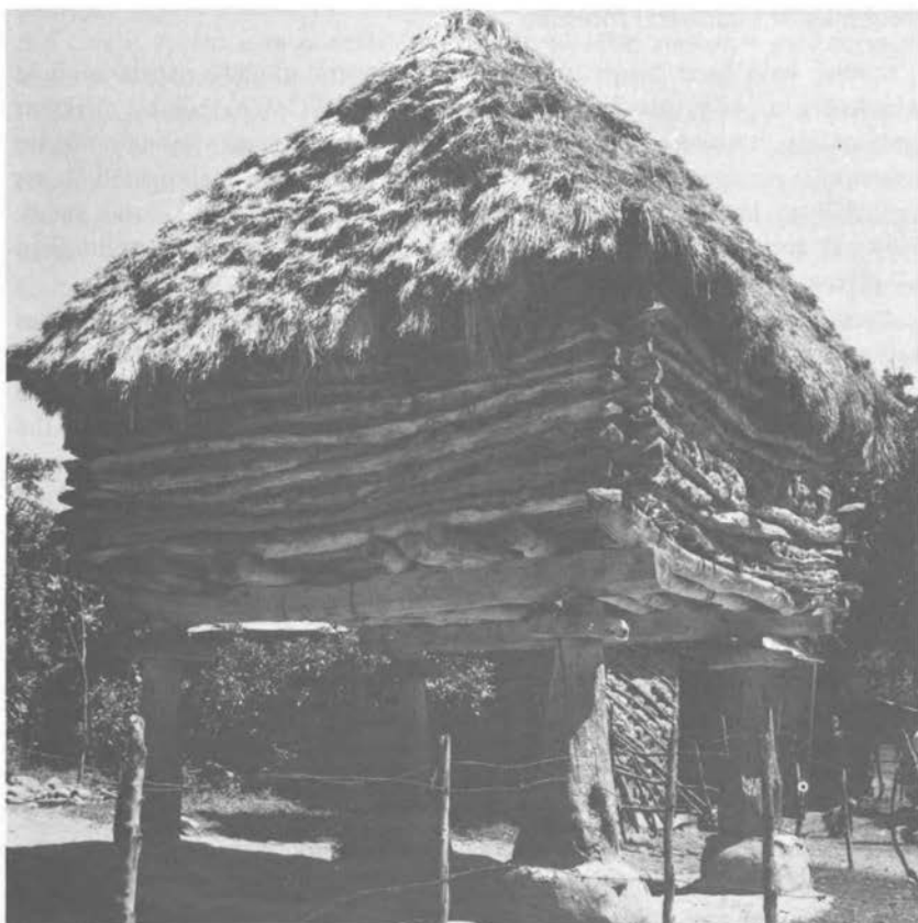
"Kanduch" lath and clay rice store, Chasemabad District, Gilan Province, Iran. Note the log-disc rodent baffles. (FAO photo)
