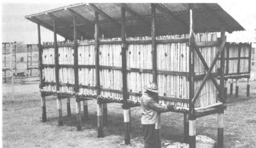
Large conventional crib constructed mainly from local materials (Courtesy W. Boshoff)
