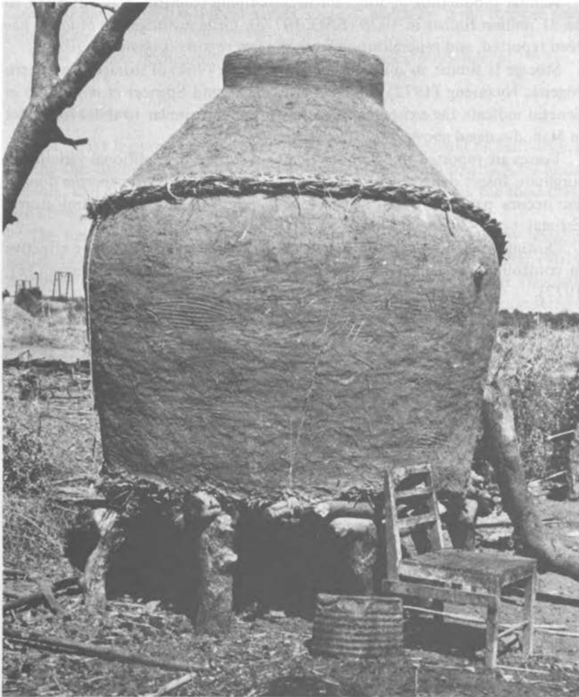
Traditional mud and straw grain store, N'Djamena, Chad (FAO photo by J. C. Abbott)
