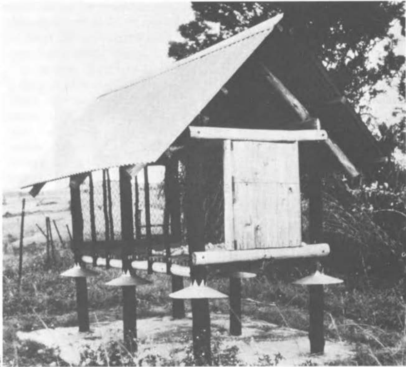
TPI commended mesh-sided crib, Swaziland. Note the corrugated iron roof and metal rat guards. (Crown copyright, Courtesy TPI)
