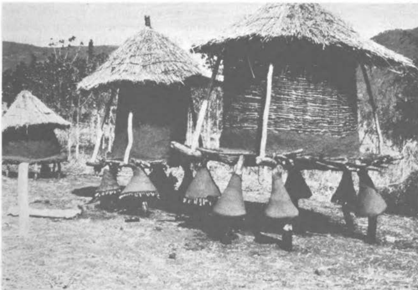
Muddied (left) and unmuddied (right) traditional nkhokwe, Malawi. Note the mud rat guards on wood framework. (Crown copyright, Courtesy TPI)
