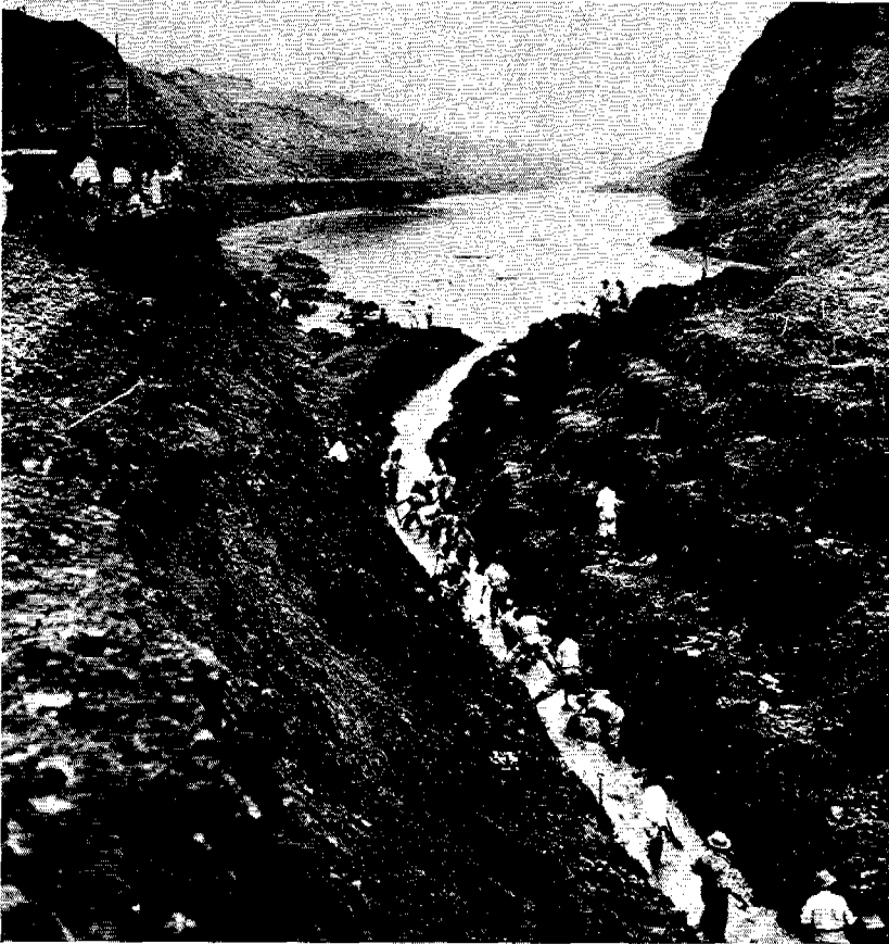
Laborers excavating a ditch through the toe of Cucaracha slide, Panama Canal (Photograph courtesy the National Archives).
