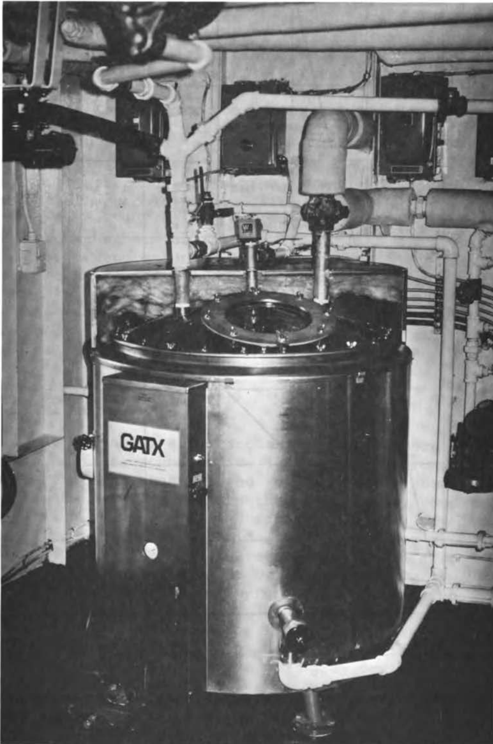
FIGURE 6 The ETS evaporator as installed on a U.S. Coast Guard vessel.
