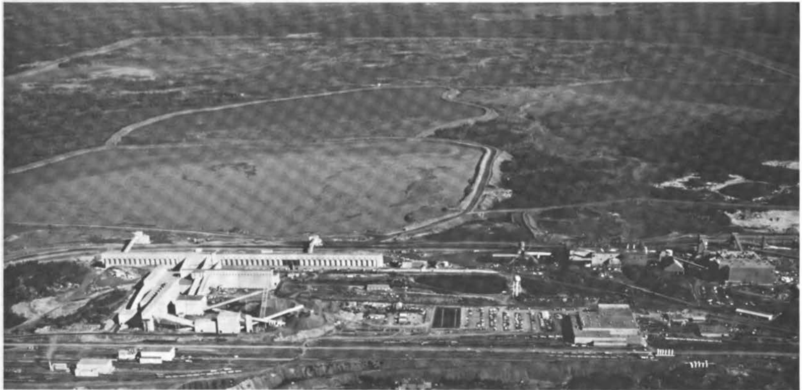
FIGURE 3.1 View of the Minntac taconite mines processing and waste disposal facility, Mountain Iron Minnesota, on the Mesabi Iron Ore Range. Wastes from ore processing are disposed of in the tailings basin (left center and background), which occupies an area of 16 square miles. The present disposal site is immediately behind the ore crushers and the concentrating plant in the left foreground. The narrow area extending across the top of the photograph is reserved for future tailings disposal.
