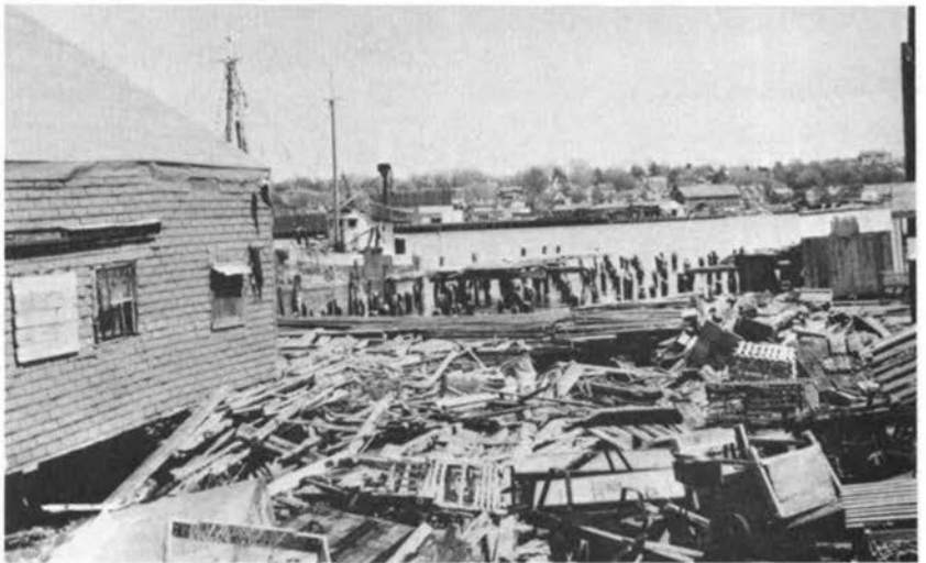
Dilapidated waterfront pier and shed with lobster pots, Gloucester, Massachusetts, 1962.
