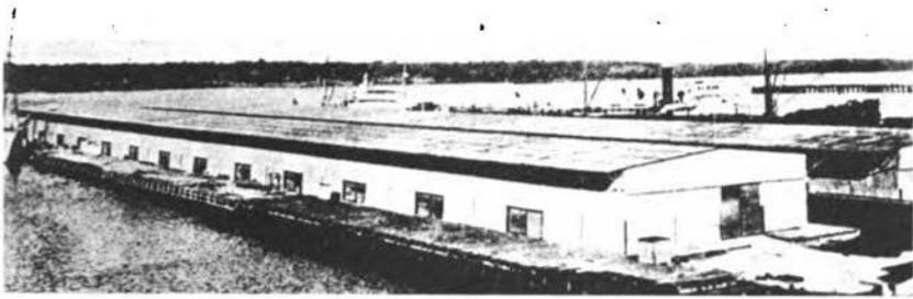
FIGURE 2 View of municipal piers and warehouses, Main Pier No.2.
