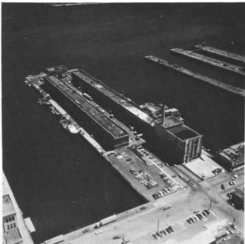
FIGURE 5 Boston Fish Pier.
