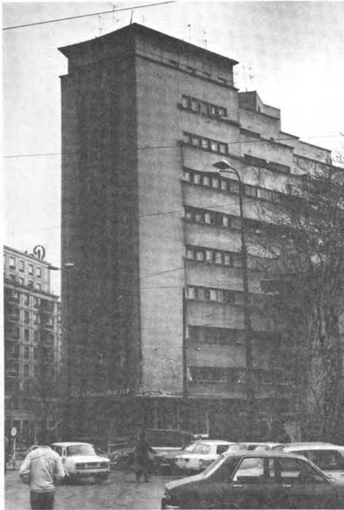
Figure 17 Apartment building with soft ground story designed and constructed prior to the 1940 Romanian earthquake.
