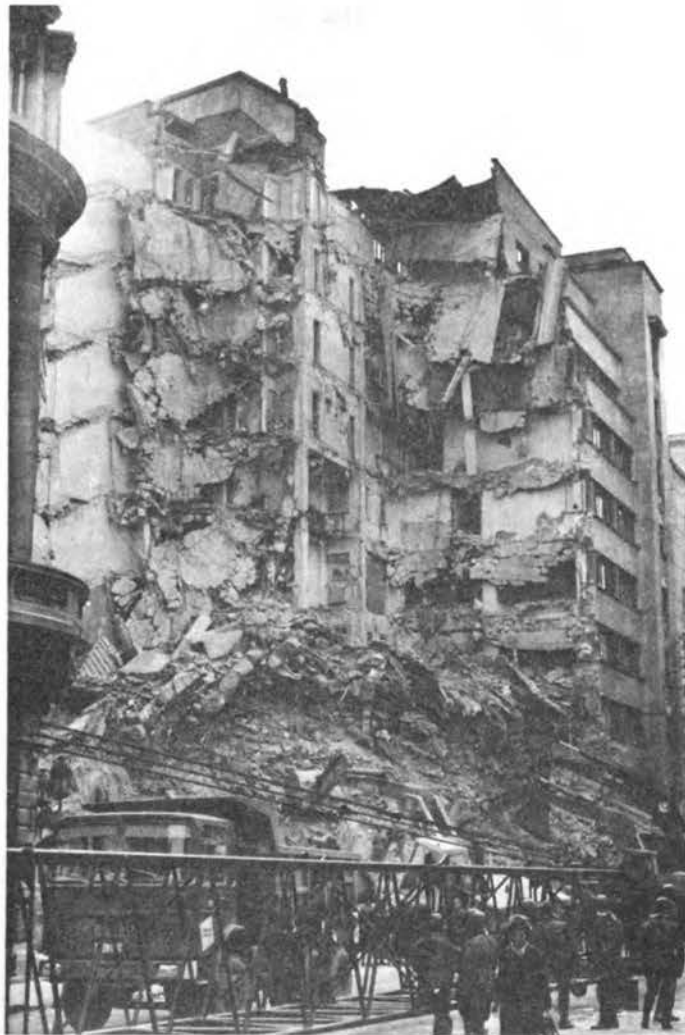
Figure 16 Collapsed building constructed prior to the 1940 Romanian earthquake.
