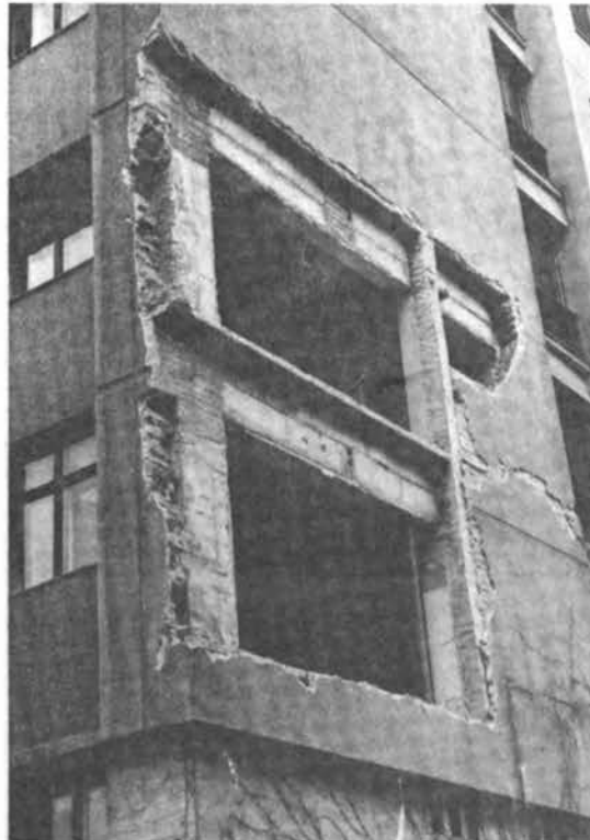
Figure 22 End wall of Emergency Hospital.
