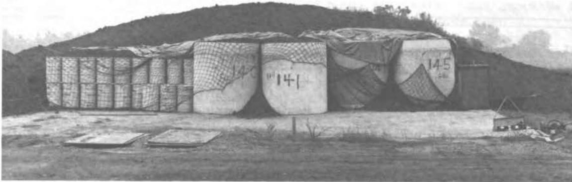
FIGURE 5 Storage pad and container for TRU alpha waste.
