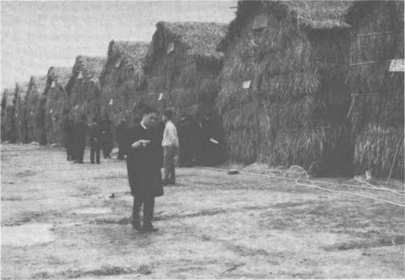
FIGURE 2.3 Completed mushroom houses covered with rice straw. ( Asian Business )
