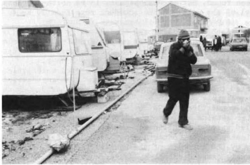
Figure 33. Aboveground water line with hookup for trailer in the town of Lioni.
