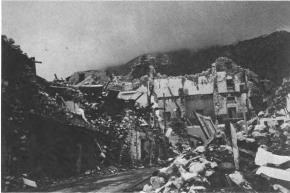
Figure 25 (cont'd). Damage in Laviano. (c) A view from the top of the town, showing the city hall in the background.
