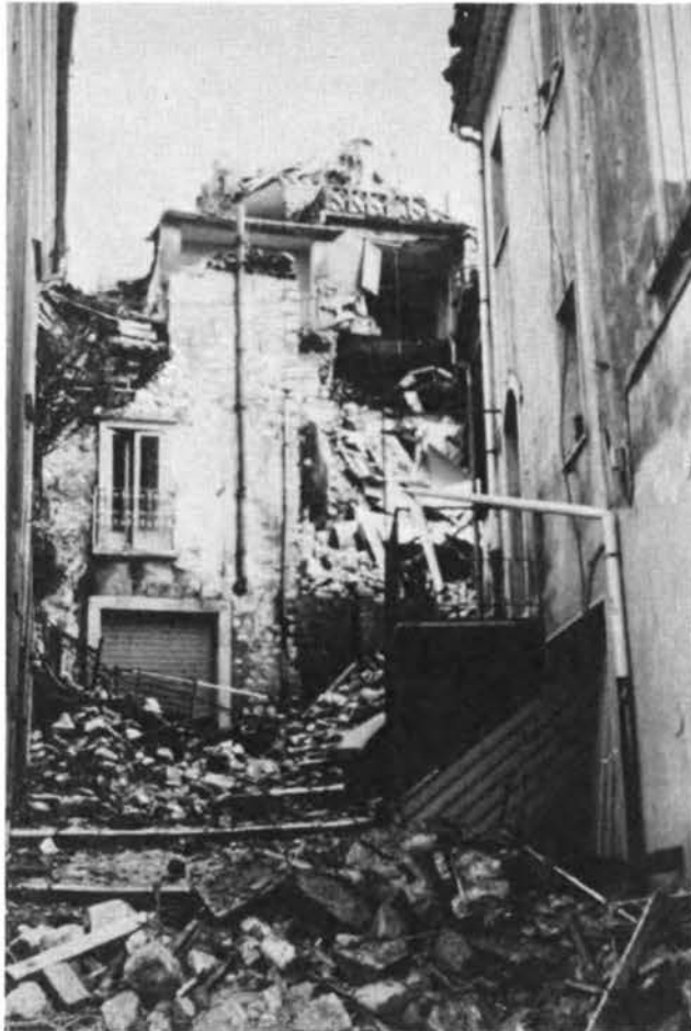
Figure 37. Narrow streets blocked with debris.
