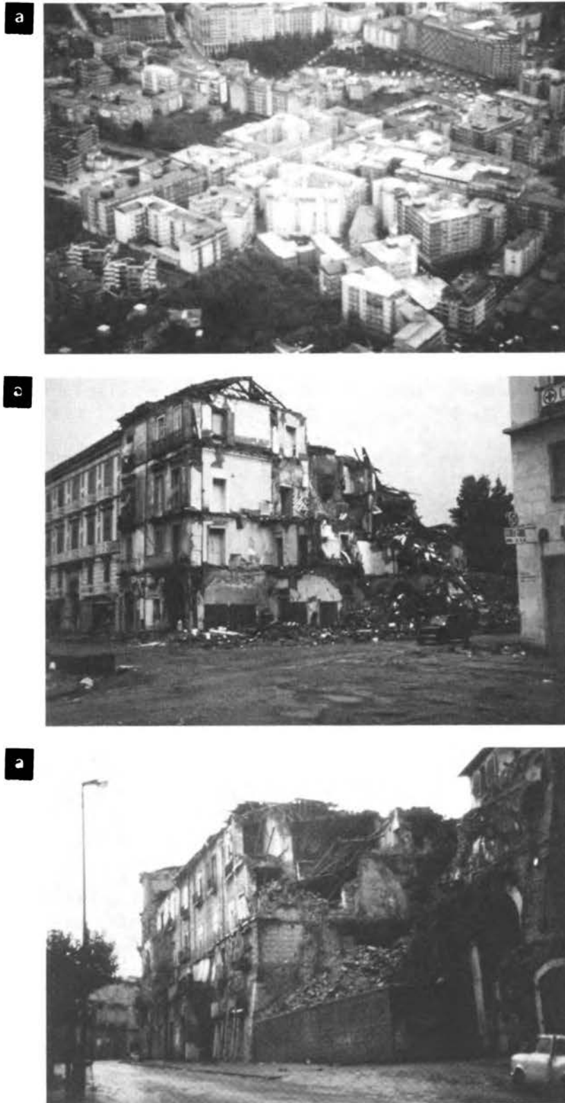
Figure 18. Damage at Avellino. (a) Aerial view. (b) Older construction collapsed. (c) The nearly total collapse of the old construction shows a large inward movement of the front wall at the second floor.
