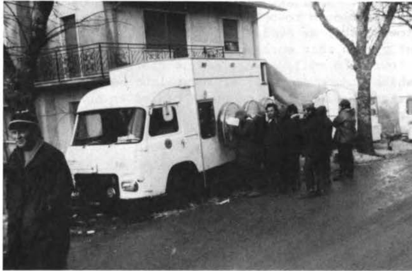
Figure 35. Mobile telephone substation being operated in the town of Teora. Telephones are on the sides of the vehicle.
