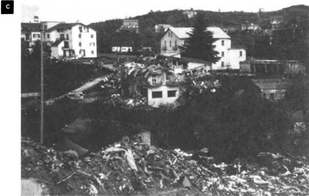
Figure 20 (cont'd). Damage to housing and police headquarters. (c) Failure of the local police headquarters. Need for these facilities to remain operational is obvious.
