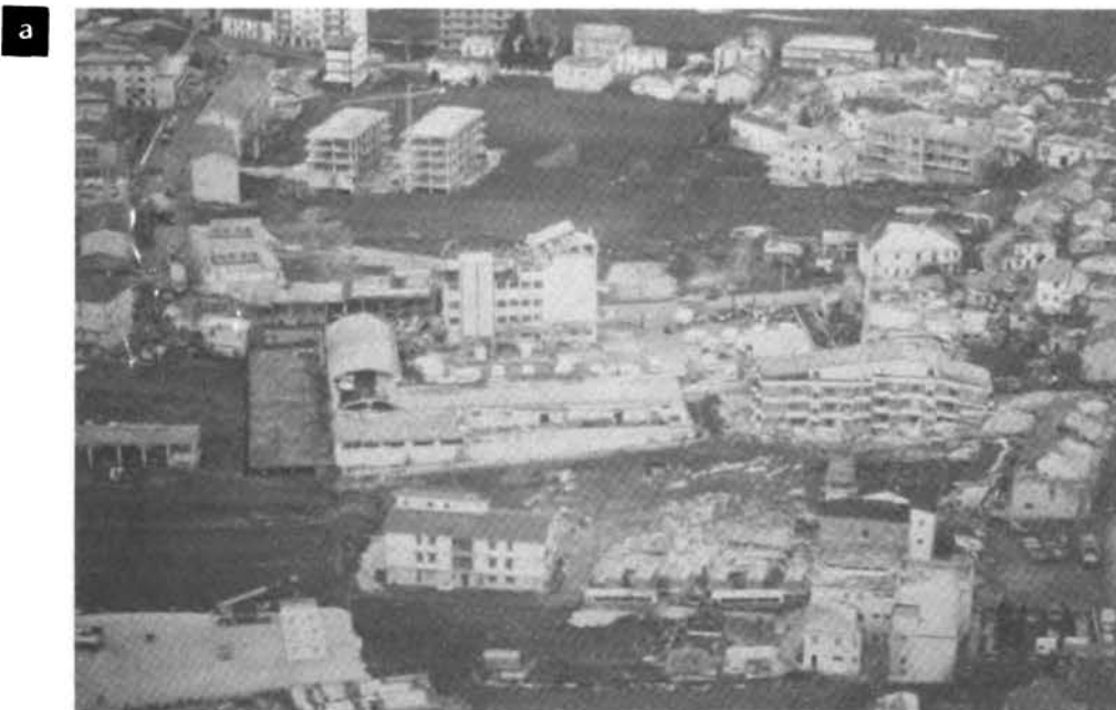
Figure 21. Damage to the Pallante factory. (a) This aerial view shows severe damage. The two housing units in the upper left were discussed earlier; to the right is the damaged housing unit shown in Figure 12.
