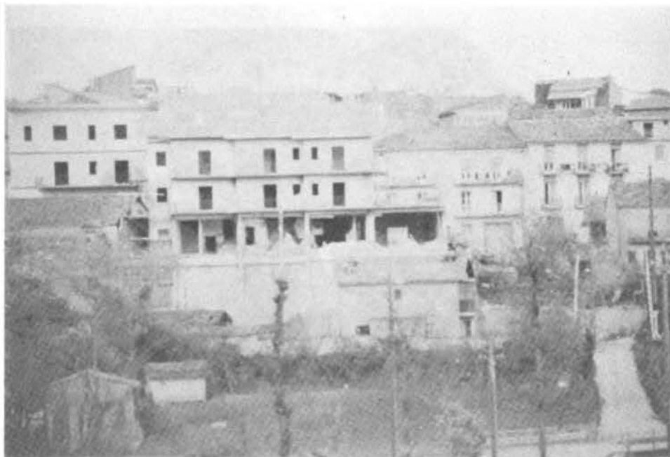
Figure 12. Damage to multistoried residential units. Both of these were so badly damaged that they could easily have collapsed with slight additional shaking.
