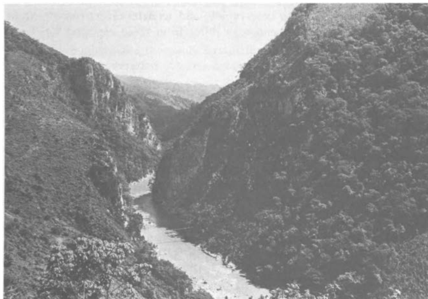
FIGURE 8-1 A narrow valley forms an ideal site for a high-arched, hydroelectric dam on the Sula River at El Cajon, Honduras. Slash-and-burn agriculture has removed much of the topsoil from this area, and the chief agricultural concern is for the fertility of banana plantations and flood control in the Sula Valley below. (Courtesy C. R. Goldman)
