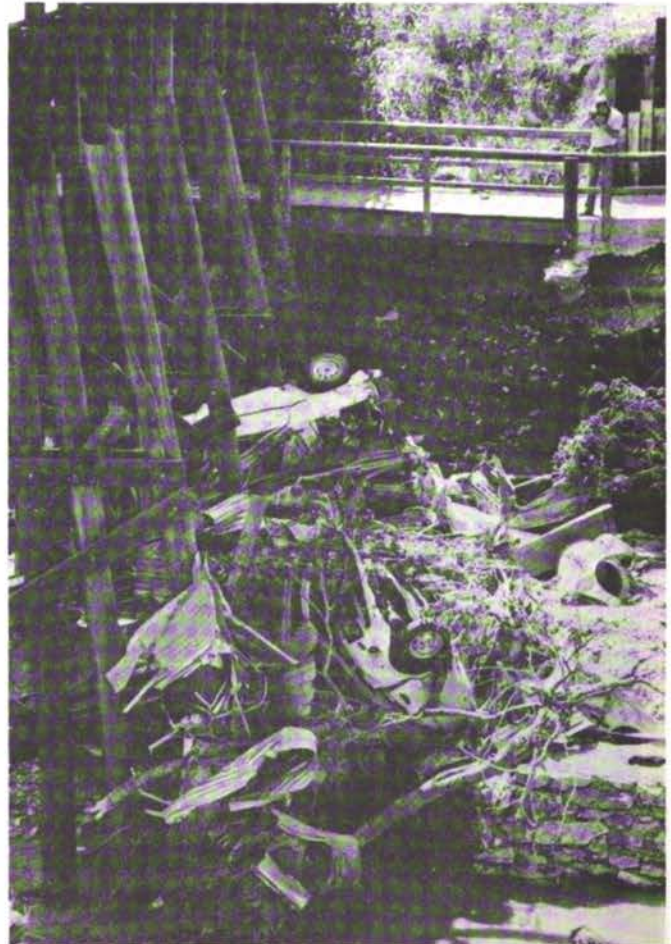
FIGURE 3.5 Debris and automob- iles partially blocking rail- road trestle.
