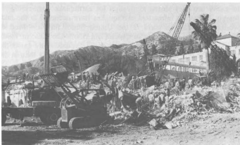
The Sylmar Veterans Administration Hospital collapsed during the 1971 San Fernando, California, earthquake. Forty-nine people were killed in the collapse, and 16 survivors were dug out of the ruins. This photograph was taken 2-1/2 days after the earthquake, just before the last survivor was found.
