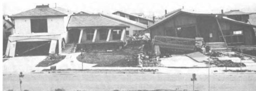
These split-level houses were damaged by the 1971 San Fernando earthquake. In this type of structure, part of the house is built above the garage, so special bracing is needed to resist seismic forces.
