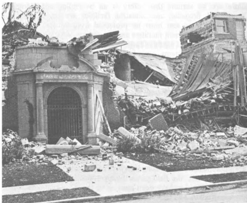
The magnitude 6.3 earthquake of March 10, 1933, in Long Beach, California, damaged many school buildings, such as the high school shown here. It occurred late on a Friday afternoon when no students were in the schools, though some 200 people were killed in other buildings. This earthquake marked the beginning of earthquake engineering in the United States.
