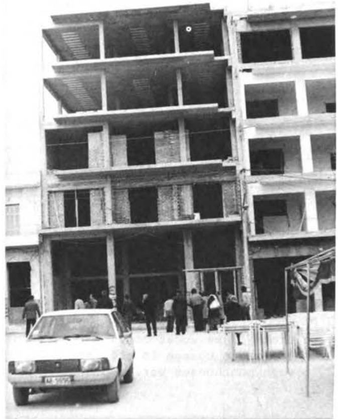
FIGURE 4.17 Flat slab construction without any stiffening walls in Megara. The brick walls were constructed afterward. The building suffered considerable damage with permanent deformations.
