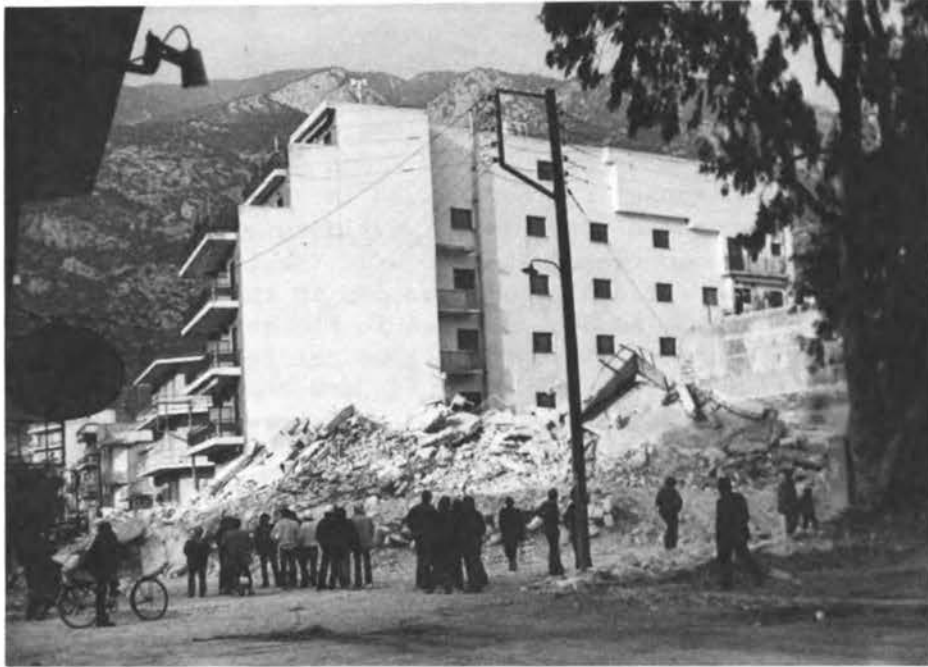
FIGURE 6.8 Contis Hotel in Loutraki. Southwest view one week after collapse. Photograph courtesy A. Manis.
