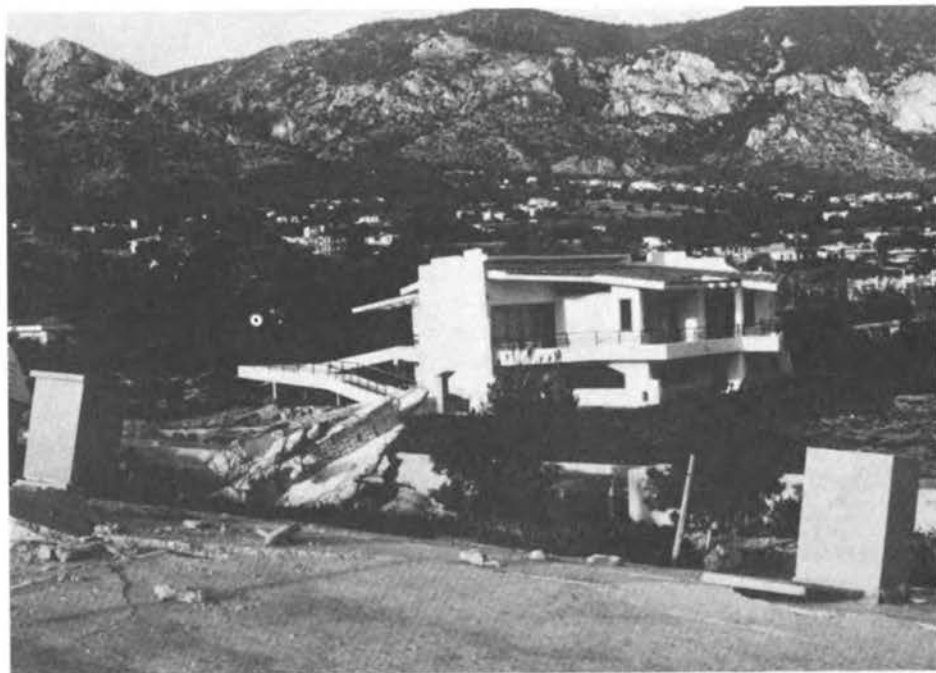
FIGURE 5.36 Column stubs on roof of Kineta hotel to accommodate future expansion. Home in background was undamaged.
