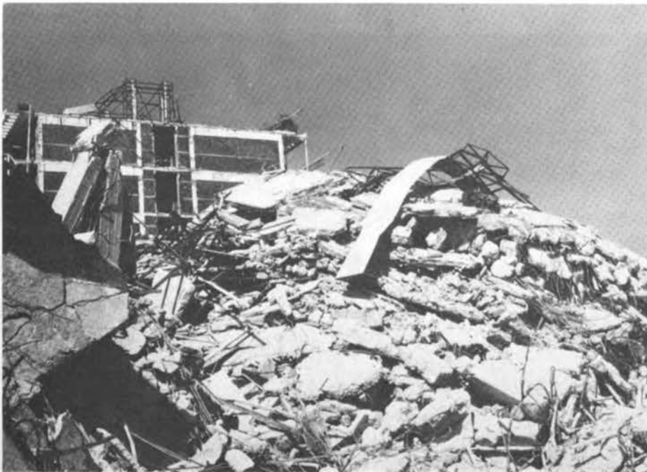
FIGURE 5.26 Collapse of nearly completed hotel in Vrahati.
