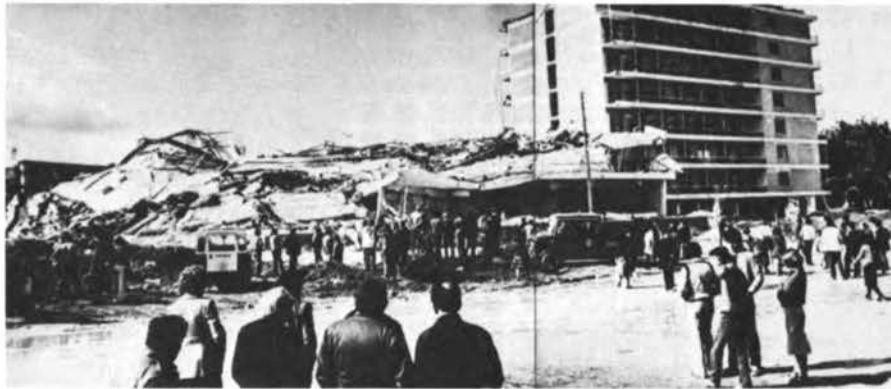
FIGURE 6.20 Galaxy Hotel in Vrahati. View from the east one day after the earthquake and collapse. Photograph courtesy N. Floros.
