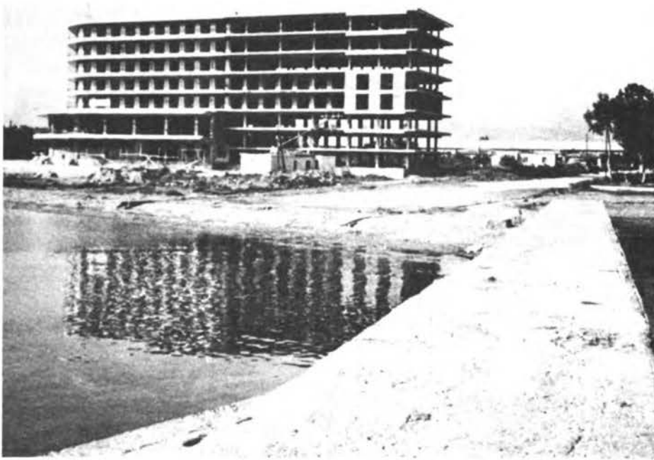
FIGURE 6.18 Galaxy Hotel in Vrahati. North view of the hotel after the earthquake. The remaining part of section III is shown in Figure 6.14a and 6.14b.
