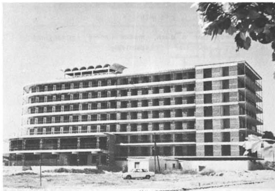
FIGURE 6.17 Galaxy Hotel in Vrahati. North view of the hotel during construction.
