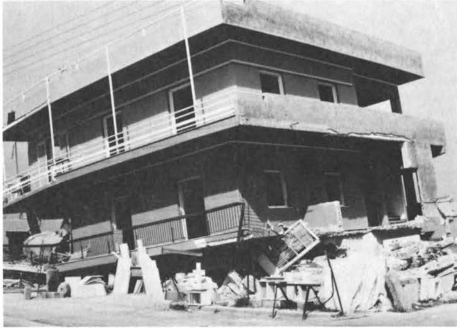
FIGURE 5.21 Collapse of three-story house in Kiato. (Lower floor was stone mason's shop.)
