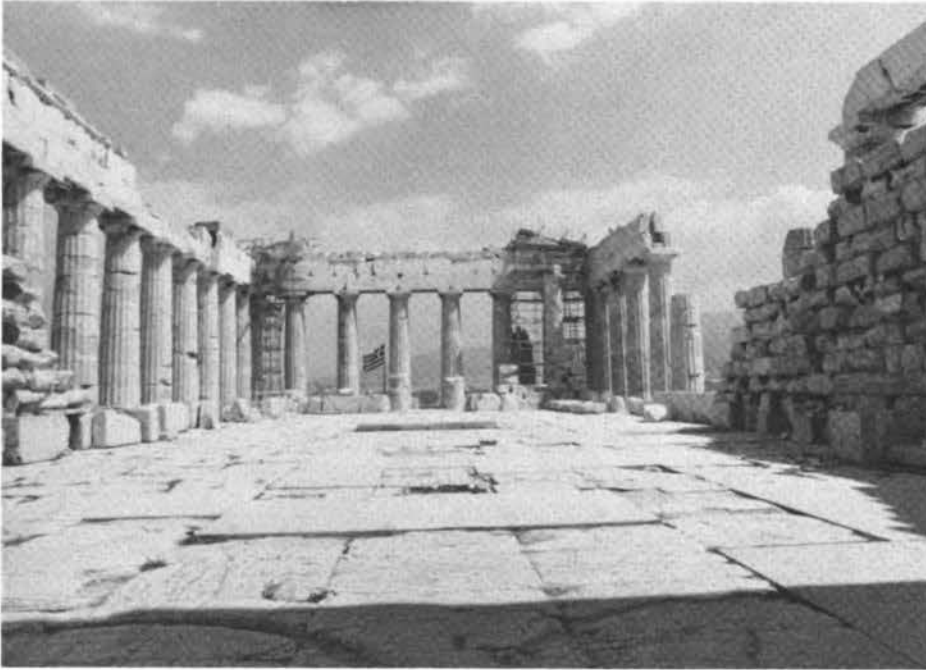
FIGURE 6.45 East side of the Parthenon viewed from the inside. The head beam is supported horizontally only at its two ends. The most damage was concentrated around these two points. Source: Dontas (1981).
