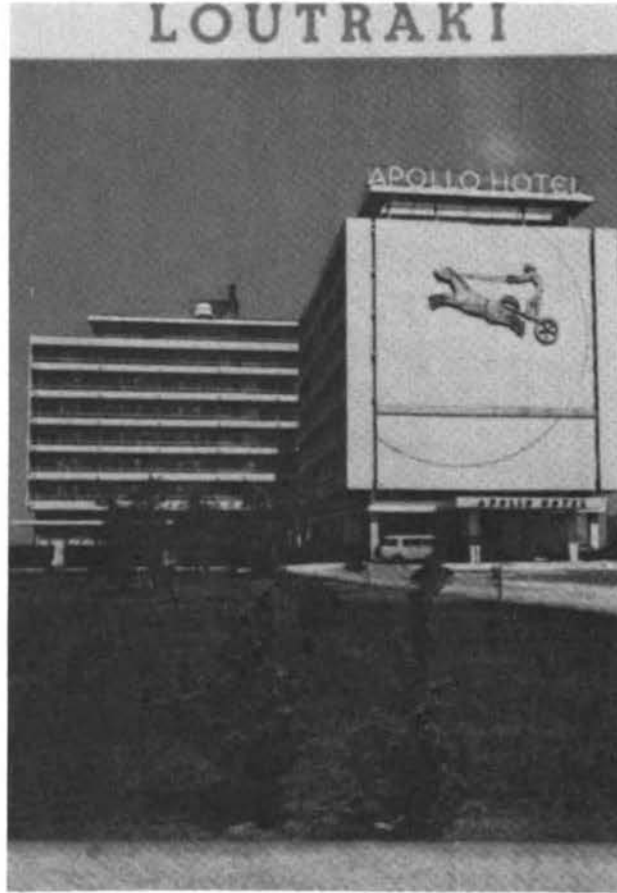
FIGURE 6.27 Apollo Hotel in Loutraki. View from the southeast before the earthquake.
