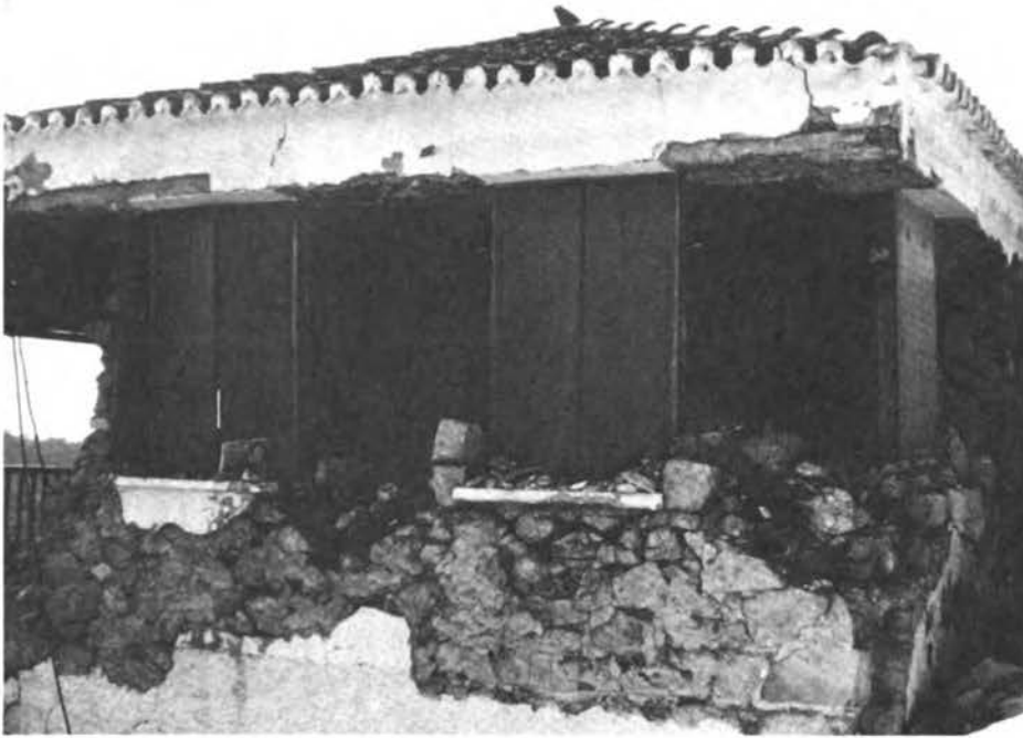
FIGURE 4.1 Tile roof supported by timber frame in Perahora.
