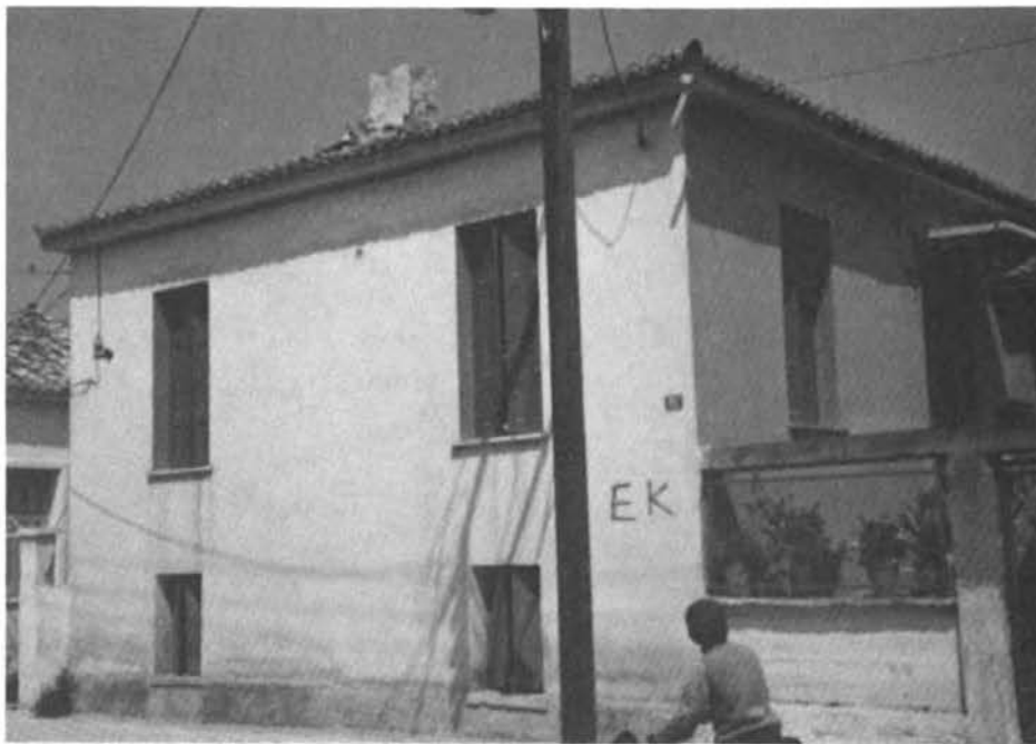
FIGURE 5.28 Some well-maintained earthen buildings in the area, including this one in Kiato, suffered no damage.
