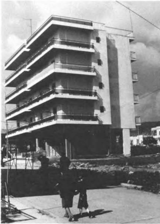
FIGURE 5.51 New apartment building in Athens (Anthoupolis region).
