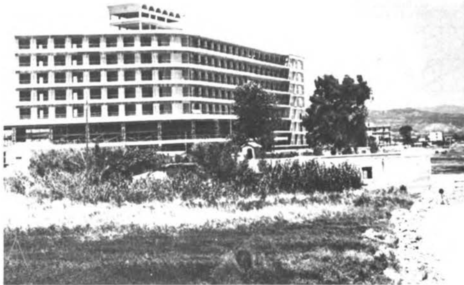
FIGURE 6.16 Galaxy Hotel in Vrahati. Northeast view of the hotel during construction.
