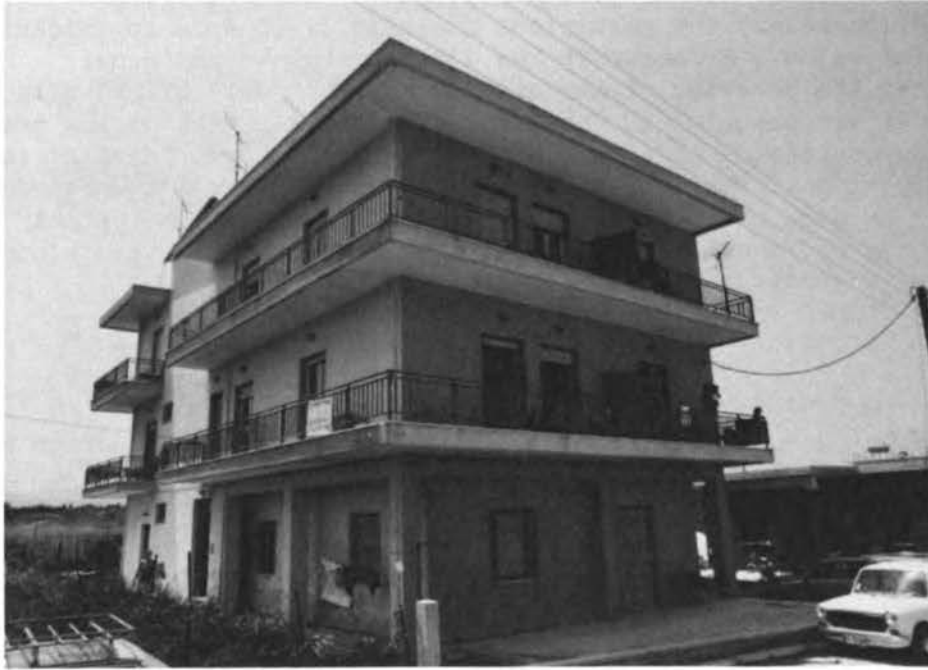
FIGURE 4.7 Undamaged building in Vrahati, founded on silty soil and mud. There is a small brook at left. The building is an addition to an old one in height and length. The old one is made of very good quality concrete blocks, produced locally by the owner. The mortar used for the masonry of these concrete blocks is cement and sand.
