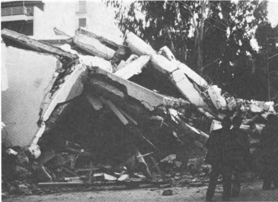
FIGURE 5.6 Collapse of Contis Hotel in Loutraki.
