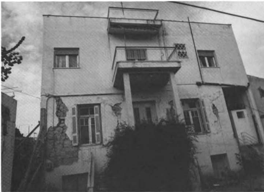
FIGURE 4.4 Additions are very vulnerable, as in this case in Megara. Usually the old building (the lower one) suffers most of the damage.
