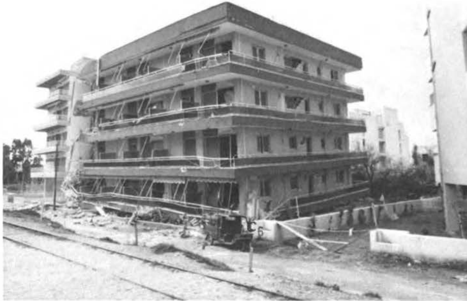
FIGURE 6.38 Block of Flats Segas in Loutraki. The structure from the northeast.
