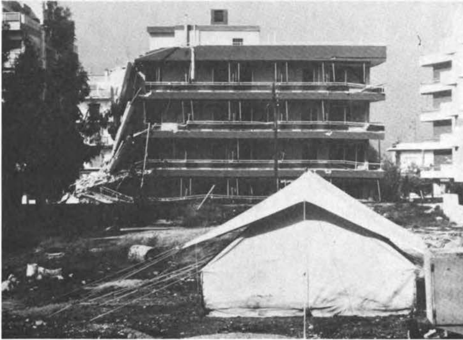
FIGURE 5.2 Partially collapsed five-story block of flats "Segas" in Loutraki. (Note temporary tent shelters in foreground.)
