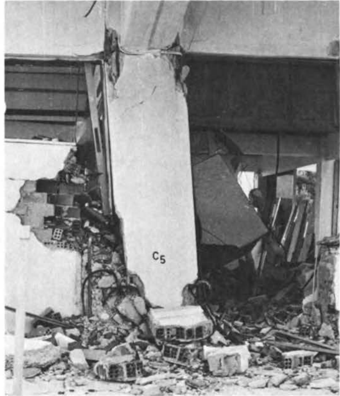
FIGURE 6.6 Vip's Hostel in Perahora. Column c_5 on the second story, viewed from the southeast.
