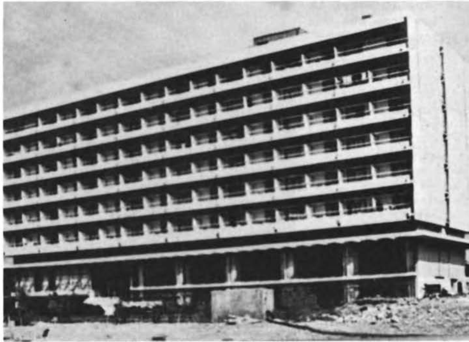
FIGURE 6.29 Apollo Hotel in Loutraki. View from the sea on the west side.
