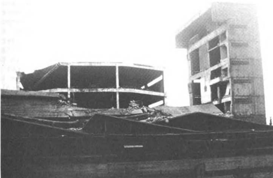
FIGURE 5.38 Ceramic factory near Isthmia (front view, with elevator shaft on right).
