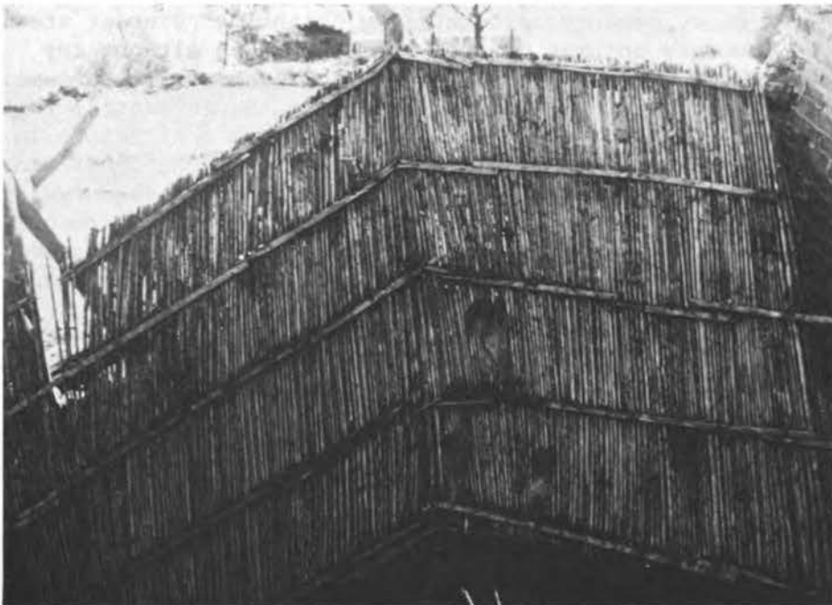
FIGURE 4.2 Timber roof supporting tiles in Perahora.
