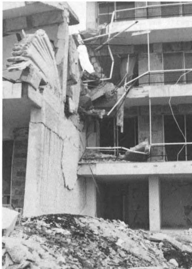
FIGURE 6.21 Galaxy Hotel in Vrahati. North side of the expansion joint between sections II and III.
