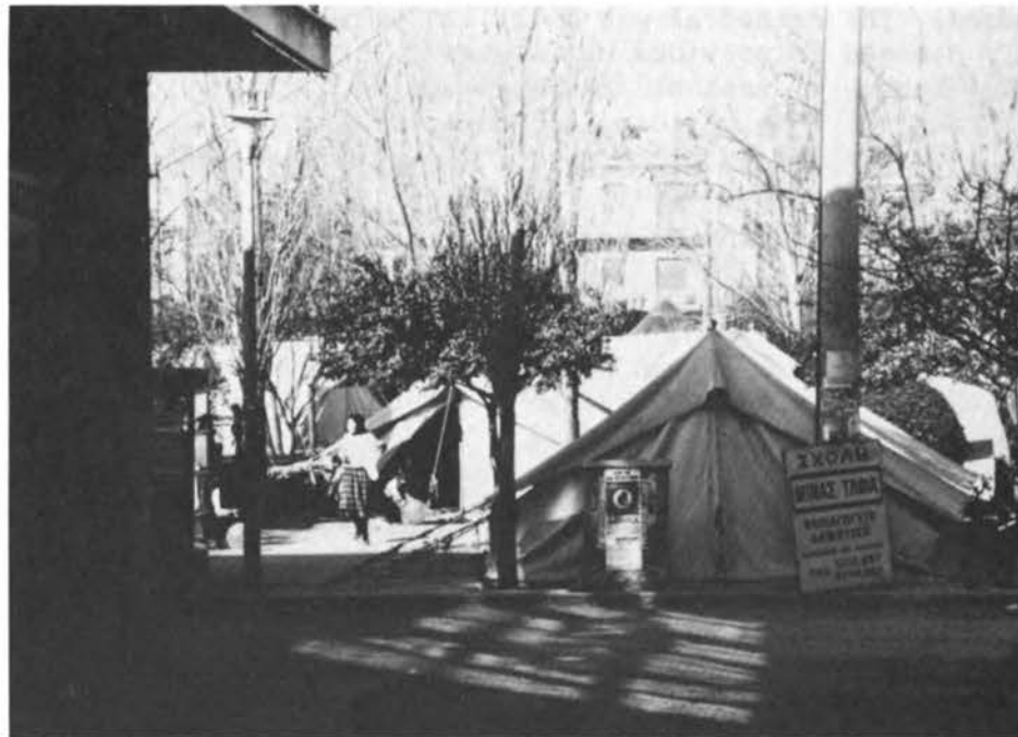
FIGURE 5.48 Temporary tent housing in Athens.
