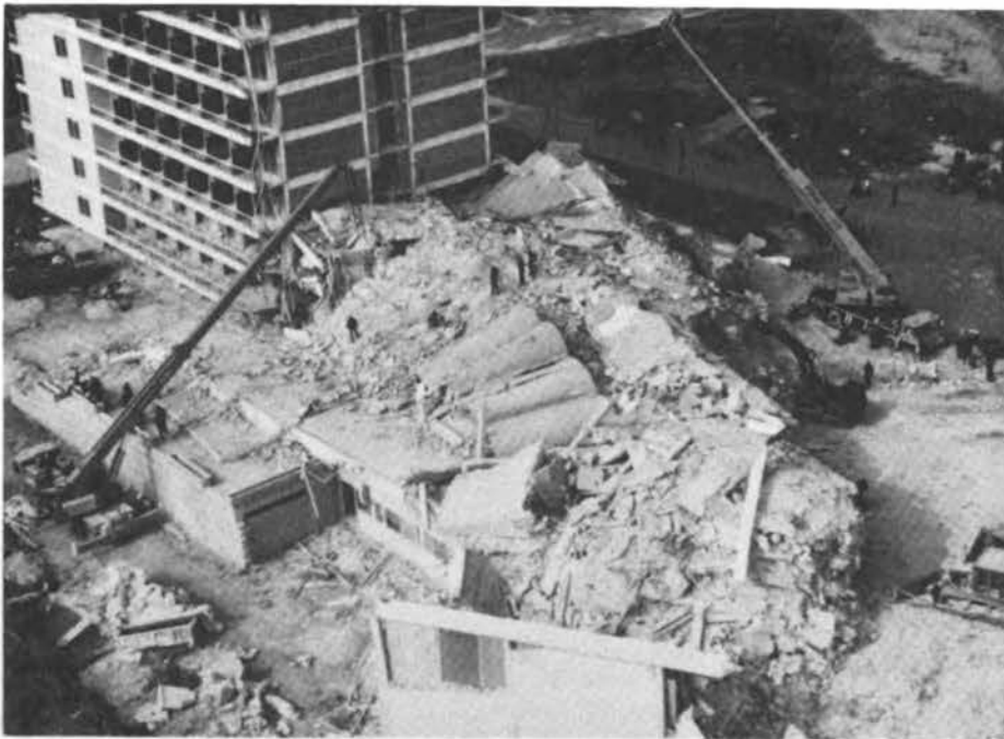
FIGURE 6.19 Galaxy Hotel in Vrahati. Aerial view from the south of the collapsed sections I and II (see Figure 6.14) a few days after the earthquake. Photograph courtesy Tachydromos magazine.
