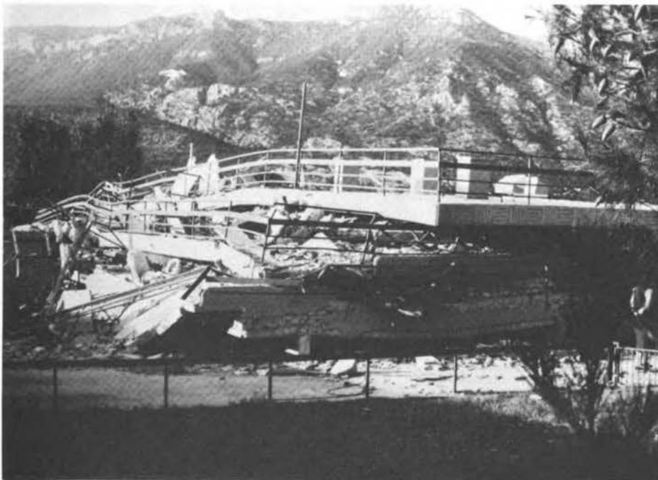
FIGURE 5.34 Collapsed hotel in Kineta.
