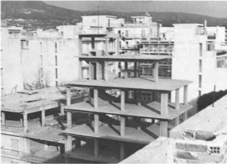
FIGURE 4.15 Eccentrically located walls in reinforced concrete frame under construction. This is a typical example of a drastic change in the plan area in a penthouse. Collapses of such penthouses were reported.
