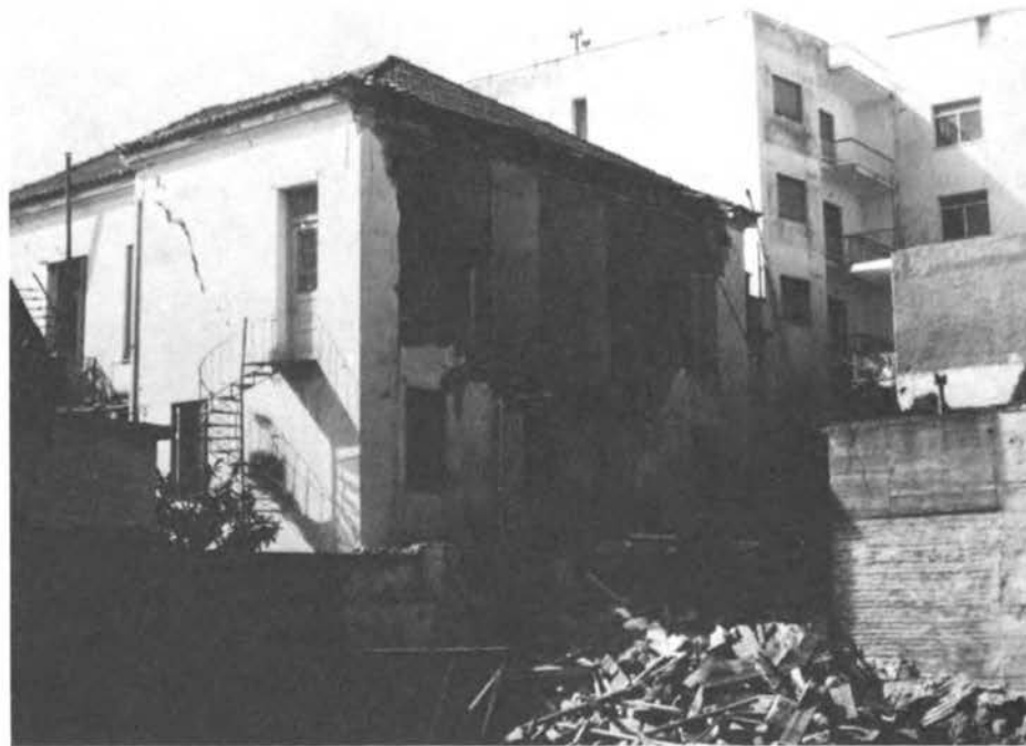
FIGURE 5.22 Older stone wall buildings in Vrahati.
