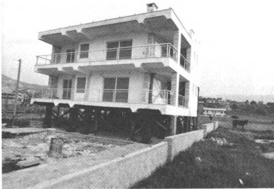
FIGURE 4.33 Modern resort apartment building in Alepohori with open first story. The damage was limited to the lower story. The heavy scaffolding (placed after the earthquake) consists of H-shaped steel beams.
