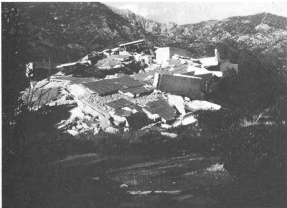
FIGURE 5.30 Collapse of Kineta bungalows.
