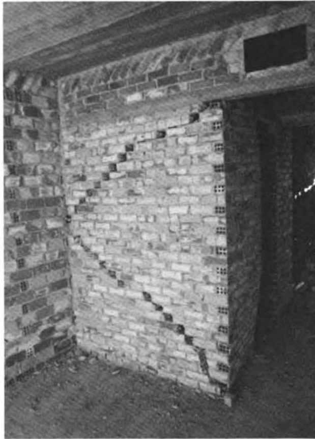
FIGURE 4.9 Unreinforced hollow brick wall in an apartment building.
