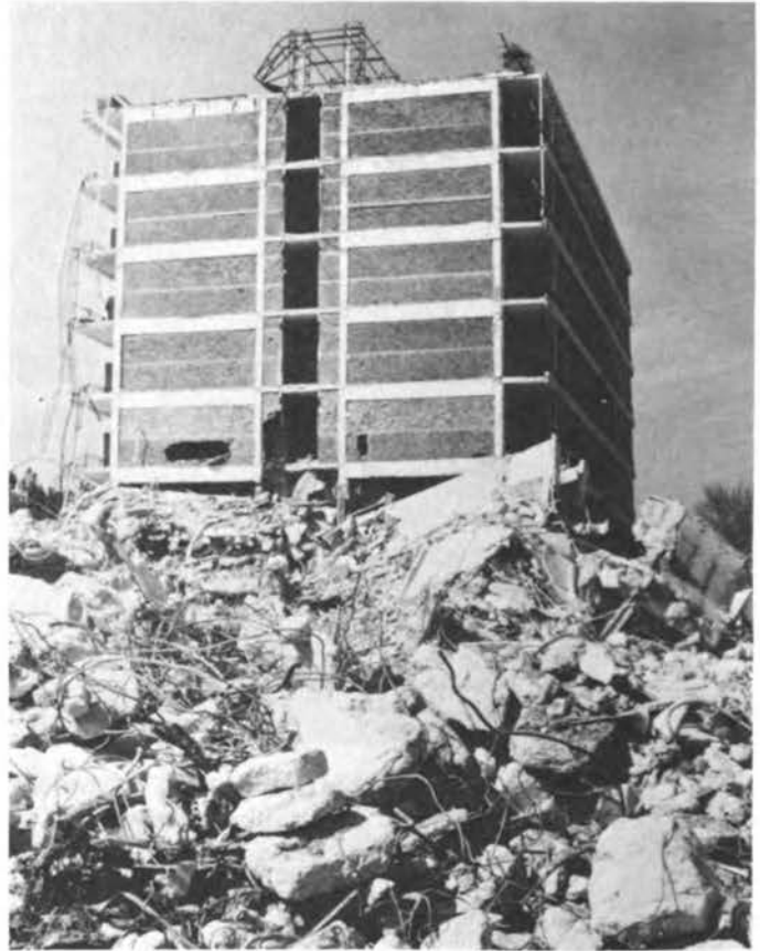
FIGURE 5.27 Portion of hotel standing (an expansion joint separated the sections).
