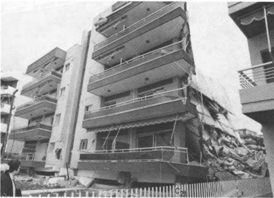
FIGURE 6.37 Block of Flats Segas in Loutraki. The structure from the west.
