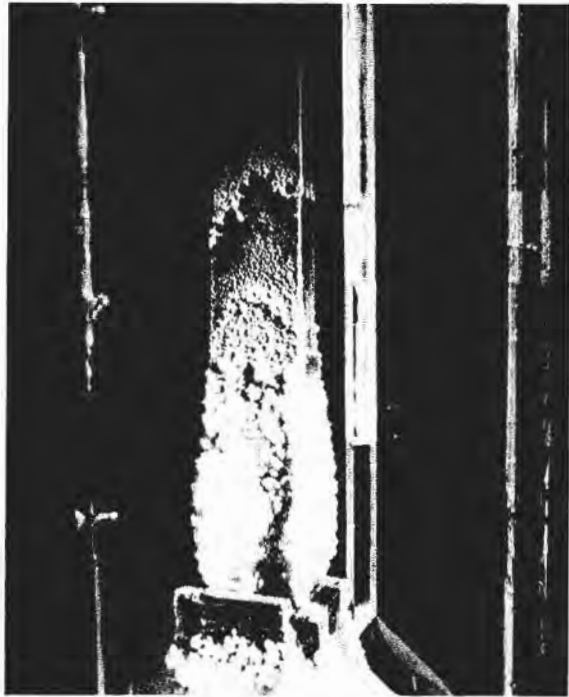
FIGURE 3a Sandstone column with encrustation of salt due to migration of solution from the interior of the stone to the surface. The triangular patch near the top shows the height to which sub-surface pores appeared to be wet. Solution was 5.3 M NaCl.
