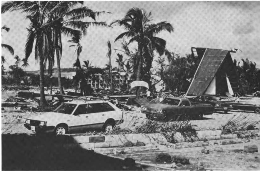
FIGURE 3.18 Damage to Beach House Restaurant at Kuhio Shores, Kauai.
