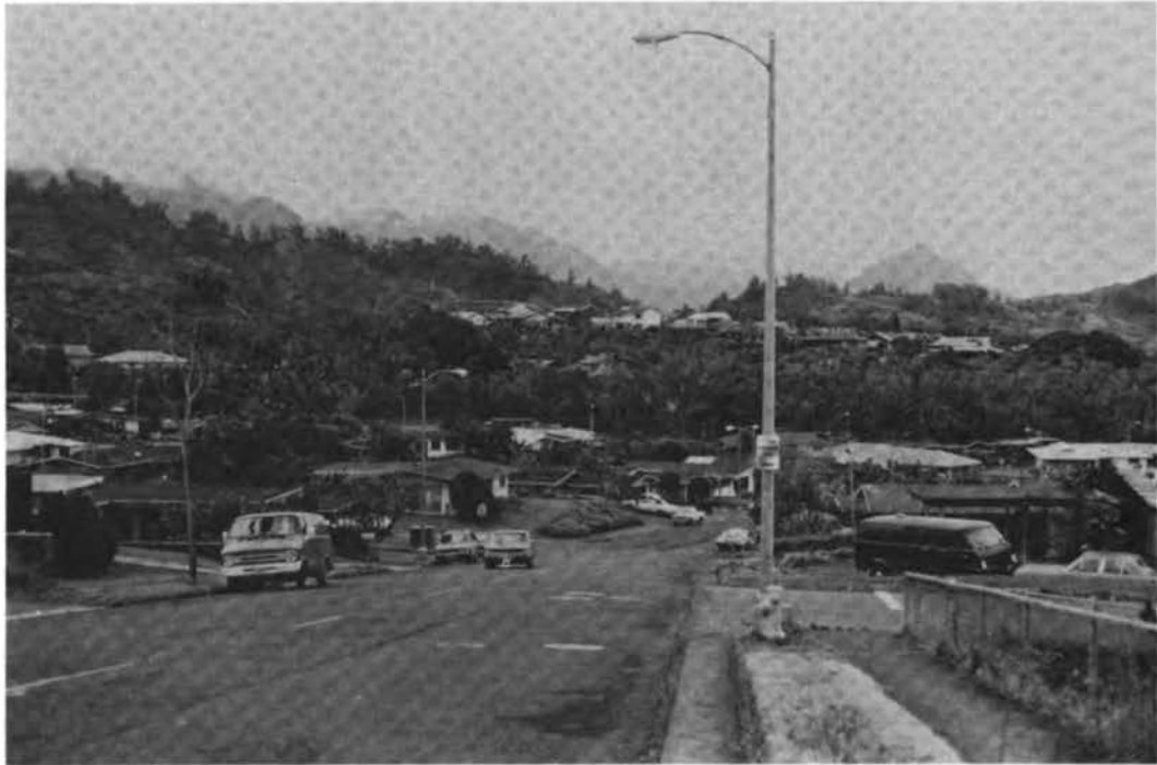
FIGURE 3.86 Roof damage to homes located along ridge line at Kaneohe, Oahu (there was little or no damage to homes not sited along the ridge in this area).
