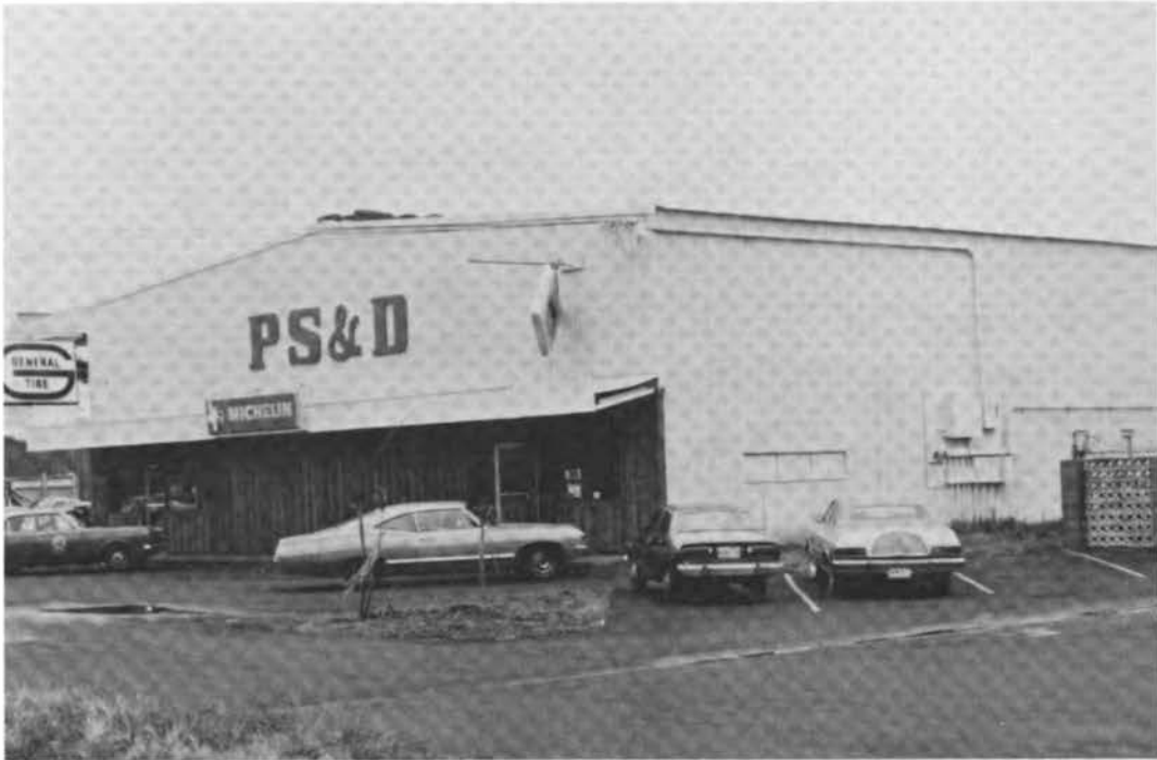
FIGURE 3.55 Undamaged preengineered metal building at Lihue, Kauai.
