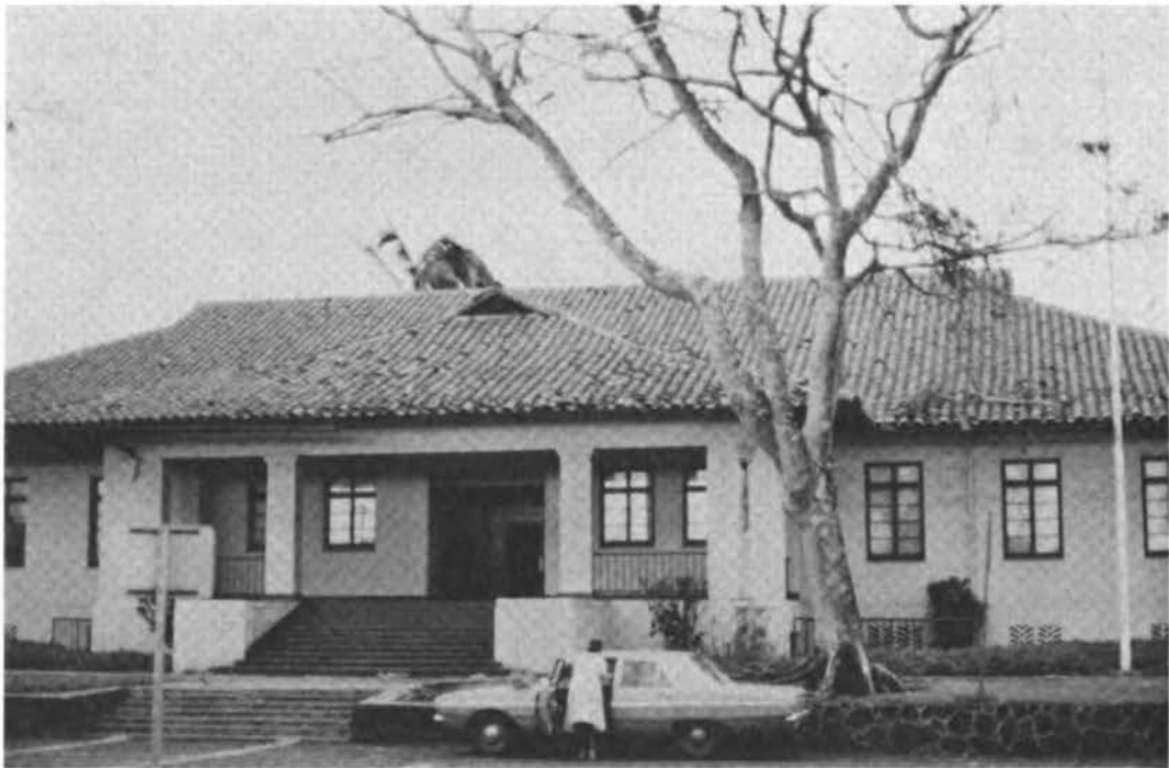
FIGURE 3.52 Minor wind damage to city building at Lihue, Kauai.
