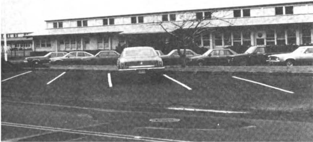
FIGURE 3.53 Undamaged Wilcox Elementary School at Lihue, Kauai.
