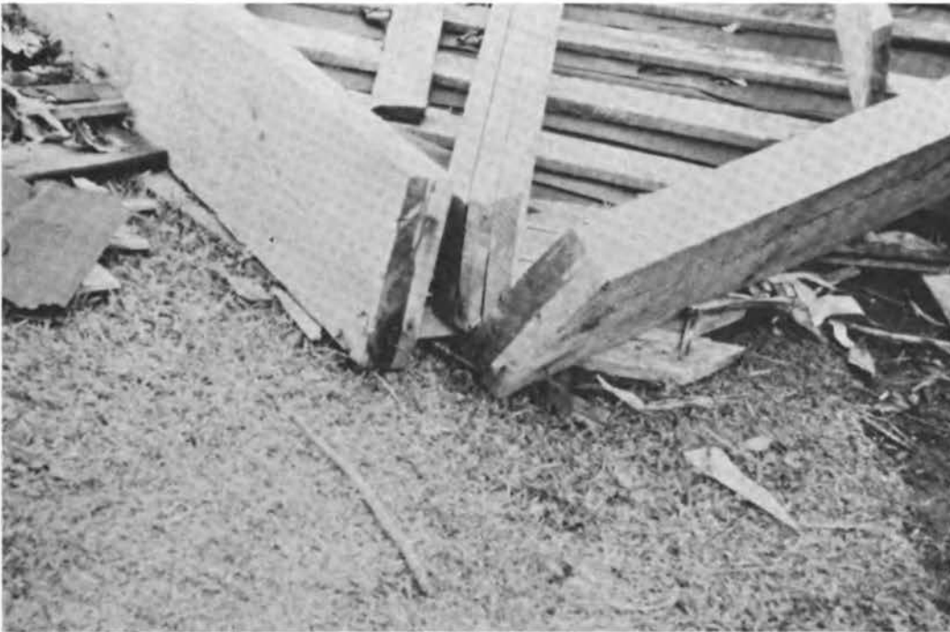
FIGURE 3.69 Fastener details of hip roof.
