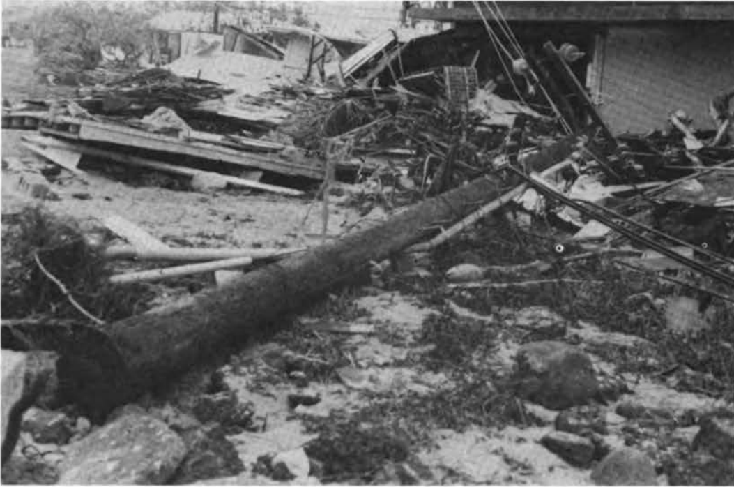
FIGURE 4.3 Power and telephone pole at Poipu, Kauai, that toppled due to soil embedment failure.
