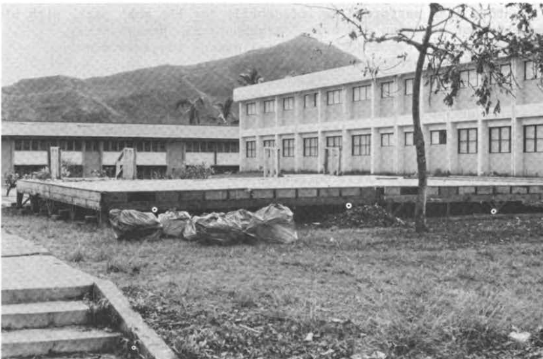
FIGURE 3.48 Kauai High School (site of heavily damaged temporary building).
