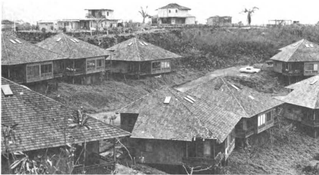
FIGURE 3.41 Minor cladding damage to sheltered condominiums sited in Poipu Crater at Makahuena Point, Kauai.
