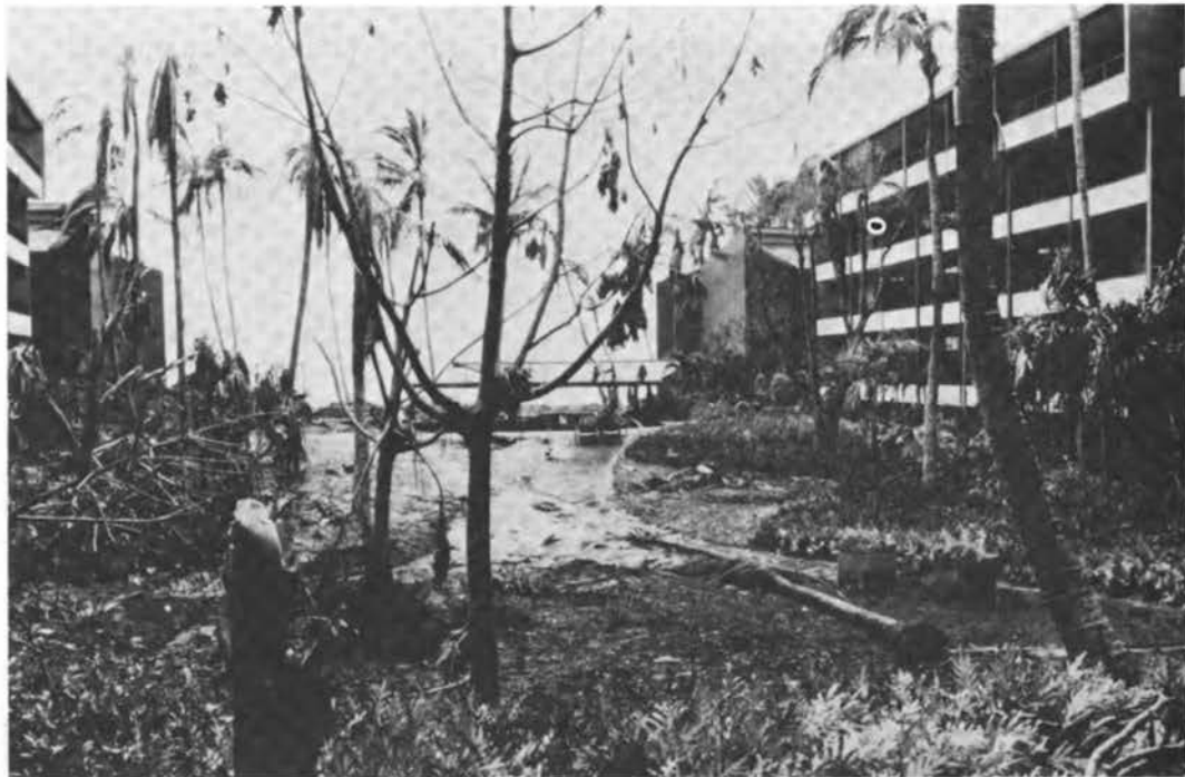
FIGURE 3.31 Wave and flooding damage at Waiohai Hotel, Kauai.
