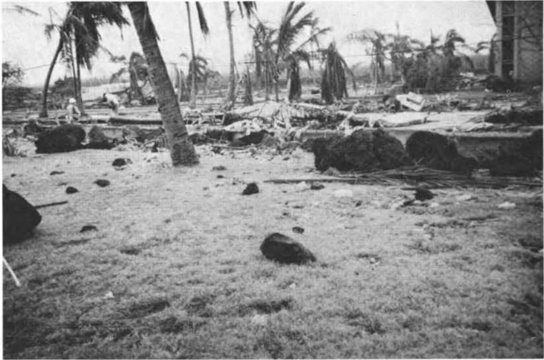
FIGURE 3.30 Waterborne debris at Sheraton-Kauai.
