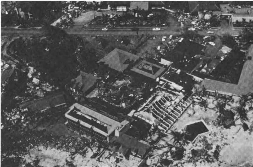
FIGURE 3.2 Damage at Sheraton-Kauai on Poipu Beach.
