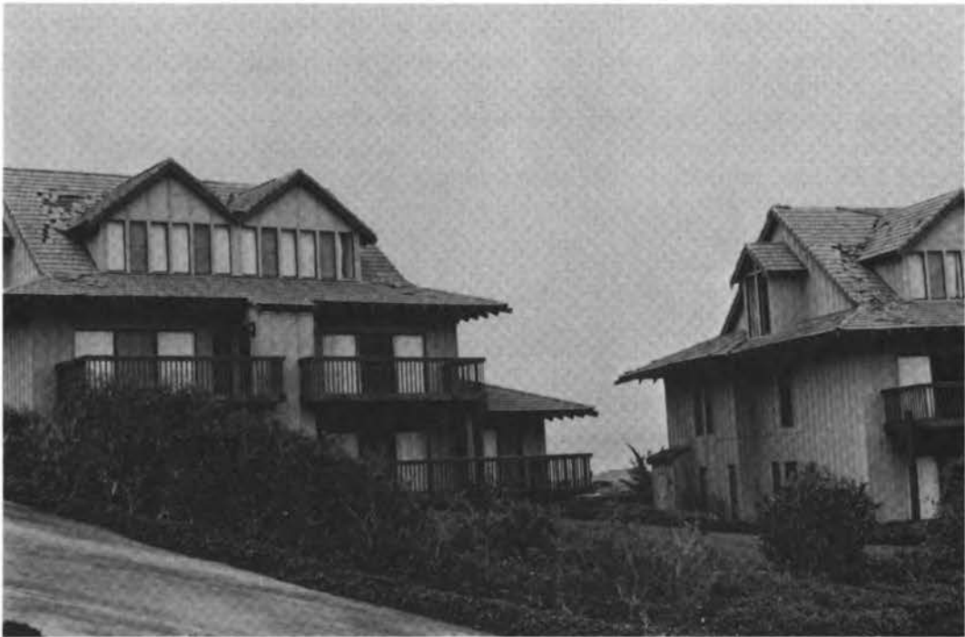
FIGURE 3.40 Minor cladding damage to homes inland from Makahuena Point, Kauai.
