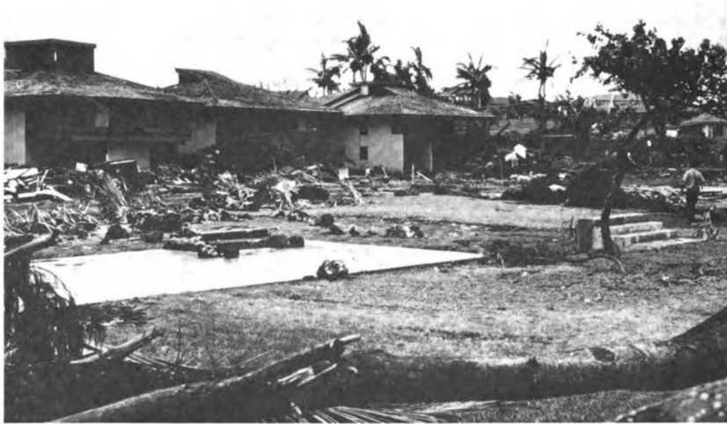
FIGURE 3.13 Damage to beachfront single-family dwellings on Kauai.
