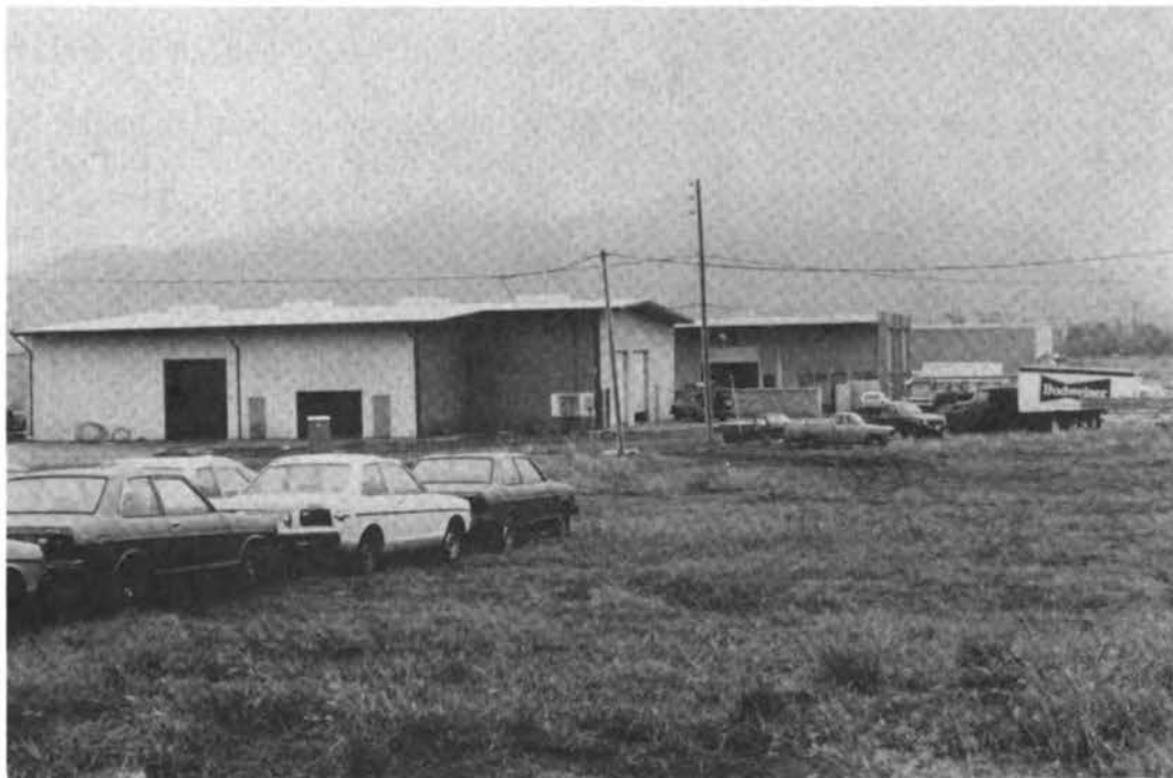
FIGURE 3.10 Preengineered metal buildings at Kauai (no observed damage).
