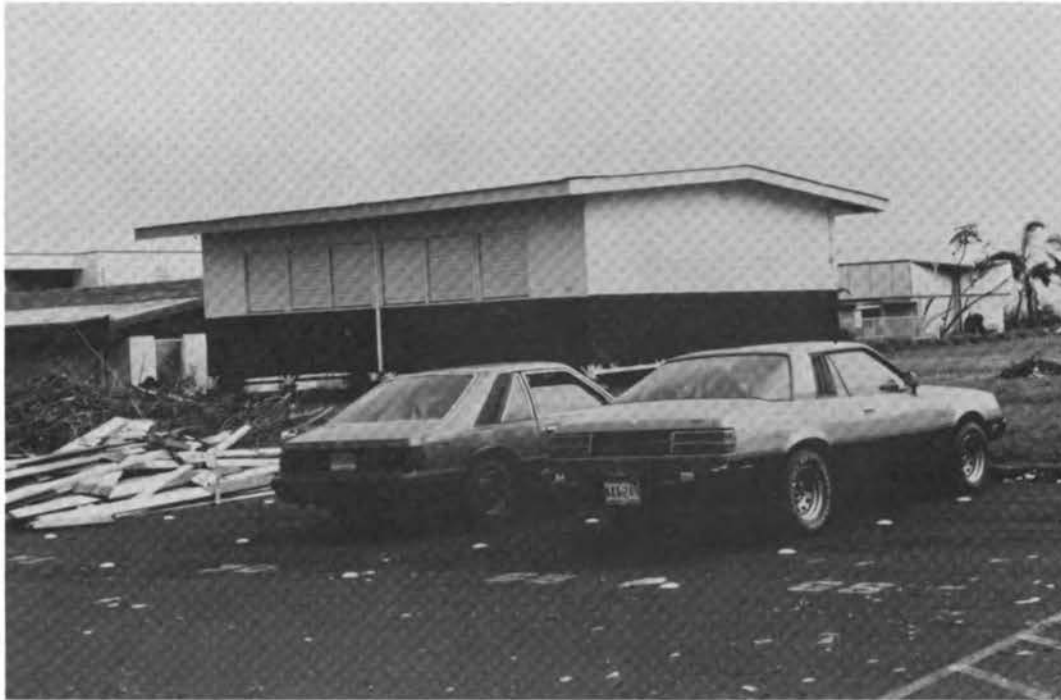
FIGURE 3.49 Undamaged bungalow unit at Kauai High School.
