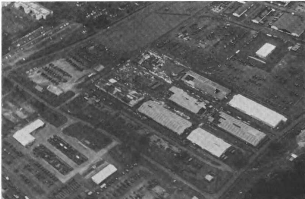
FIGURE 3.8 Damage to warehouse buildings at Schofield Barracks, Oahu.
