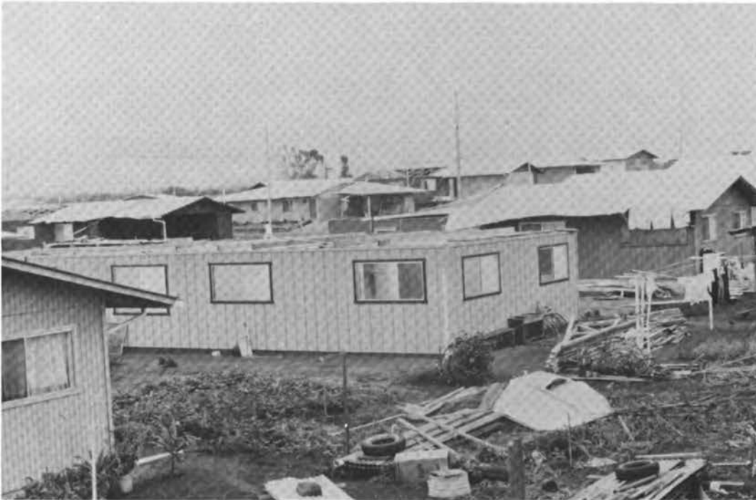
FIGURE 3.5 Damage to residential development at Kapaa Meadows, Kauai.
