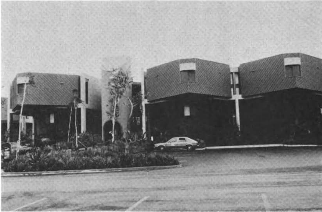
FIGURE 3.63 Undamaged Pu'u Po'a units, Princeville, Kauai.
