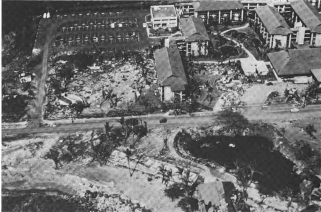
FIGURE 3.24 Damage to Sheraton-Kauai at Poipu Beach due to storm surge, wave action, and wind.
