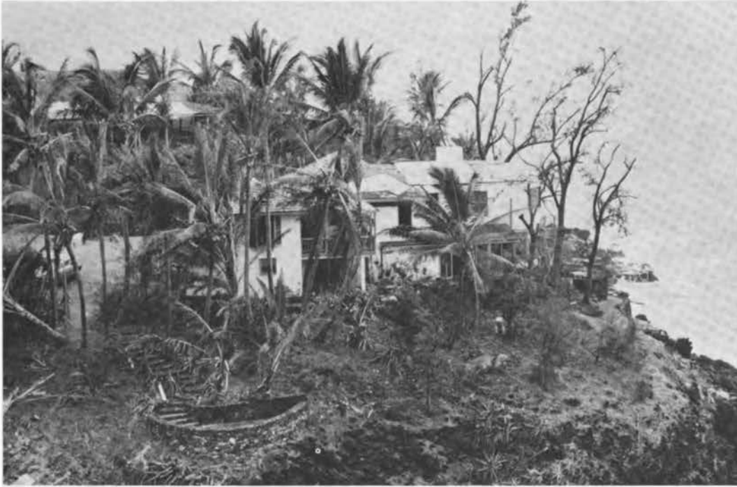
FIGURE 3.37 Wind damage to single-family dwelling on bluff at Makahuena Point, Kauai.
