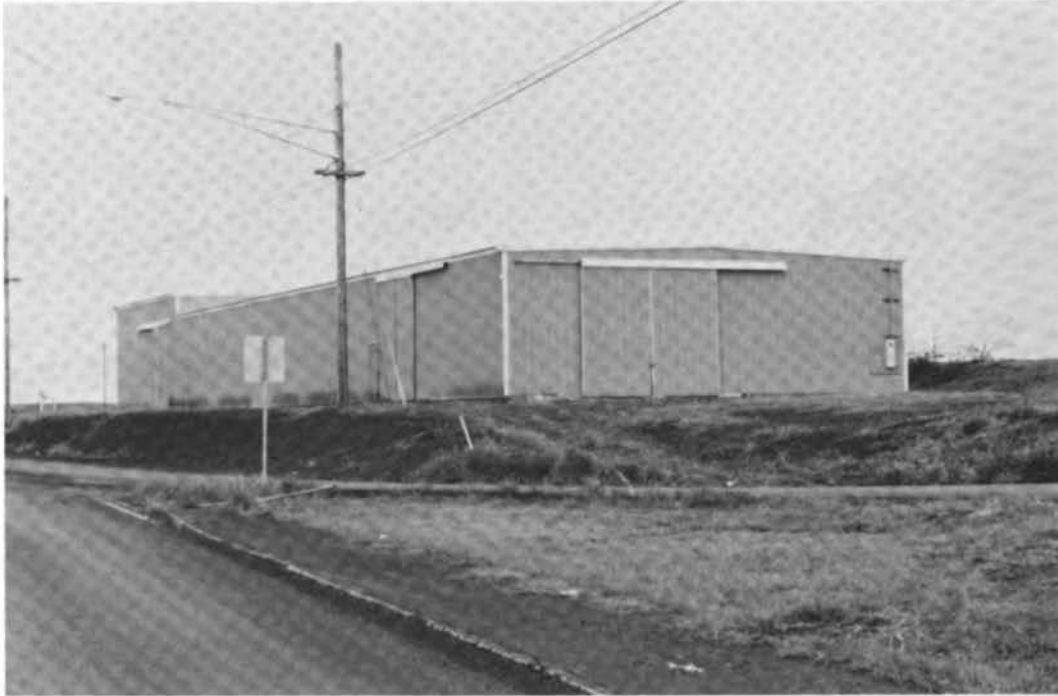
FIGURE 3.83 Undamaged preengineered metal building located on Kamehameha Highway near Wahiawa, Oahu.
