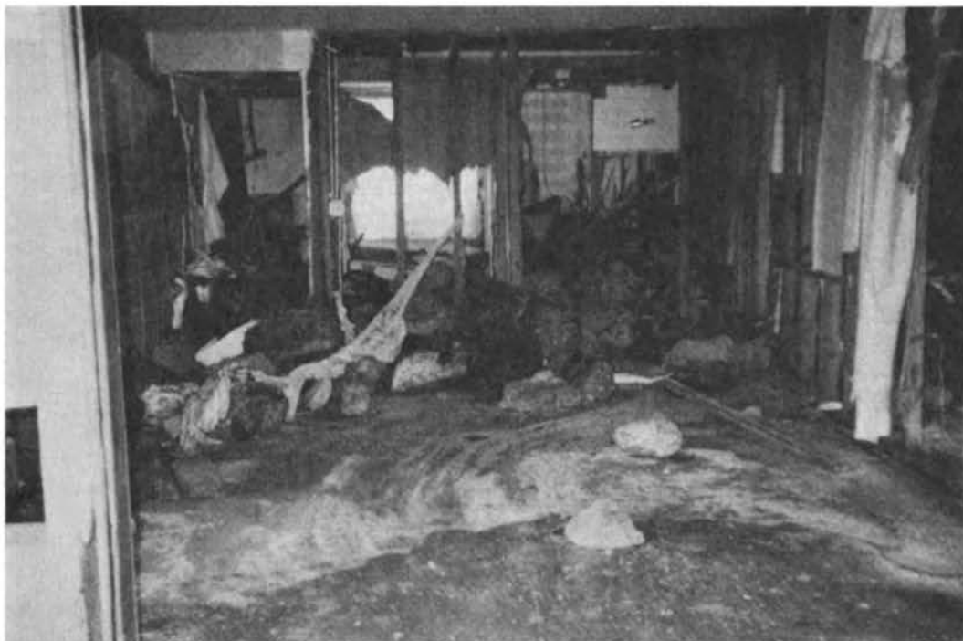
FIGURE 3.29 Storm surge, wave, and flooding damage to interior of unit at Sheraton-Rauai.
