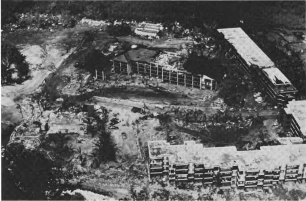
FIGURE 3.17 Damage to Kuhio Shores Resort development, Kauai (note proximity of buildings to shoreline).
