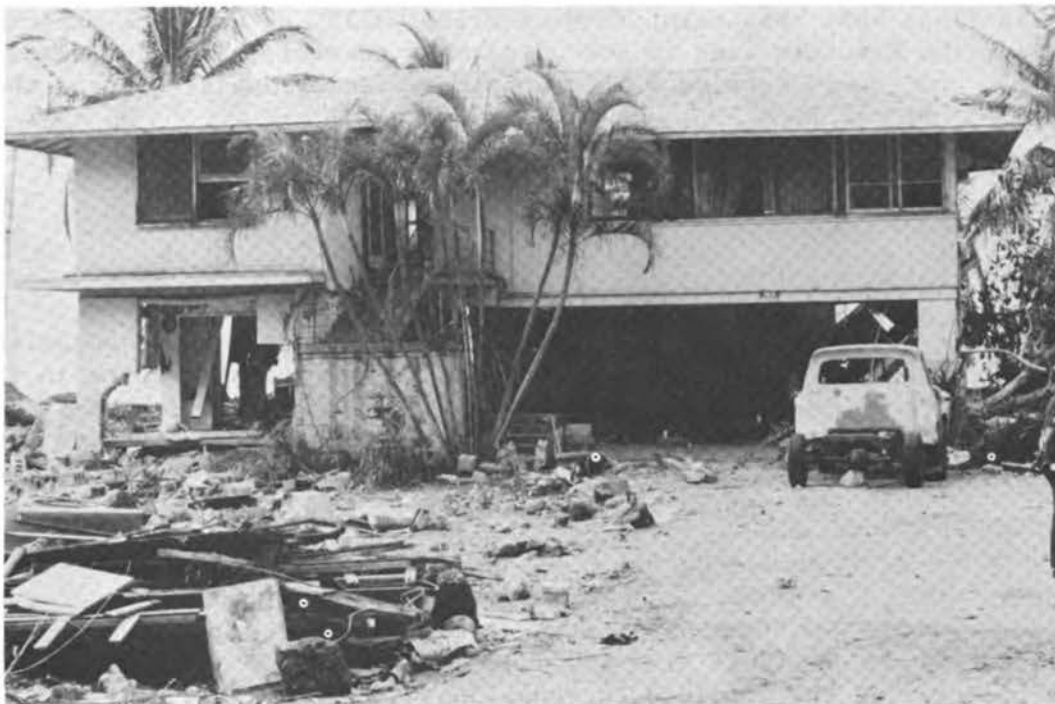
FIGURE 3.74 Damage to single-family dwelling at Makaha, Oahu.
