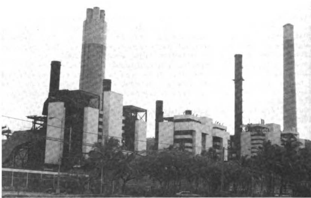
FIGURE 4.2 Undamaged Kahe power plant on the coast of Oahu 4-1/4 miles north of Barbers Point.
