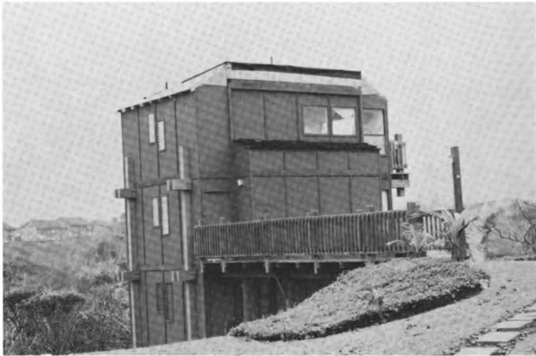
FIGURE 3.67 Pole house type construction of Hanalei Bay Villas at Princeville, Kauai.
