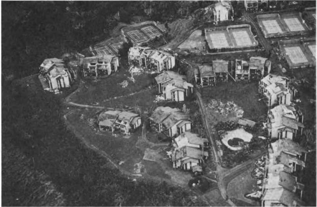
FIGURE 3.70 Damage to Hanalei Bay Resort townhouses (viewed from southeasterly direction).
