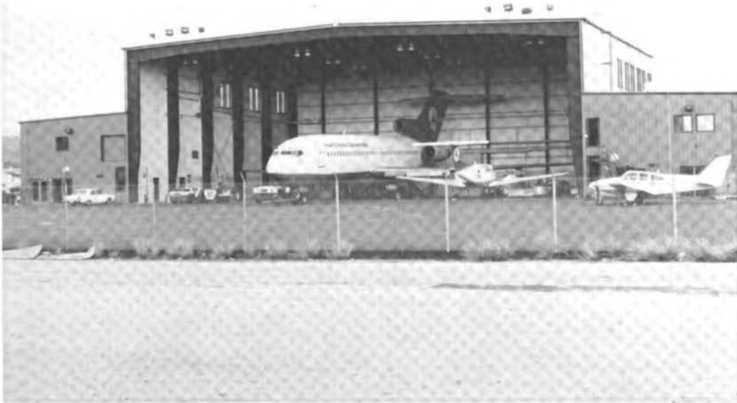
FIGURE 3.77 Undamaged preengineered metal hangar building at Honolulu International Airport (note building was open on windward face for Iwa).
