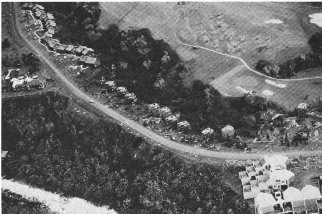
FIGURE 3.62 Aerial view of wind damage at Princeville, Kauai.
