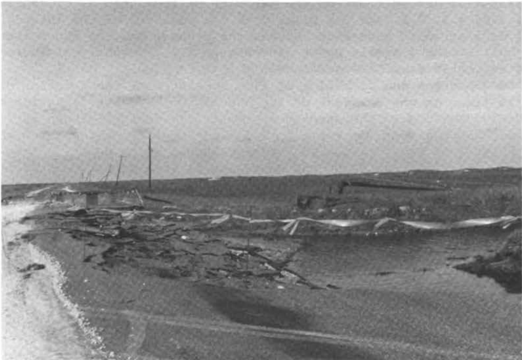
FIGURE 3.8 Washout channel looking south toward the Gulf about 7 miles west of San Luis Pass on Follets Island.
