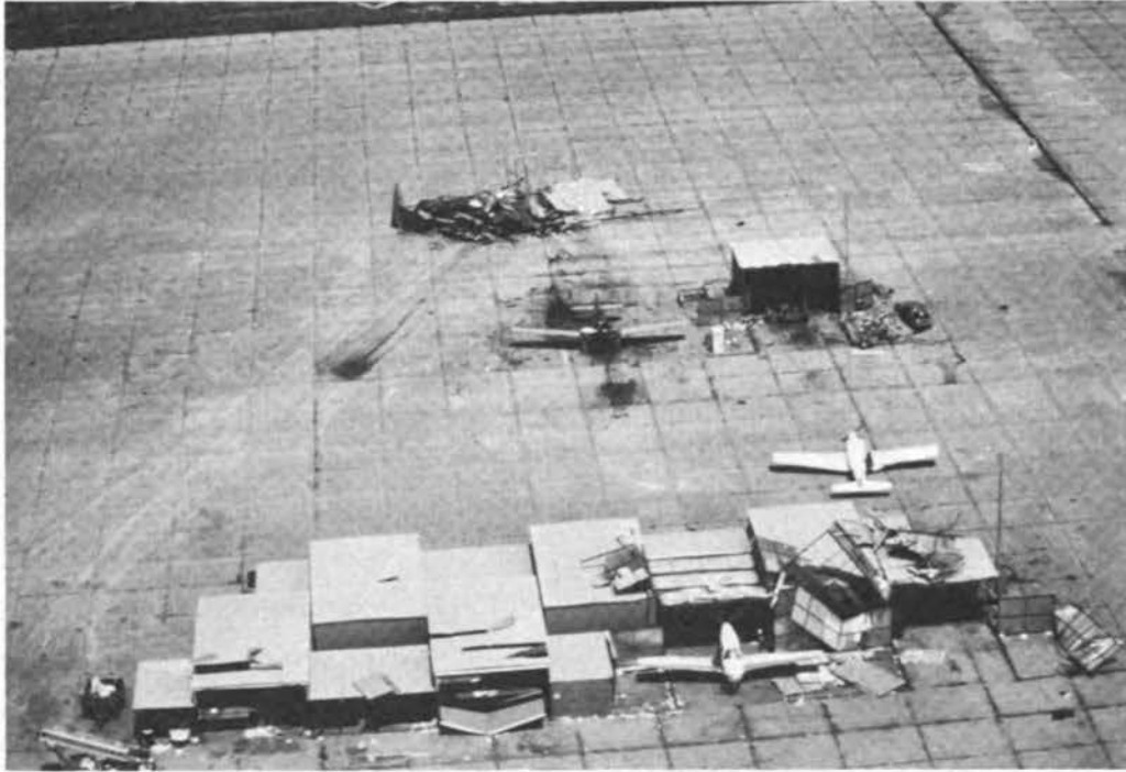
FIGURE 4.38 Damaged hangars and small aircraft at Galveston Airport.
