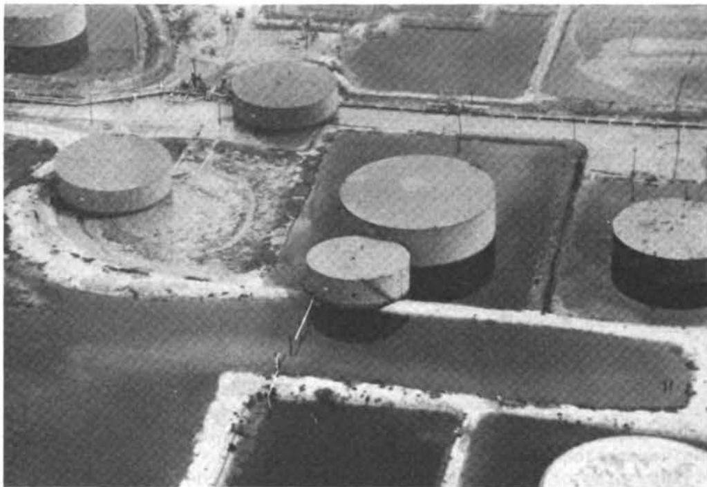
FIGURE 4.18 Displaced oil storage tanks.
