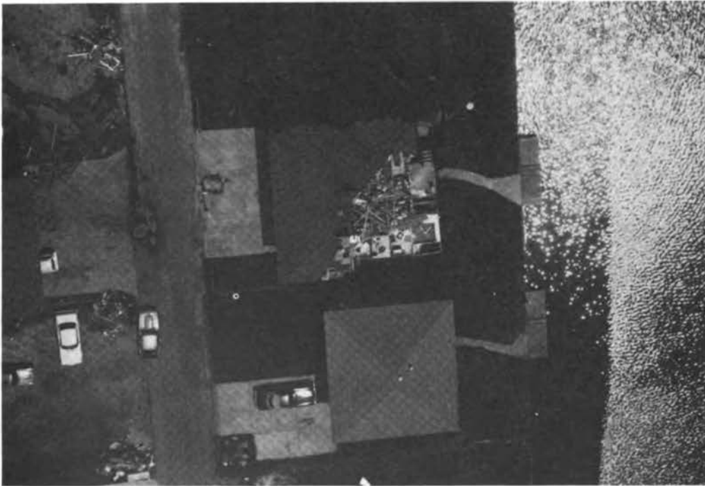
FIGURE 4.54 Aerial view of roof damage.
