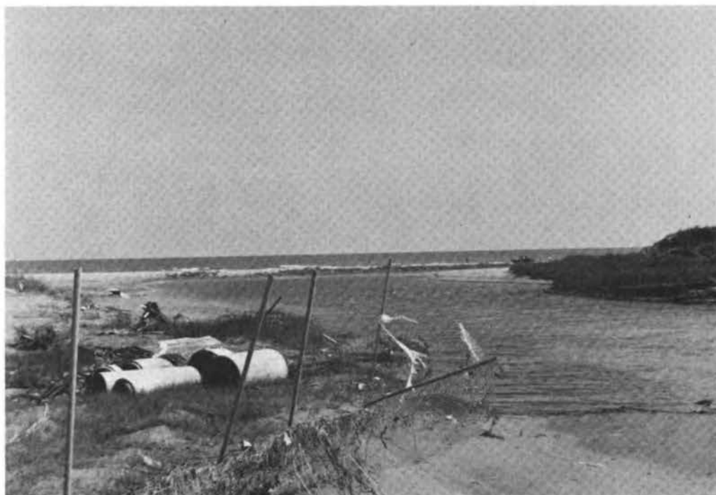
FIGURE 3.6 Landward end of the scour channel shown in Figure 3.5.
