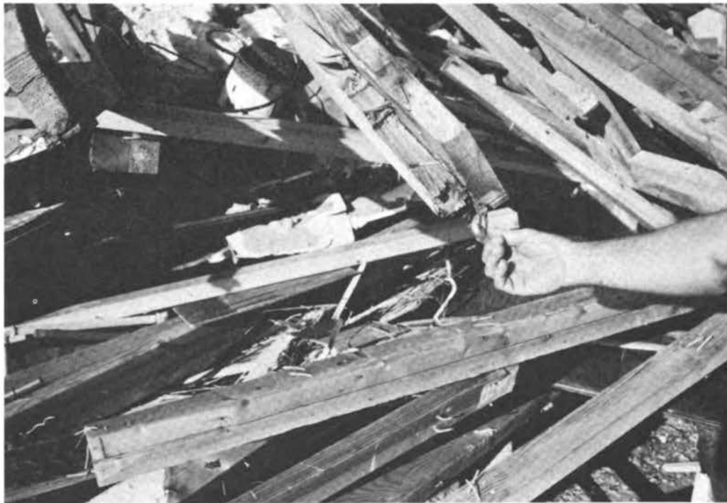
FIGURE 4.44 Details of toe nail connections.
