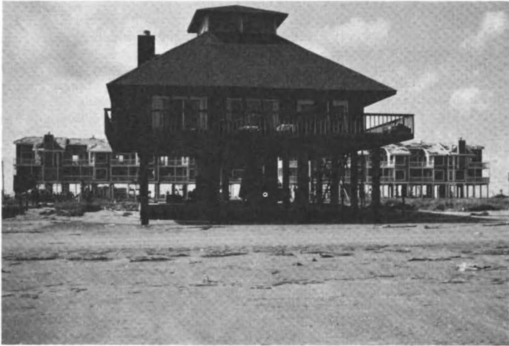
FIGURE 4.51 Example of a well-constructed house that performed very well except for erosion around the foundation.
