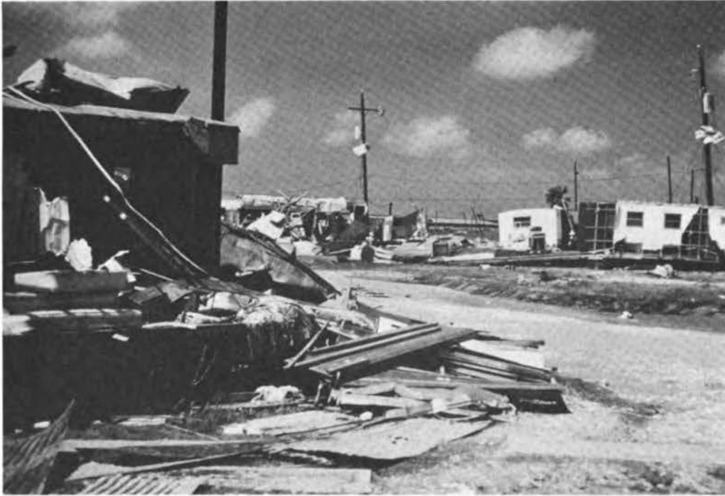
FIGURE 4.26 Damaged mobile home park on East Beach.
