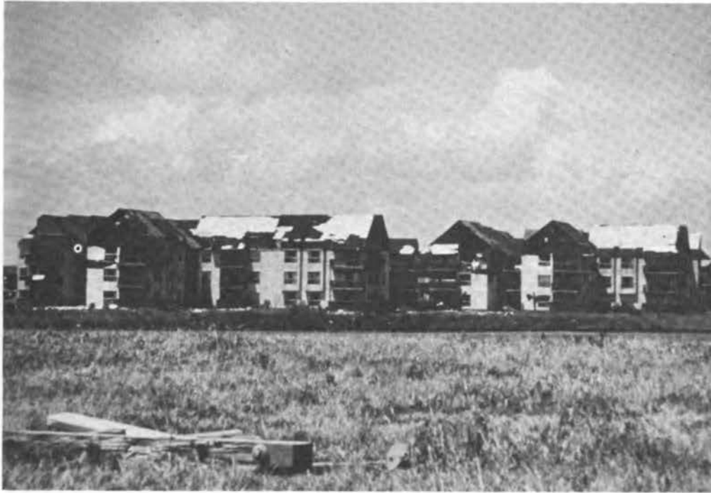
FIGURE 4.32 Roof damage to apartments near the seawall.
