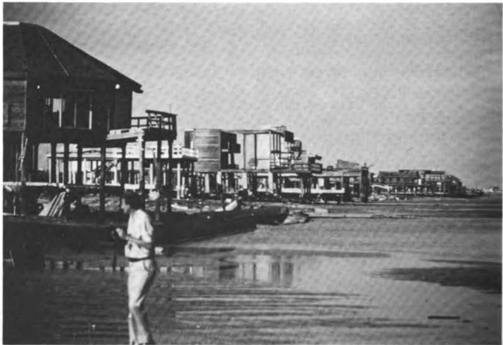
FIGURE 4.40 General view of damaged houses along Terramar Beach.
