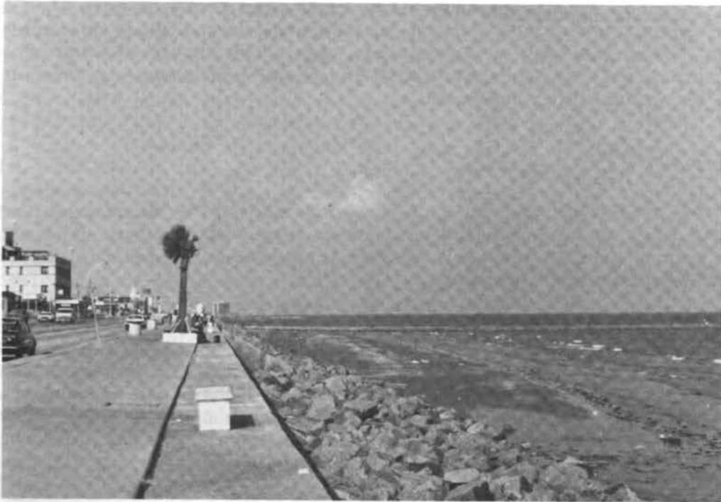
FIGURE 4.56 Galveston seawall and groin.
