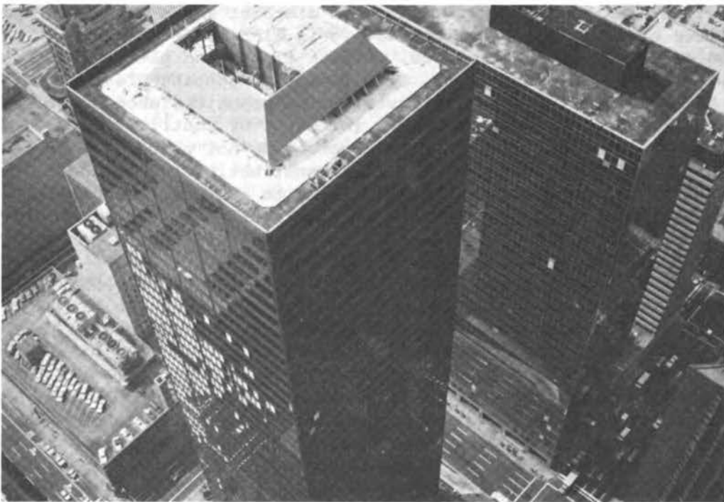
FIGURE 4.12 General view of the roofs of the Milam and Entex buildings.
