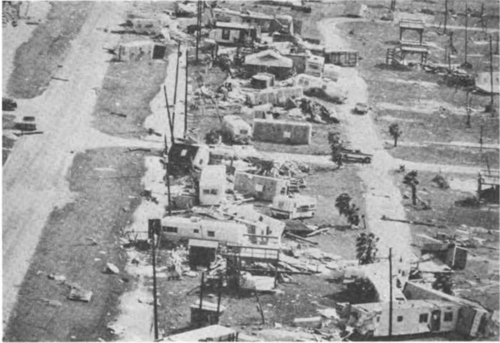
FIGURE 4.28 Damaged mobile home park on West Beach.
