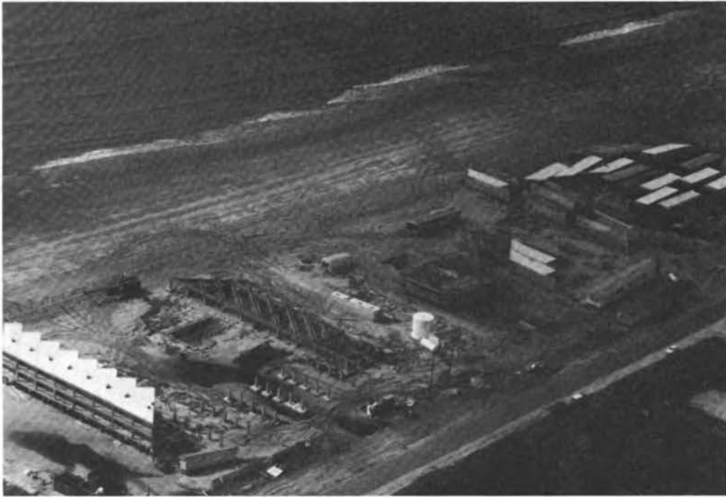
FIGURE 4.53 General view of a modular condominium project that experienced damage from wind and storm surge.
