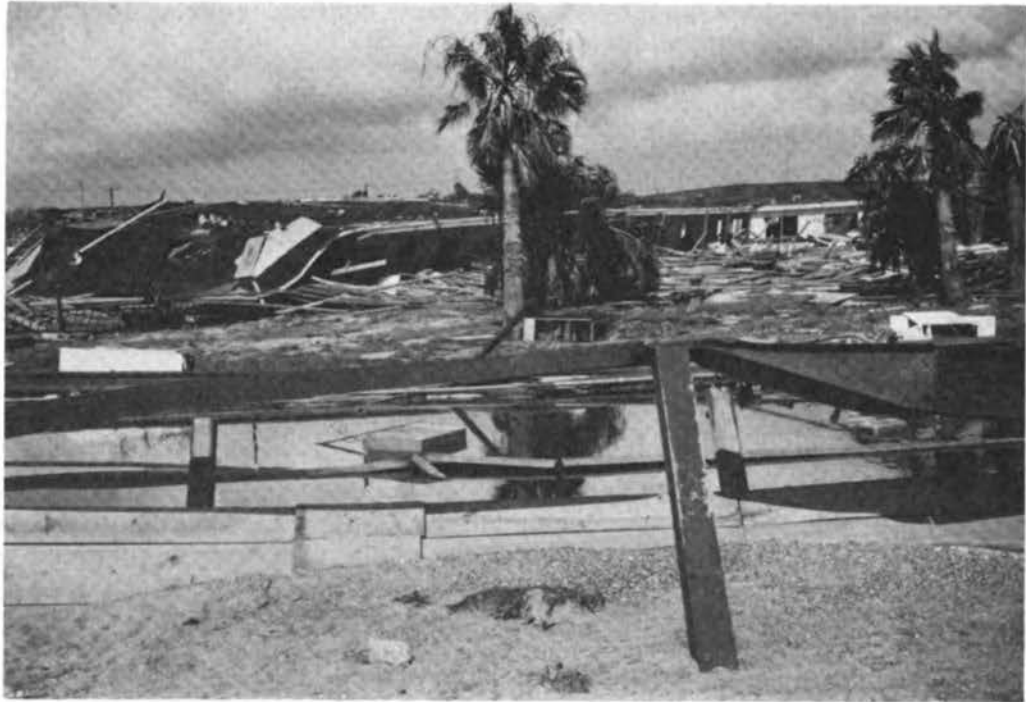
FIGURE 4.57 An elevated motel transported off its foundation by the storm surge.
