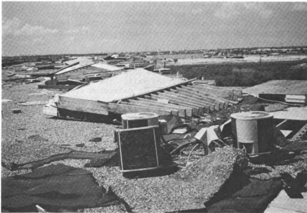
FIGURE 4.31 General view of the roof of the Victoria Hotel, showing damaged overhangs that landed on the roof.
