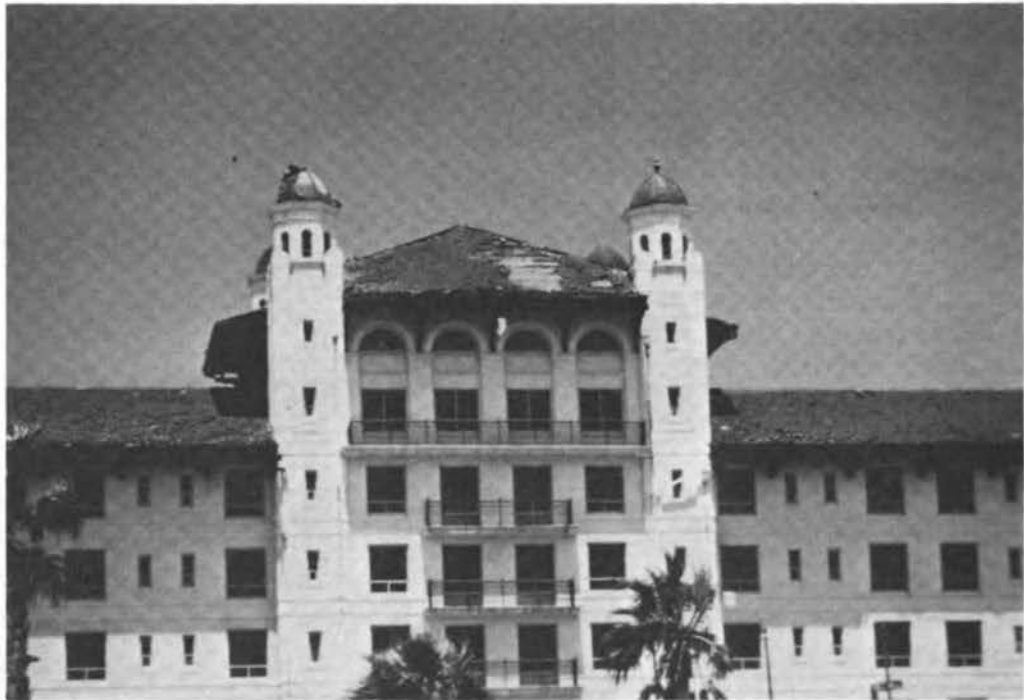
FIGURE 4.22 Damage to tiled roof of the Hotel Galvez.
