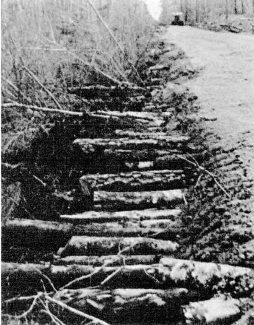
Figure 5 Corduroy road for crossing swampy areas.
