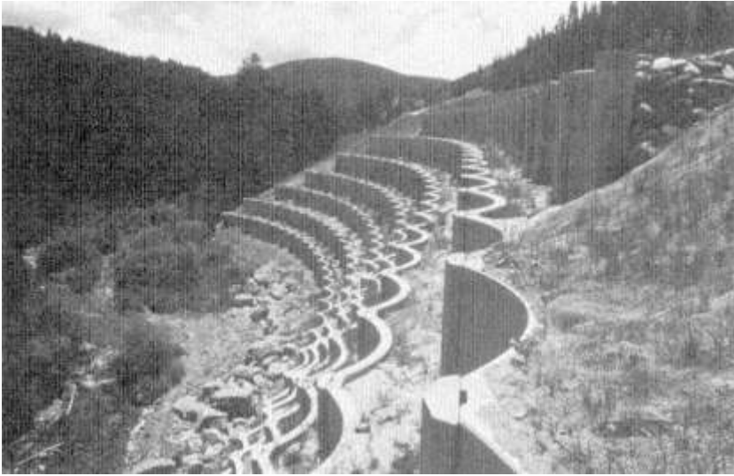
Figure 10 Special facing panels for reinforced earth wall along Interstate Highway 70 through Vail Pass, Colorado.
