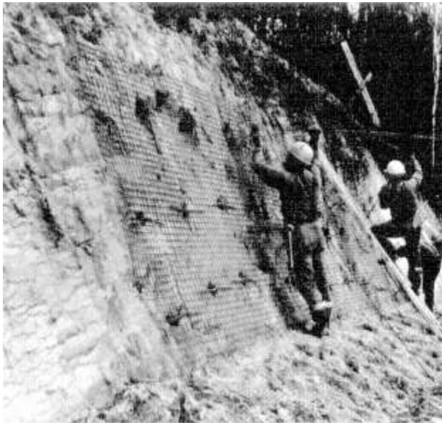
Figure 17 Soil nailing for improving cut slope stability.
