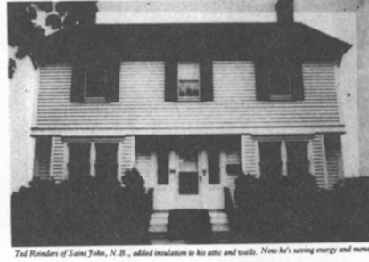
Ted Reinders of Saint John, N.B., added insulation to his attic and walls. Now he's saving energy and money.
