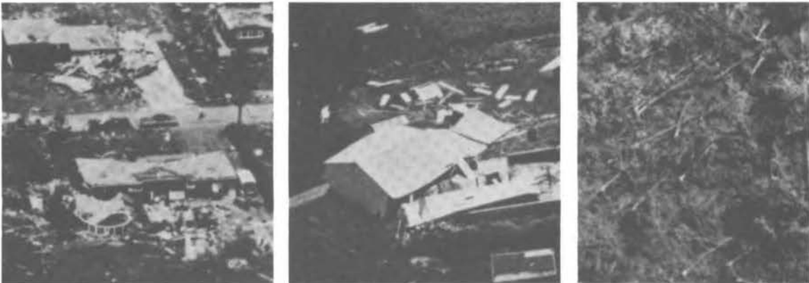
FIGURE 9B Moderate damage (F1) on the Fujita scale (winds 73 to 112 mph). Surfaces of roofs peeled off; windows broken; mobile homes pushed off foundations or overturned; outbuildings demolished; some trees uprooted or snapped; moving automobiles pushed off roads.
