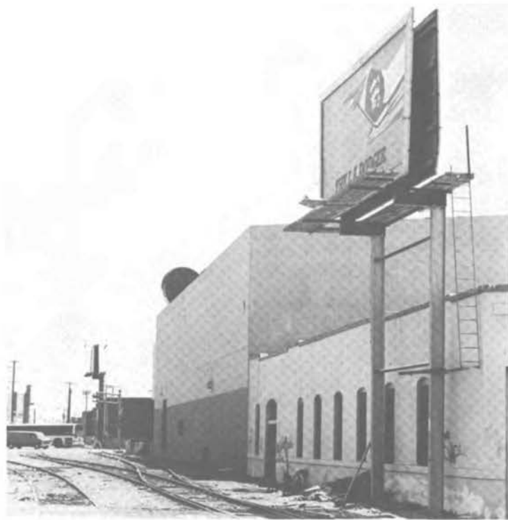
FIGURE 14B Repaired sign.
