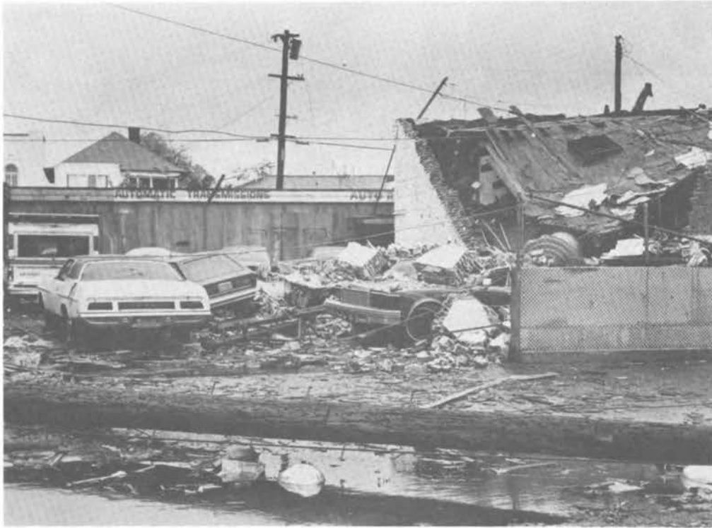
FIGURE 19 Failed masonry bearing wall.
