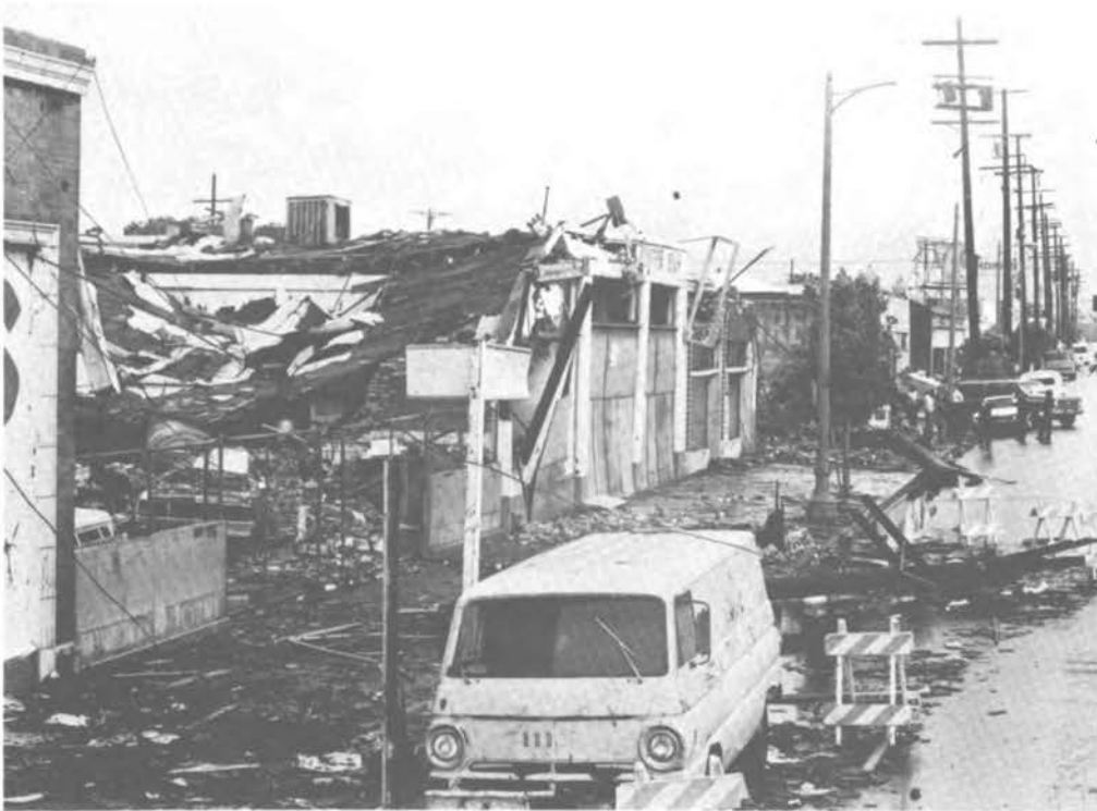
FIGURE 20 Failed masonry bearing wall.
