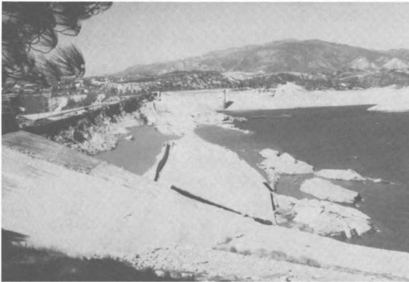
FIGURE 2-4 Failure of the Lower Van Norman San Fernando Dam during the San Fernando earthquake of 1971. Part of the upstream face of this 140-ft-high dam lost strength and slipped beneath the water. Eighty thousand people living below the dam in Los Angeles were evacuated from their homes for several days until the water level behind the dam was drawn down. Photograph: Courtesy of R. V. Whitman.
