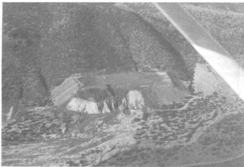
FIGURE 2-7b Liquefaction failure of a tailings dam in Cerro Negro, Chile, from the March 3, 1985, earthquake. Photograph: Courtesy of G. Castro.
