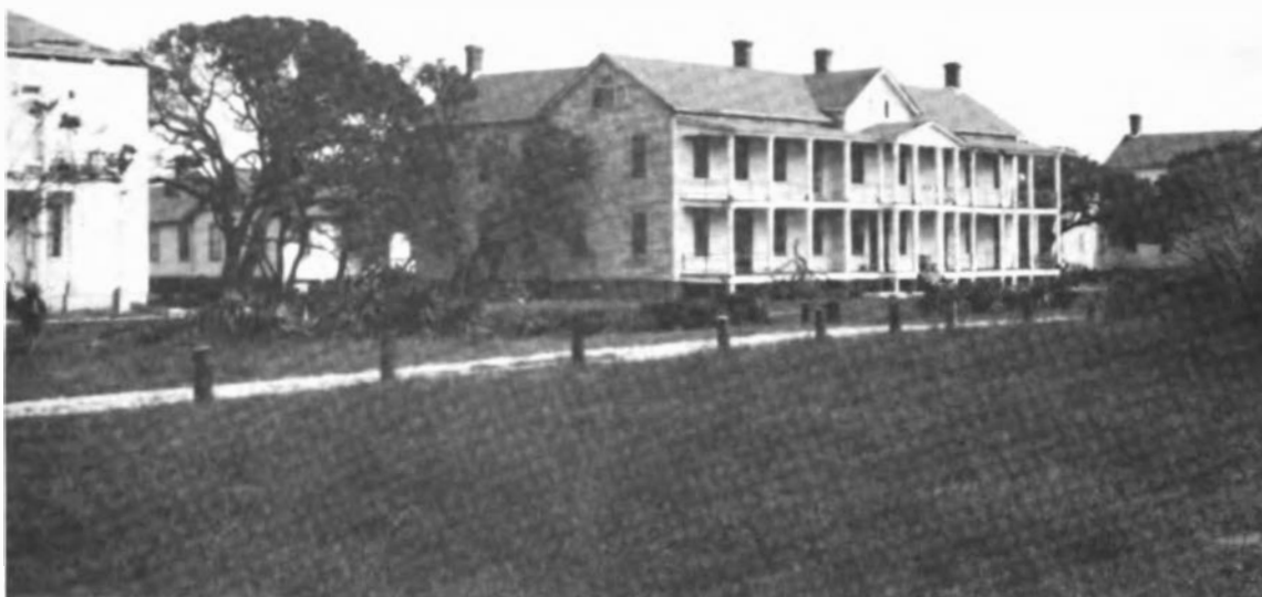
FIGURE 3.16 Undamaged military building, Fort Caswell.
