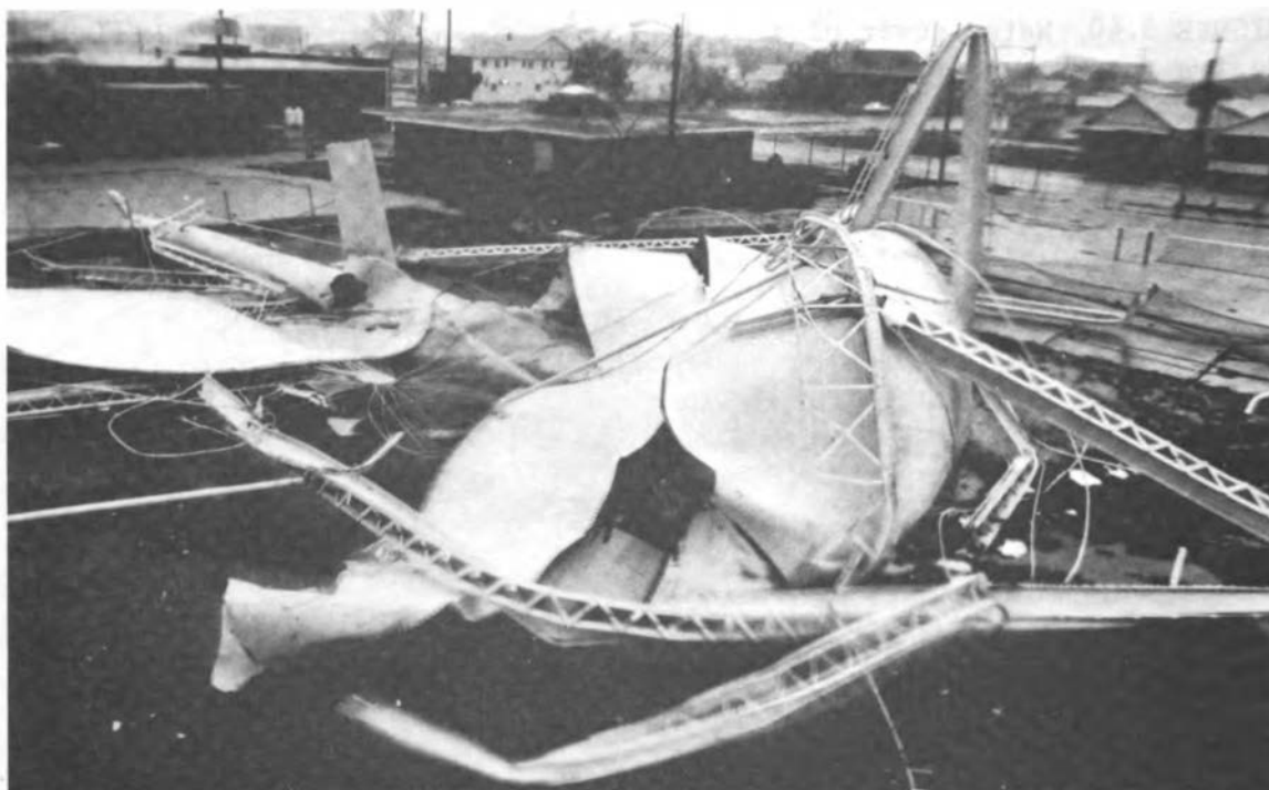
FIGURE 3.41 The tangled remains of Carolina Beach's 50 year-old 100,000-gallon water tower, which fell Wednesday, September 12, 1984. Photograph courtesy of Wilmington Morning Star , Friday, September 14, 1984; staff photograph by Jack Upton.
