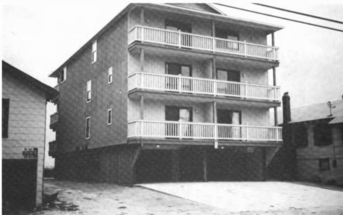
FIGURE 3.29 Undamaged condominium, Carolina Beach.
