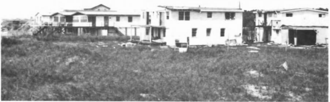
FIGURE 3.7 Apartment damage, Long Beach.
