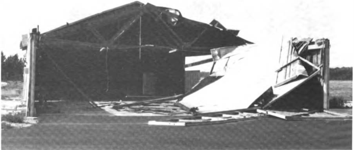
FIGURE 3.39 Brunswick County Airport hangar.
