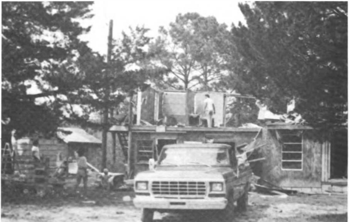
FIGURE 3.18 Severe building damage, Grouse Landing.
