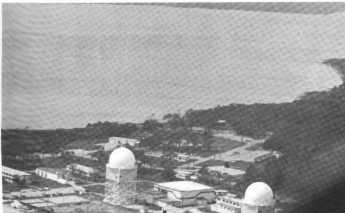
FIGURE 3.21 Undamaged radomes, Fort Fisher.
