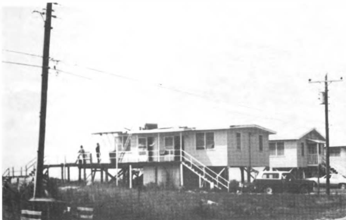
FIGURE 3.9 Typical weak porch construction, Long Beach.
