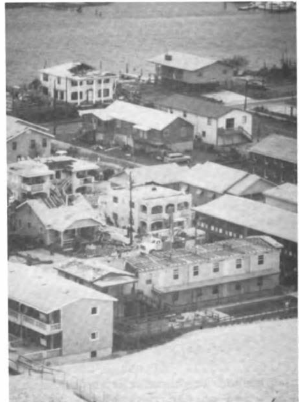
FIGURE 3.26 Motel roof failure and debris damage, Carolina Beach.
