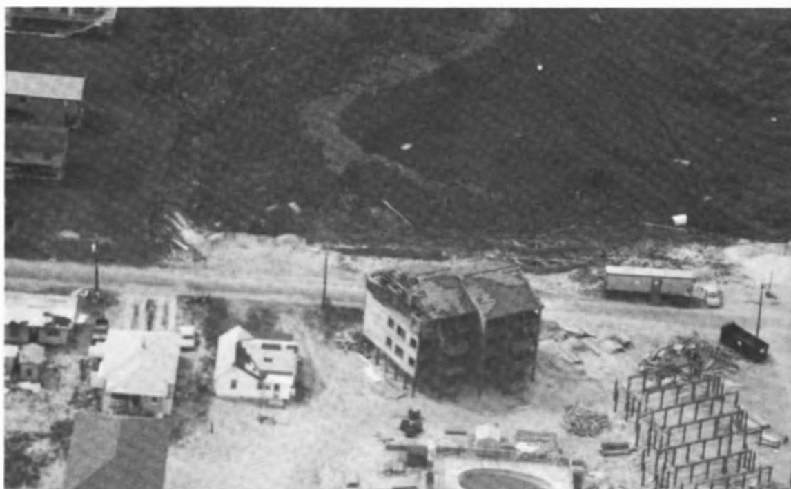
FIGURE 3.30 Gable-end failure in a condominium building, Carolina Beach.
