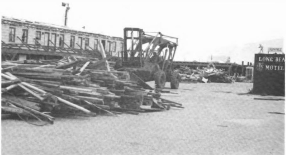
FIGURE 3.8 Porch failure at the Long Beach Motel.
