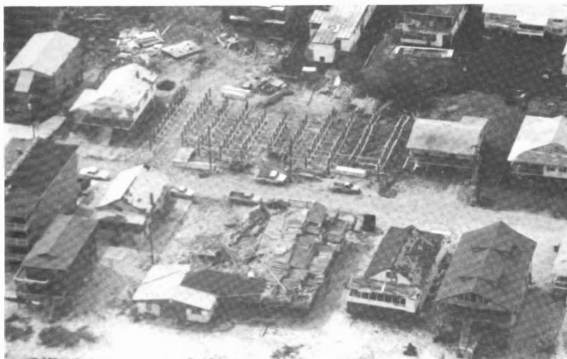
FIGURE 3.28 Collapse of condominium building, Carolina Beach.
