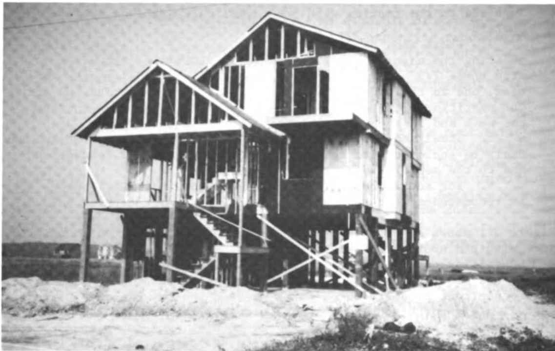
FIGURE 3.1 Typical coastal construction, North Carolina.
