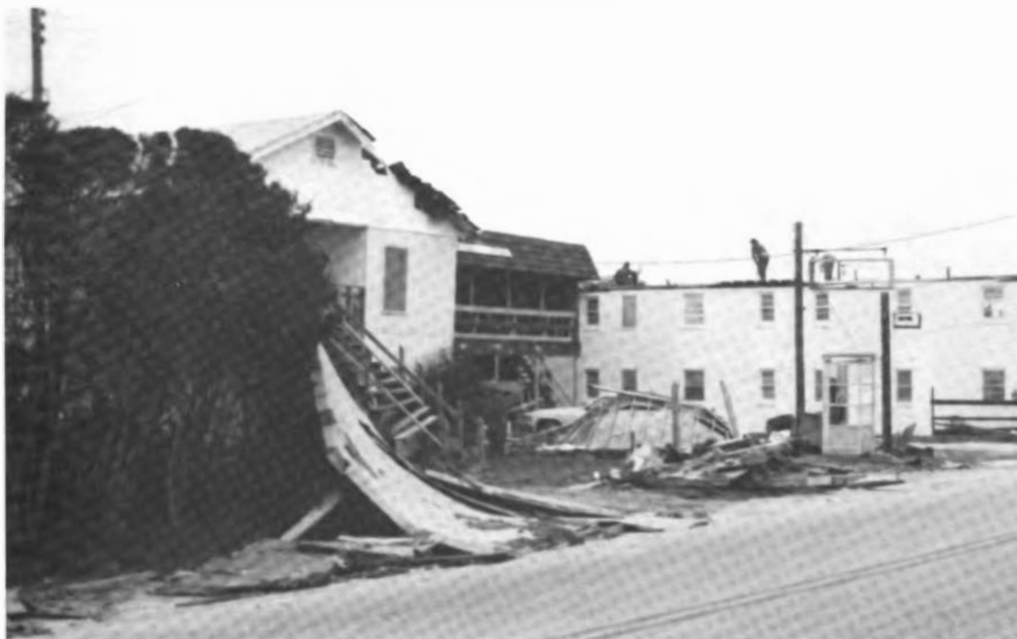
FIGURE 3.22 Motel damage, Wilmington Beach.
