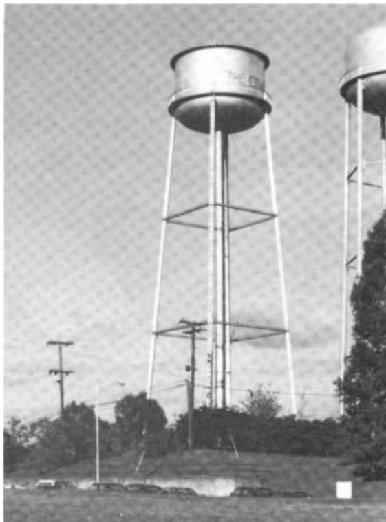
FIGURE 3.40 Water tower of similar design to the one that collapsed.
