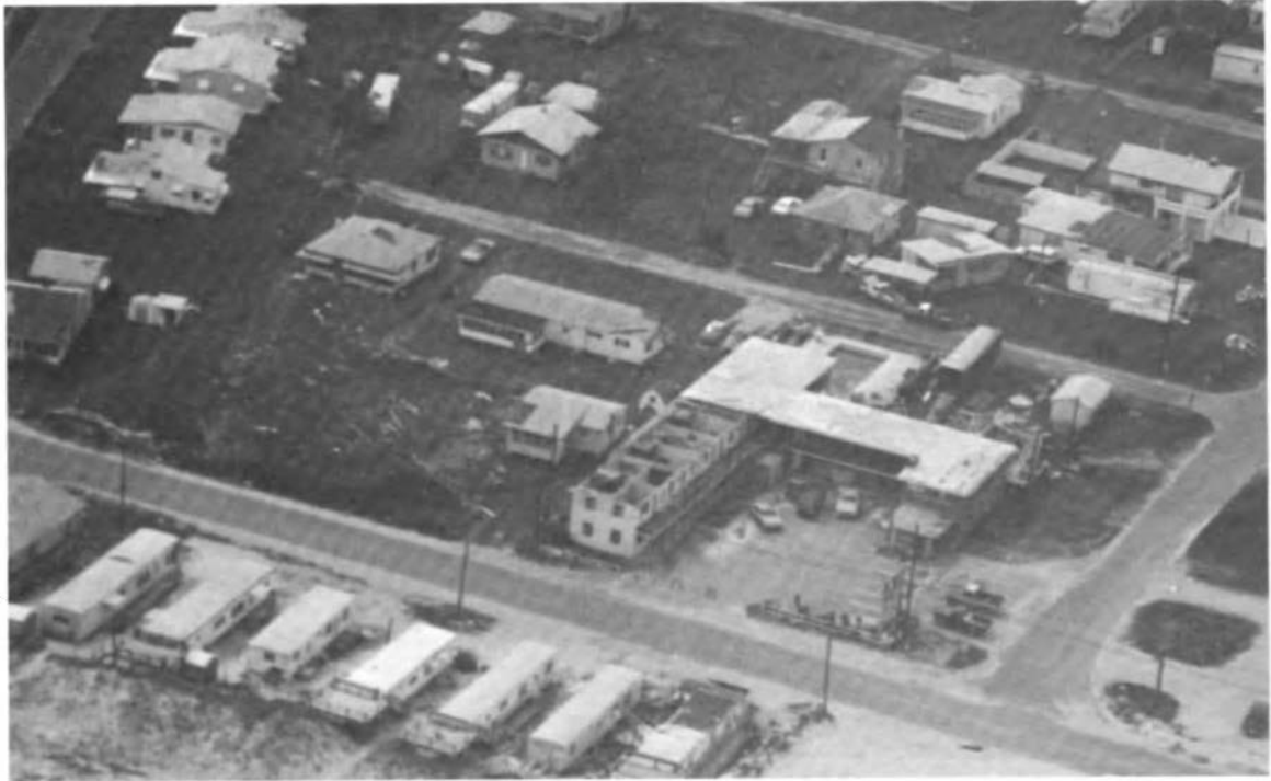
FIGURE 3.25 Roof damage to a masonry motel, Wilmington Beach.
