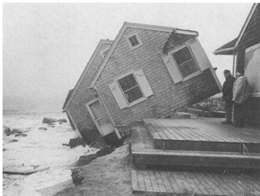
Figure 13.4 Cape Cod house tumbles into the sea in 1988 after a break in offshore barrier spit increased shoreline erosion at Chatham, Massachusetts. (Courtesy of Cape Cod Times .)
