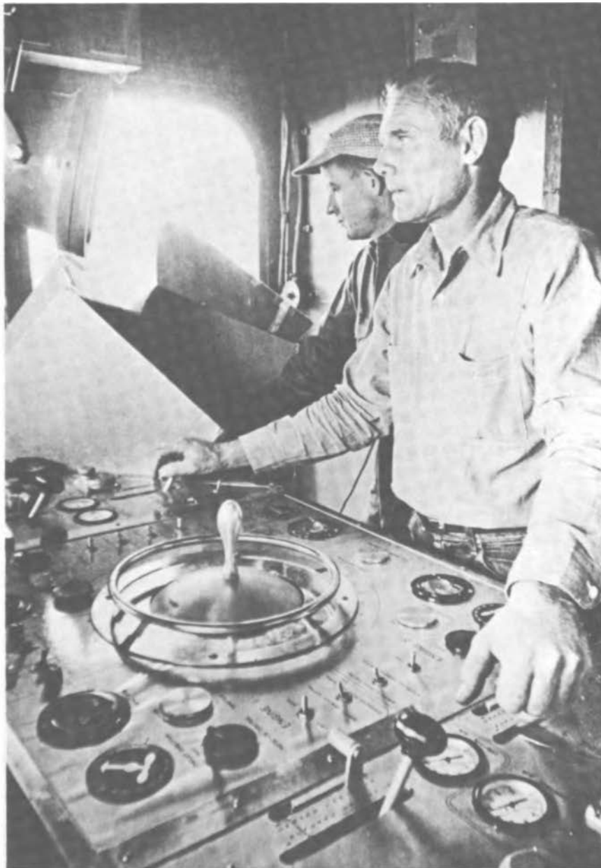
FIGURE 3 The steering console on CUSS 1 . The joystick control was used as part of the dynamic positioning system. Credit Fritz Goro, LIFE magazine, April 1961.
