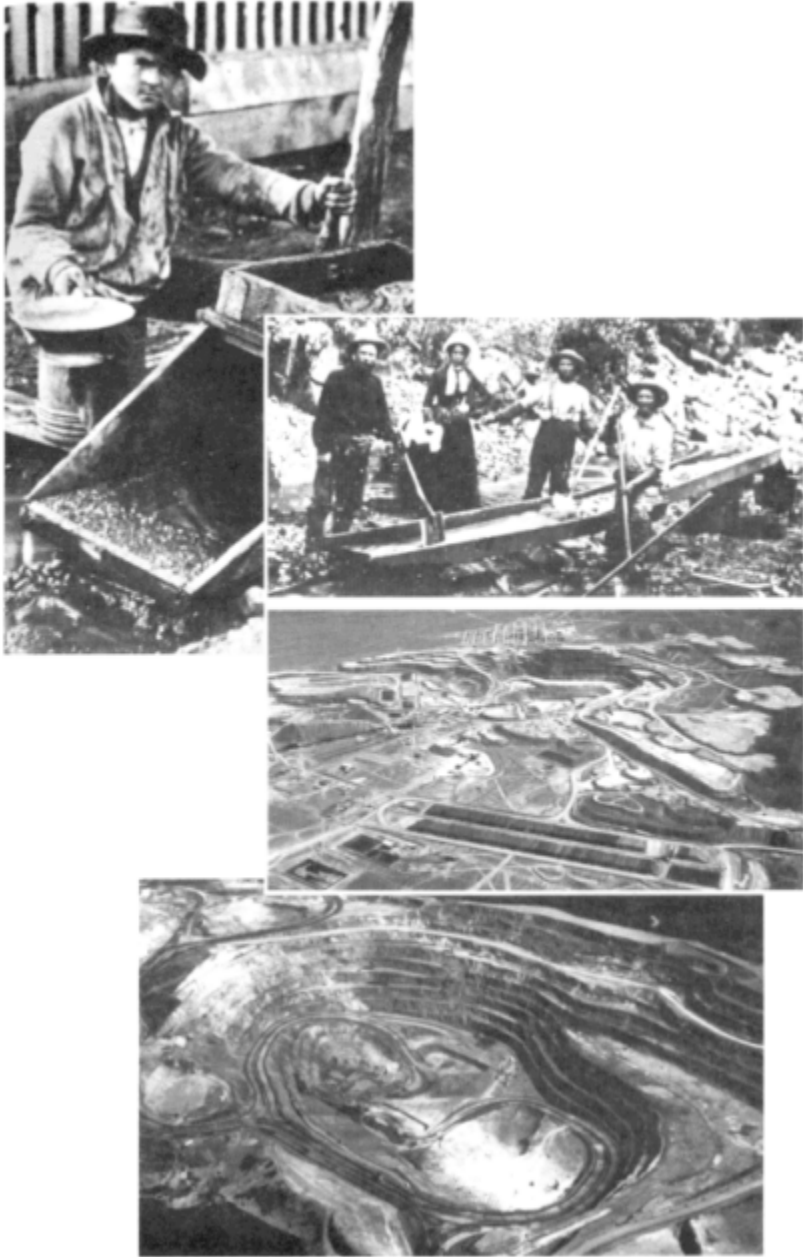
Frontispiece: California hand jig, c. 1860; California placer gold gravity rocker, c. 1860 (Courtesy N. Arbiter); Gold operations: Round Mountain, NV and McLaughlin, Lower Lake, CA (Courtesy Homestake Mining Co., photographer Mickey Brim)
