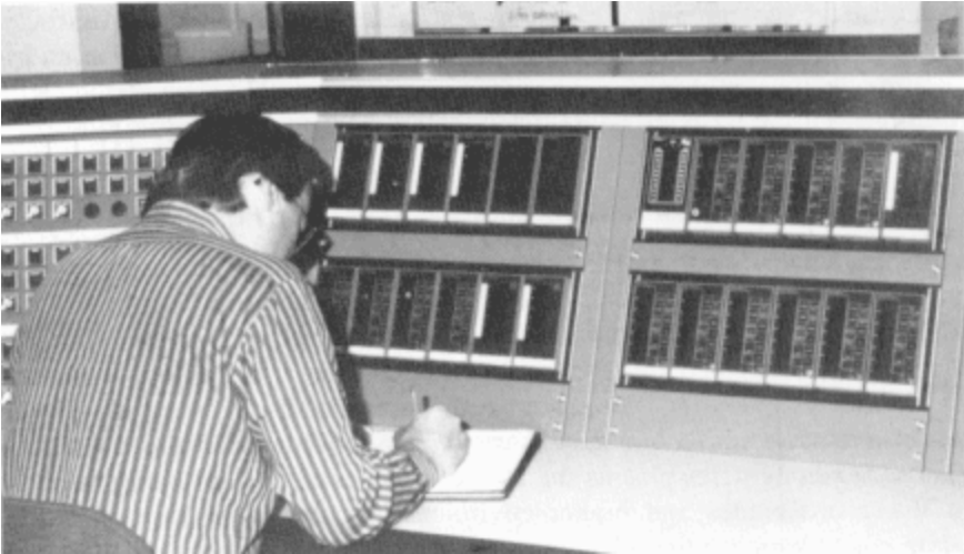
At San Manuel Copper Mine in Arizona, underground trains are controlled by a radio dispatcher from the surface. (Courtesy Magma Copper Company.)
