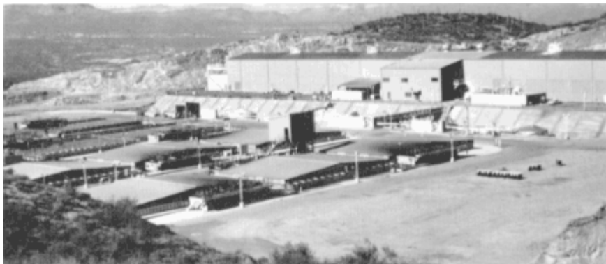
Solvent Extraction/Electrowinning Plant at San Manuel Mine, Arizona. (Courtesy Magma Copper Company.)
