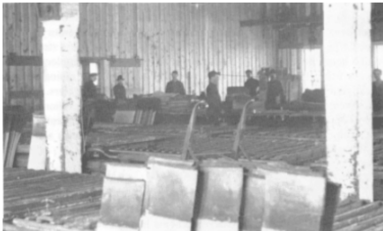
Anaconda refinery cathode room, 1902. (Courtesy N. Arbiter.)
