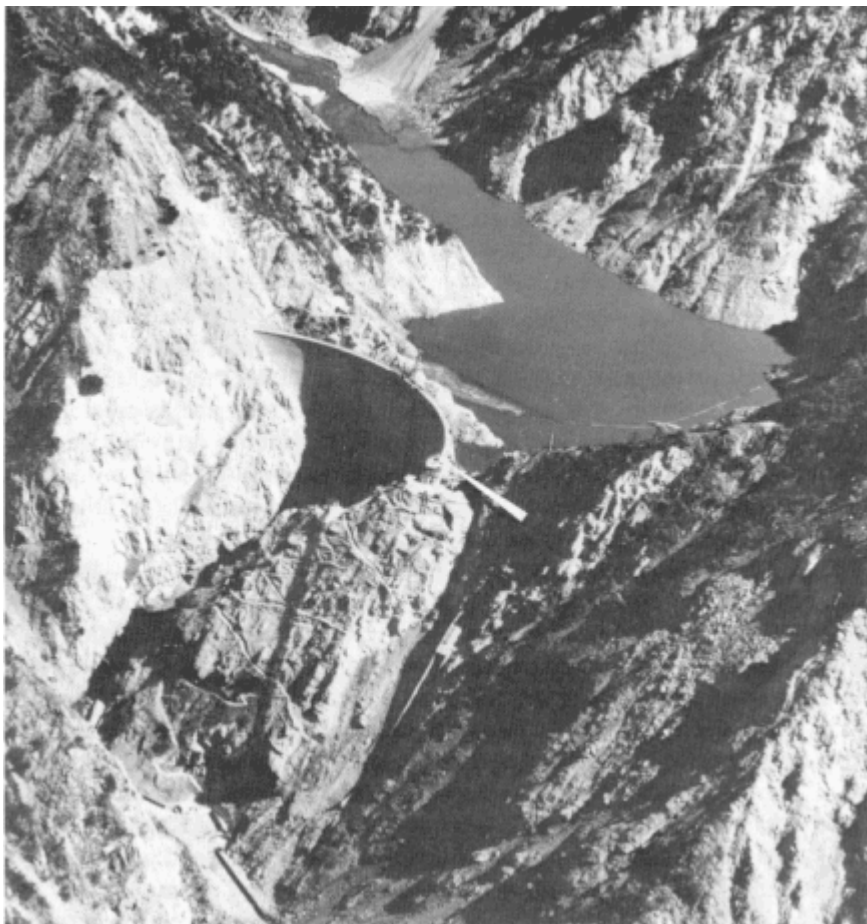
Figure 2-4 Pacoima Dam, California, was subjected to the 1971 San Fernando earthquake; the seismic motions were recorded by a seismograph on the narrow rock ridge above the left abutment, at the point indicated (2-28). (Courtesy of George W. Housner)
