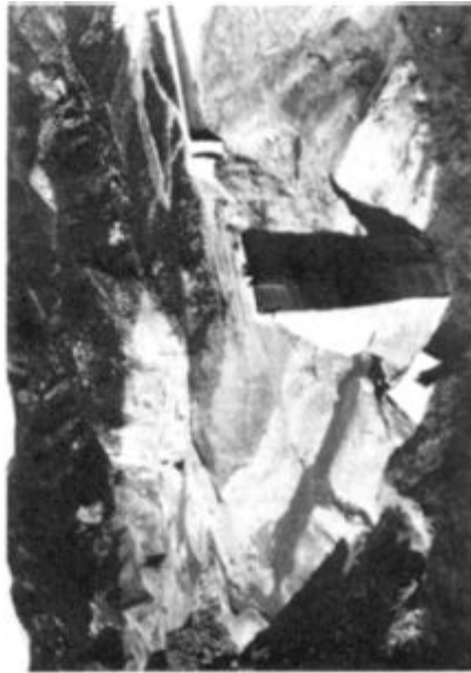
Figure 1-1 St. Francis Dam. The 1928 failure of this dam, caused by shear failure in the foundation rock, led to promulgation of dam safety legislation in California. (a) Before failure, the dam was 205 ft high and 700 ft long and retained 35,000 acre-feet of water. (b) The foundation failure caused dam rupture, and the reservoir release completely destroyed the dam.
