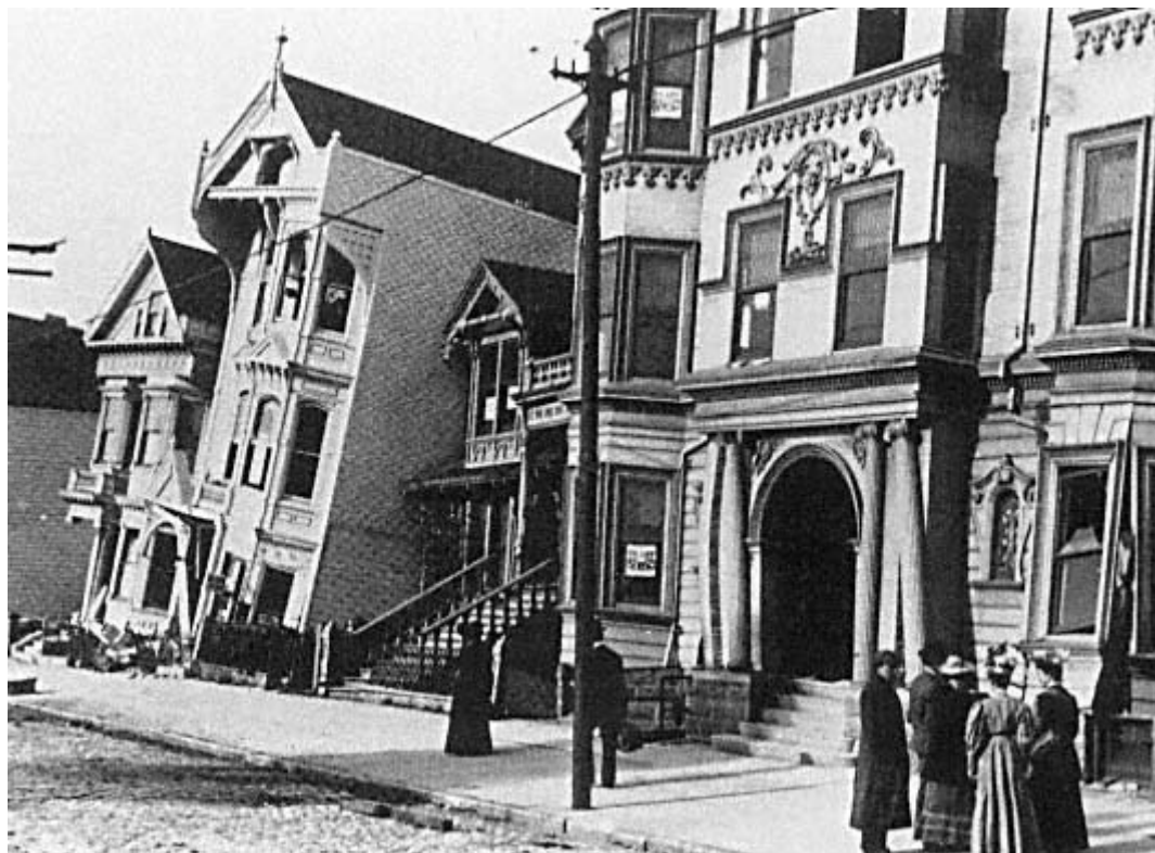
Disasters have been a part of life throughout history. San Francisco residents, circa 1906, examine the angle of list on a row of town houses damaged in the famous magnitude 8.3 quake.
