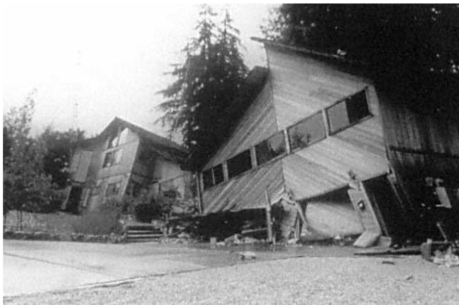
Building code and land-use management can help reduce the number of structures damaged during earthquakes and their resulting landslides, liquefaction, and upheaval.
