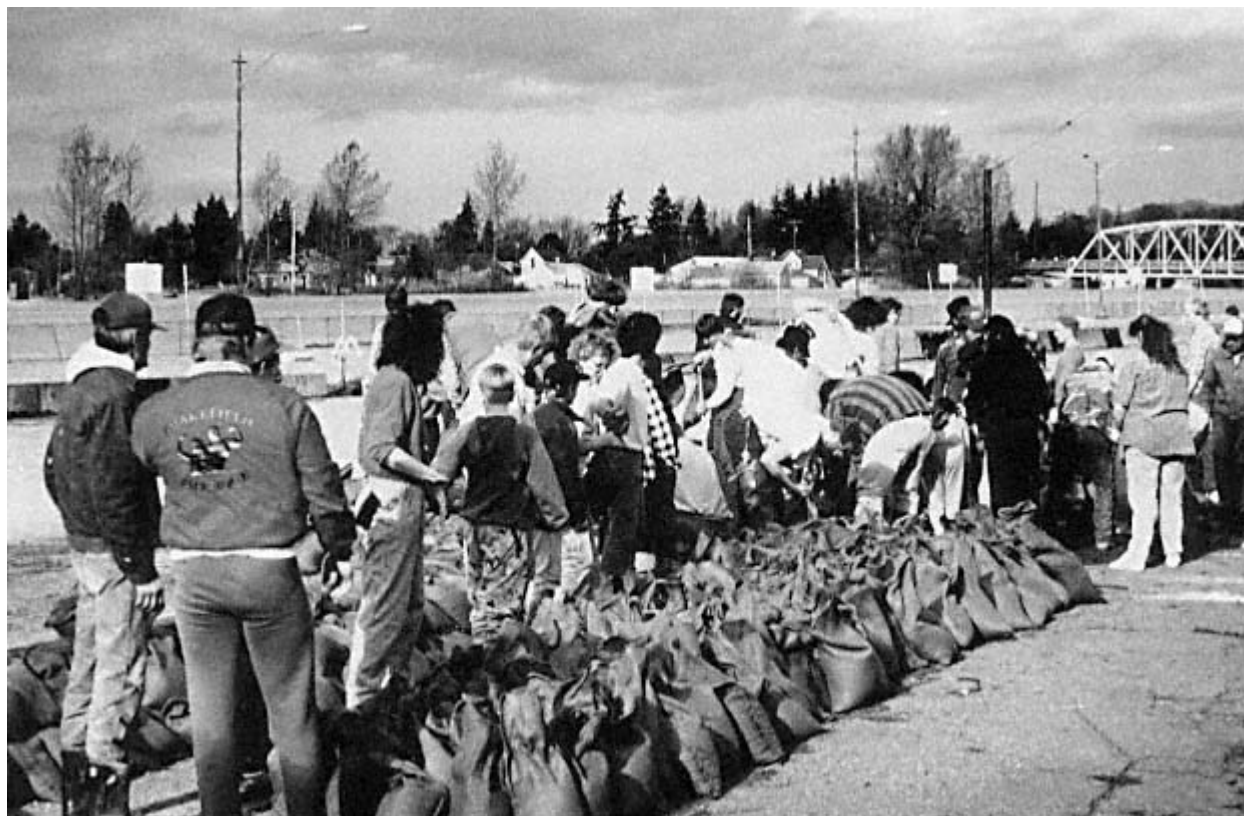
The line of action is the local community, and often mitigation and preparation are most useful in their most basic form, such as a brigade of volunteers filling and stacking bags to hold back rising river waters.
