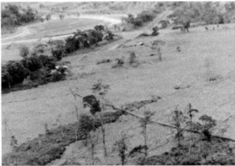
FIGURE 6.9 Broad fan of a very large debris flow with the Trans-Ecuadorian pipeline deformed in the direction of debris movement.
