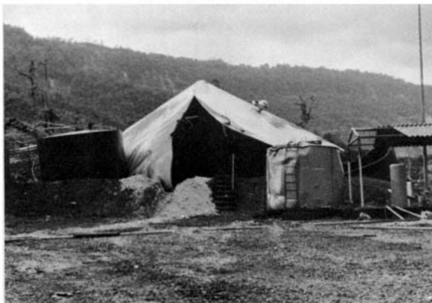
FIGURE 6.14 Oil tank destroyed by landslide debris at the Salado pump station.
