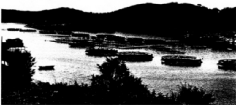
Production facility (the Fishery, Sacramento, California) for culturing striped bass, white sturgeon, and catfish. Hatchery operations are sheltered by the open shed (right center). Sturgeon and some other fish are reared in tanks (foreground), and striped bass and catfish are reared in ponds (barely visible beyond the buildings). Water discharge from the tanks flows to the ponds.
