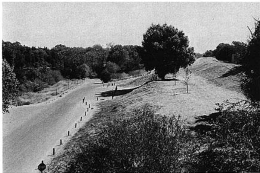
PHOTO 2.3 The potential for channel instability is increased in areas with hydraulic mining deposits, such as this site along the left bank of the American River near Watt Avenue. The terrace surface extends upstream and downstream, as well as beneath the levee. (Allan James, University of South Carolina.)
