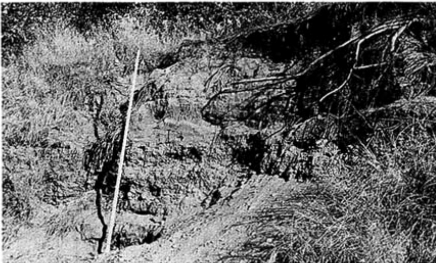
PHOTO 2.2 Hydraulic mining sediment deposits often consist of erodible, unconsolidated sand and gravel. At river mile 21, about six feet of historical sediment cap about 3 feet of older sediment. (Allan James, University of South Carolina.)
