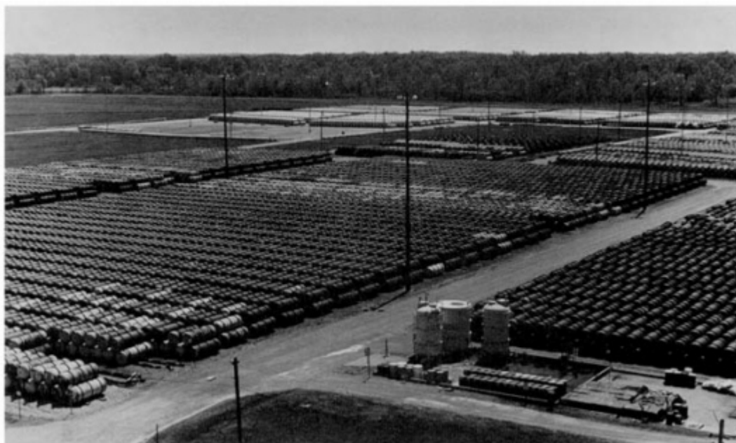
FIGURE 7-1 \text{DUF}_6 cylinder storage yards at Paducah. (Yards encompass about 40 acres and contain about 20,000 cylinders or 40 percent of total DOE inventory.)
