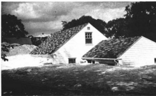
FIGURE 1-1 Alluvial fan flooding: High-velocity flows battered homes in Ocotillo Wells, California, during the September 1976 flood caused by Tropical Storm Kathleen (top). Fast-moving floodwaters caused scour, erosion, and structural damage to numerous Rancho Mirage, California, homes in September 1976 and July 1979 (middle). Large volumes of sediment can be deposited by floodwater during the course of an alluvial fan flood event (bottom). SOURCE: FEMA (1989).
