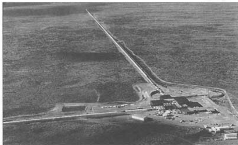
FIGURE 7.8 The LIGO site at Hanford, Washington, showing the 4-km arms stretching from the main building. The interferometer mirrors, or test masses, are isolated from ground vibrations to allow extremely sensitive measurements for the detection of gravitational waves. (Courtesy of LIGO.)
