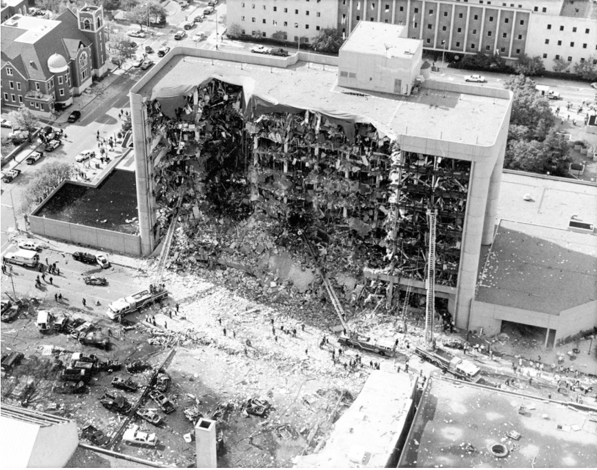
Postblast remains of the Alfred P. Murrah Federal Building, Oklahoma City, April 1995. SOURCE: AP/Wide World Photos.
