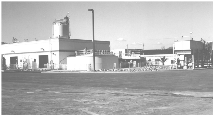
The Aqua II pilot facility, used to demonstrate the feasibility of wastewater reclamation for San Diego, California. Photo courtesy of the City of San Diego.
