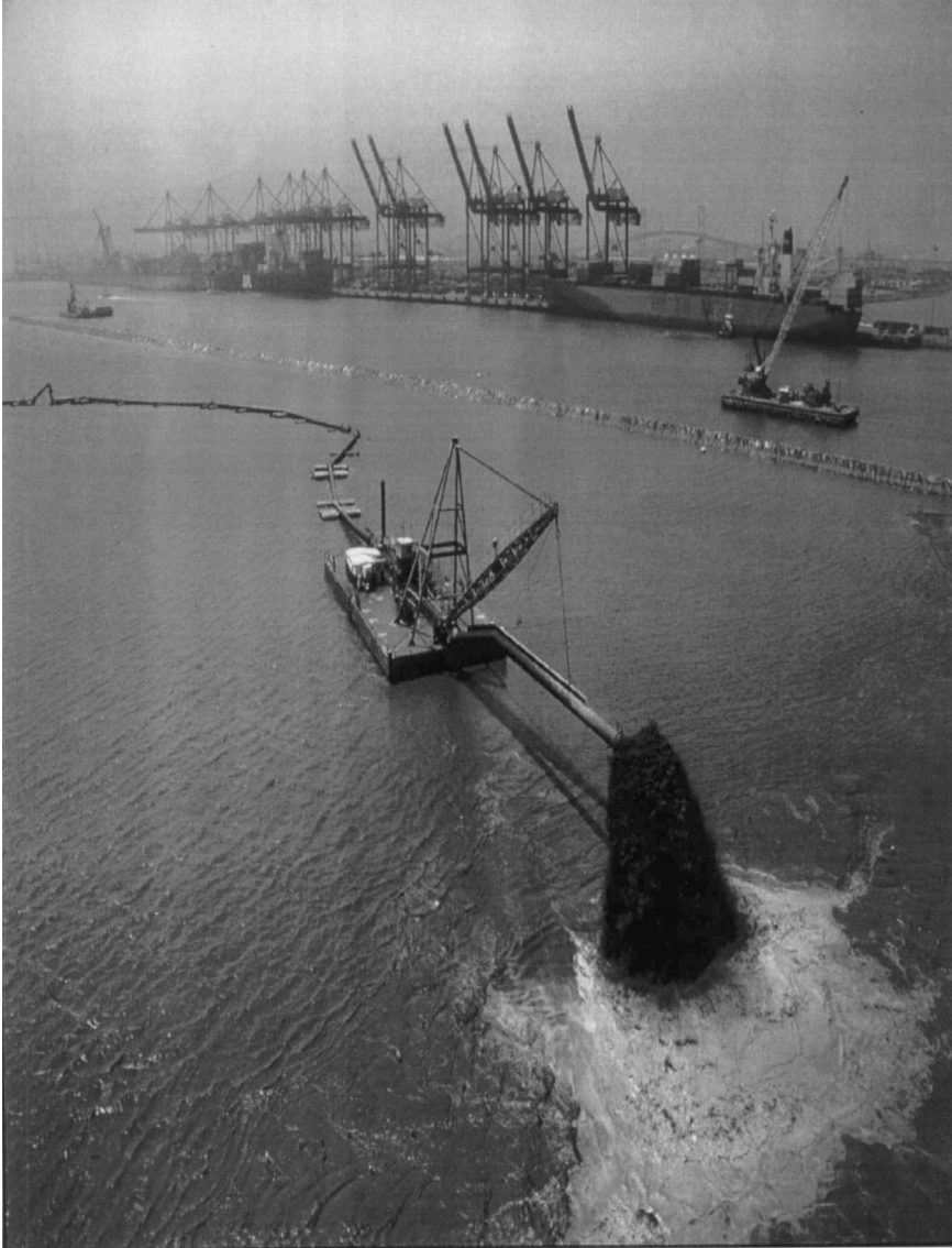
Dredging operations in the Port of Los Angeles. Courtesy of the Port of Los Angeles.
