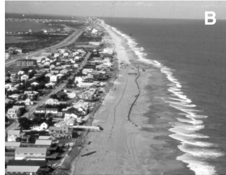
B. Fenwick Island receiving beach nourishment sand pumped from approximately three miles offshore.
