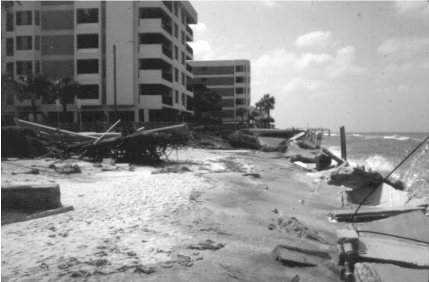
Seawalls destroyed by hurricane Elena in Pinellas County, Florida, September 1985. Courtesy of Robert G. Dean, University of Florida, Gainesville.
