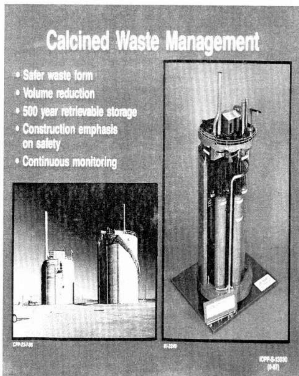
Figure 1.1(b) The photograph on the left shows Bin Set 5 and Bin Set 6 of the INTEC Calcine Solid Storage Facilities. The scale-model of Bin Set 6 on the right depicts construction details and the arrangement of bins inside each of the seven bin sets. SOURCE: INEEL photograph #ICPP-S-13030.
