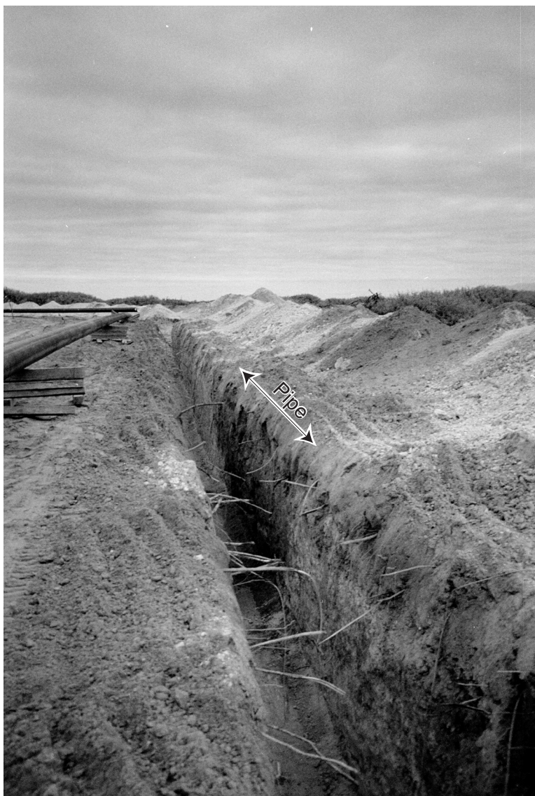
FIGURE 5-14 A pipe through an indurated calcic horizon on the La Mesa surface in New Mexico (Rodríguez-Marín and Hendrickx, personal communication, 1999).
