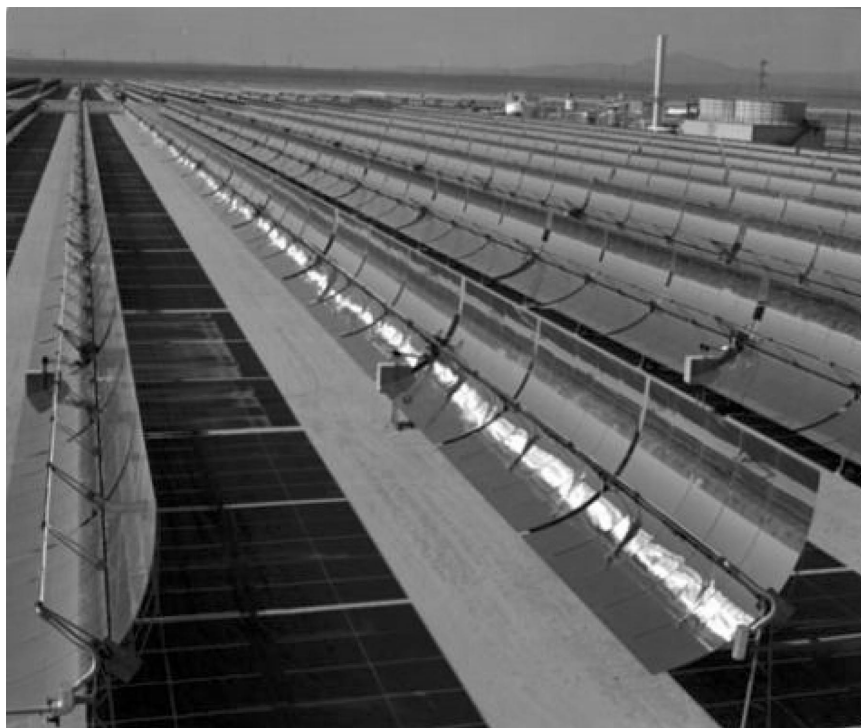
FIGURE 7.4 Nine trough power plants in California's Mojave Desert provide the world's largest generating capacity of solar electricity, with a combined output of 354 MW. These systems provide large-scale power generation from the sun and, because of their proven performance, are gaining acceptance in the energy marketplace.
