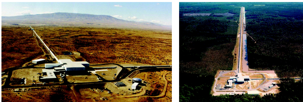
FIGURE 6.4.1 Aerial photographs of the interferometers used in the Laser Interferometer Gravitational Wave Observatory (LIGO). The long tunnels house the evacuated laser chambers, in which laser beams travel a 4-km path length. At the vertex of the L, and at the end of each of its arms, are test masses that hang from wires and that are outfitted with mirrors. Ultrastable laser beams traversing the vacuum pipes are used to detect the ultrasmall change in the separation of a pair of test masses caused by the passage of a gravitational wave. Images courtesy of the LIGO Laboratory.
