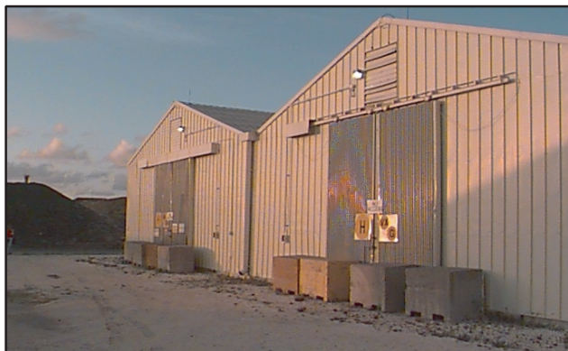
(a) West Side of Building 850
