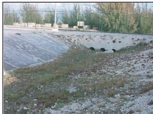
(b) Drainage Culvert Between Buildings 851 & 852
