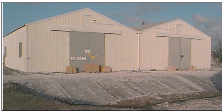
(a) East Entrance to Building 851 and Drainage Culvert
