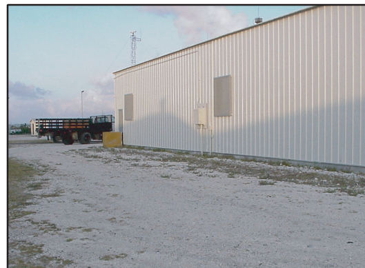
(b) South Side of Building 850
