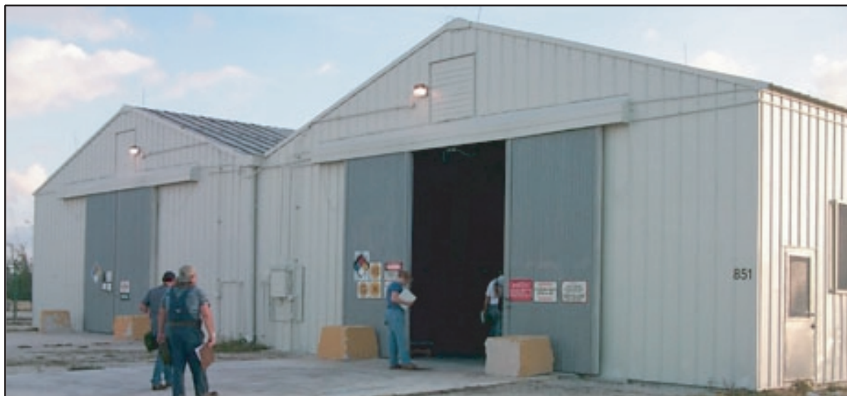
(a) West Entrance to Building 851
