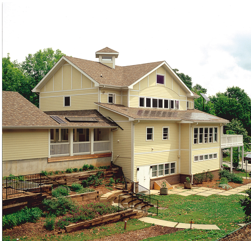
FIGURE 5-3 The Southface building was built to promote health, conserve energy, improve water efficiency and demonstrate the use of low-impact environmental materials. SOURCE: Neal Dent. Reprinted with permission from Southface Energy Institute.
