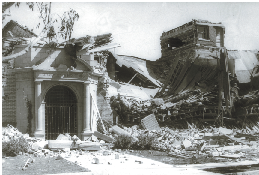
FIGURE 2.16 Jefferson Junior High School destroyed in the Long Beach earthquake. The Field Act, passed one month after the earthquake, prohibited this type of masonry construction for schools in California. SOURCE: Steinbrugge Collection, Earthquake Engineering Research Center, University of California, Berkeley. Photograph by Harold M. Engle.
