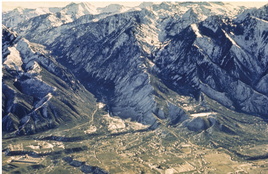
FIGURE 2.4 Aerial view, Salt Lake City, showing the scarps of active normal faults of the Wasatch Front, first recognized by G.K. Gilbert. SOURCE: Utah Geological Survey.
