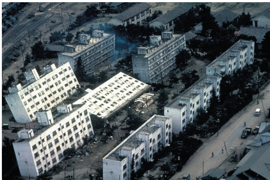
FIGURE 3.4 Tilting of apartment buildings at Kawagishi-Cho, Niigata, Japan, produced by liquefaction of loose, water-saturated sediments caused a loss of load-bearing capacity during the 1964 Niigata earthquake (M 7.5). The losses from this earthquake exceeded $1 billion in 1964 dollars. SOURCE: National Oceanic and Atmospheric Administration, National Geophysical Data Center.
