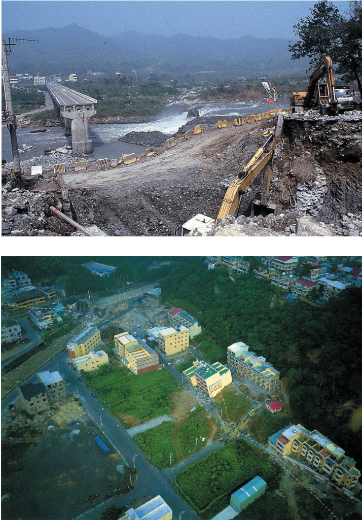
FIGURE 3.1 Damage due to fault rupture during the September 20, 1999, Chi-Chi, Taiwan, earthquake (magnitude [M] 7.6) was extensive along the Chelungpu fault. Structures that were built to withstand strong ground motion nevertheless did not survive severe dislocations along the fault. The left abutment of this bridge across the Ta-An River was constructed through the fault plane ( top ). The thrust fault slipped about 10 meters during the earthquake, severely deforming the pillar and, thus, destroying the bridge. After the earthquake, the abutment was reconstructed in the same location. Most reinforced multistory concrete structures survived the shaking, but those on the fault trace collapsed or suffered severe tilts and other distortions, which rendered them uninhabitable ( bottom ). SOURCE: Photographs courtesy of Kerry Sieh, Caltech.
