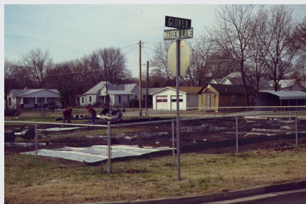
Plots at the Joplin Superfund Site being subjected to soil amendment in order to reduce metal bioavailability to residents.
