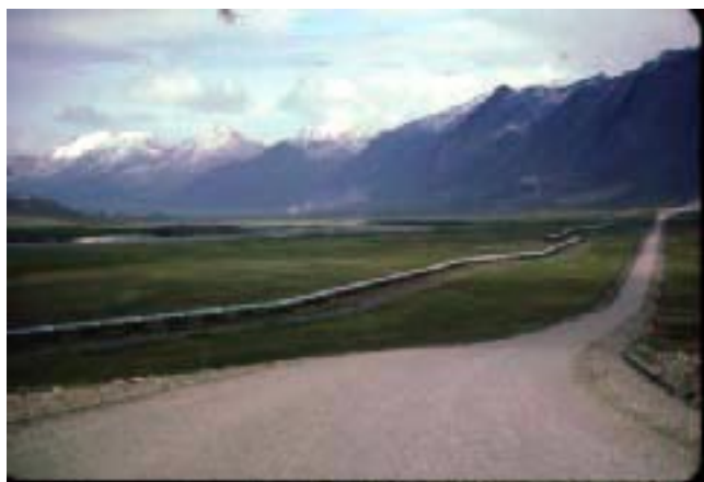
The Trans-Alaska Pipeline and Dalton Highway looking towards the Brooks Range. July 2001. Photograph by David Policansky.
