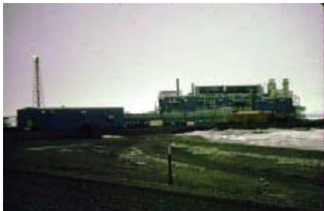
Oil-production facility, Endicott, July 2001. Photograph by David Policansky.
