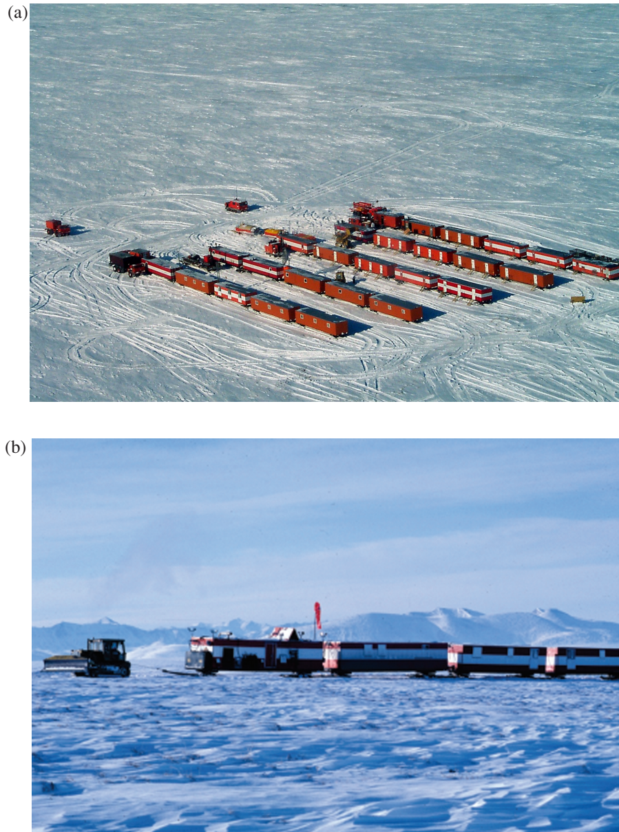
FIGURE 7-4 (a) Trailers on skids make up Camp 794 on the tundra of the National Petroleum Reserve-Alaska. Photograph by Erik Hill, courtesy of the Anchorage Daily News . Reprinted with permission. (b) Tractors towing camp trailers during a camp move in the Arctic National Wildlife Refuge, 1984. SOURCE: Jorgenson et al. 1996.
