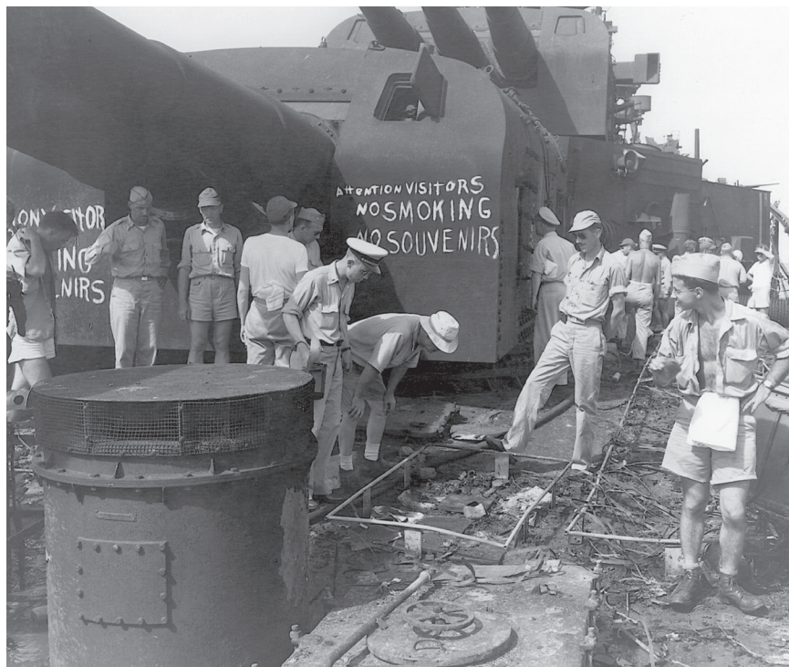
FIGURE V.B.1 Damaged quarterdeck on USS Pensacola .
