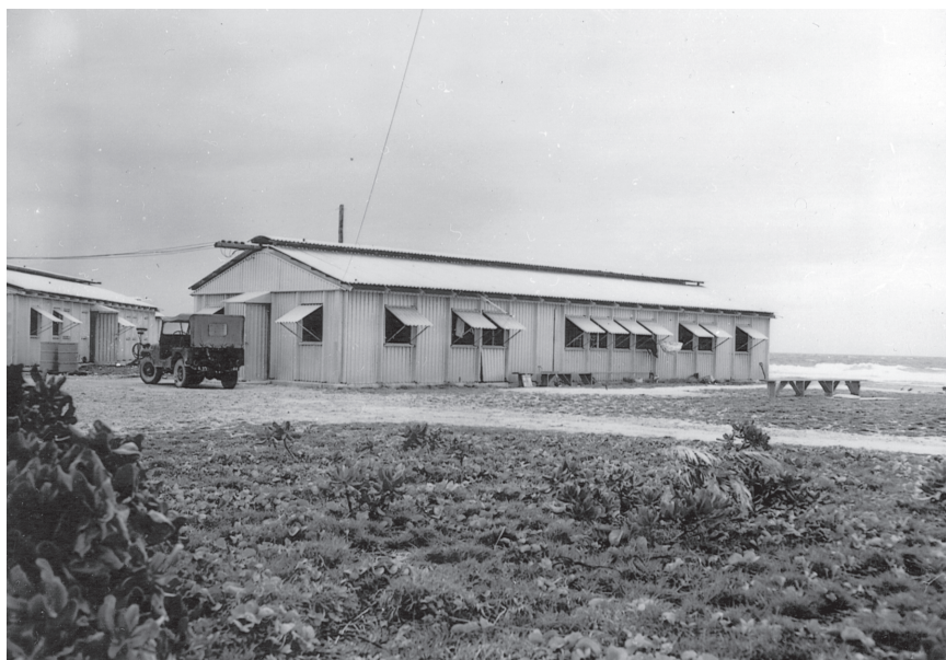
FIGURE V.A.1 Typical metal buildings used at Enewetak during Operation CASTLE.
