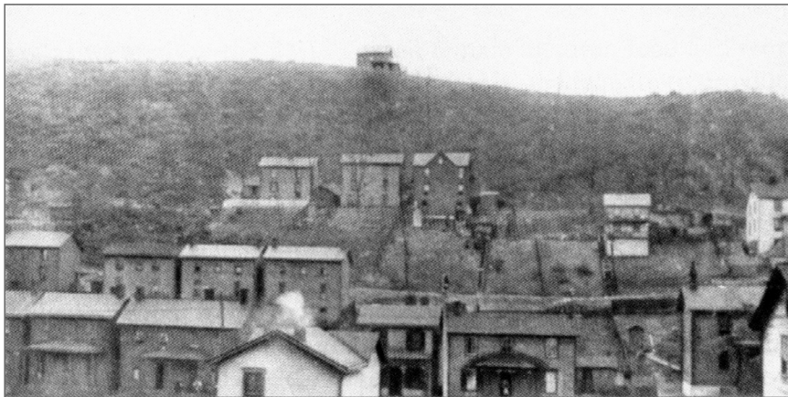
FIGURE 3–2 This picture circa 1910 on the outskirts of Pittsburgh illustrates the effect that air pollution had on the growth of vegetation. At this time, it was common to have trees denuded by the fumes. SOURCE: Byington, 1910.
